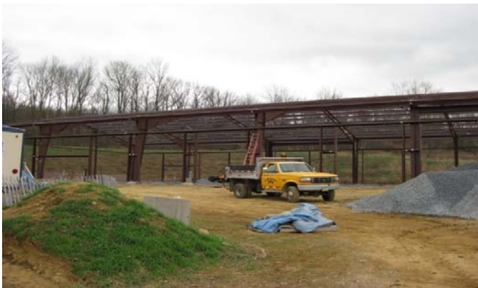
An OSC audit detailed the poor management practices that caused this Washington Borough garage project to increase nearly five-fold in cost while yielding minimal construction progress over a 10-year-period.
