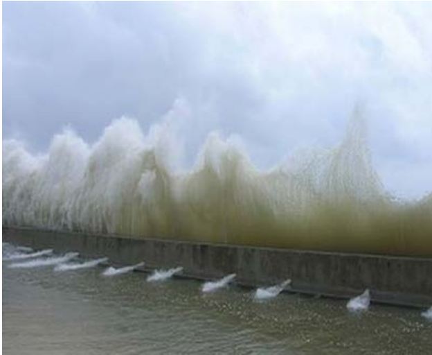
Figure 10: Wave overtopping action at waterfront structure (courtesy of FEMA)
