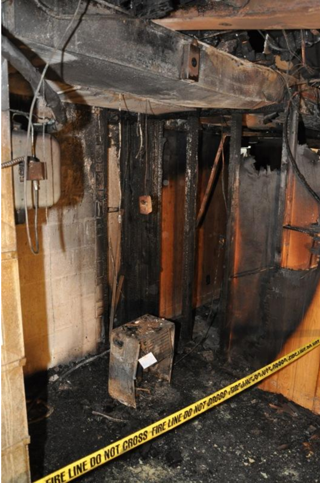
This fire at a home in Valparaiso, Ind. involved a recalled Goldstar dehumidifier and resulted in $192,000 in damage.
