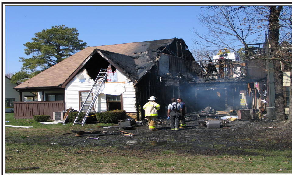
Photograph courtesy of NJDFS Office of Fire Department Preparedness
