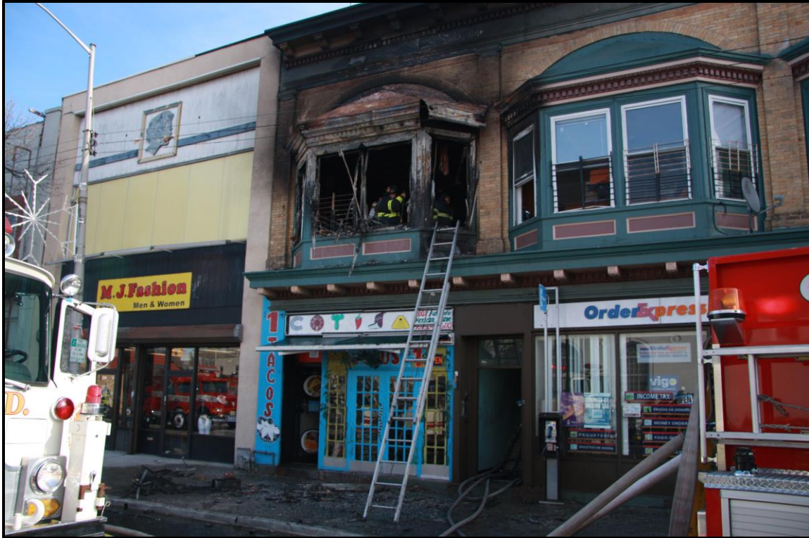
Figure 1 – Side A view of structure after fire was extinguished.
