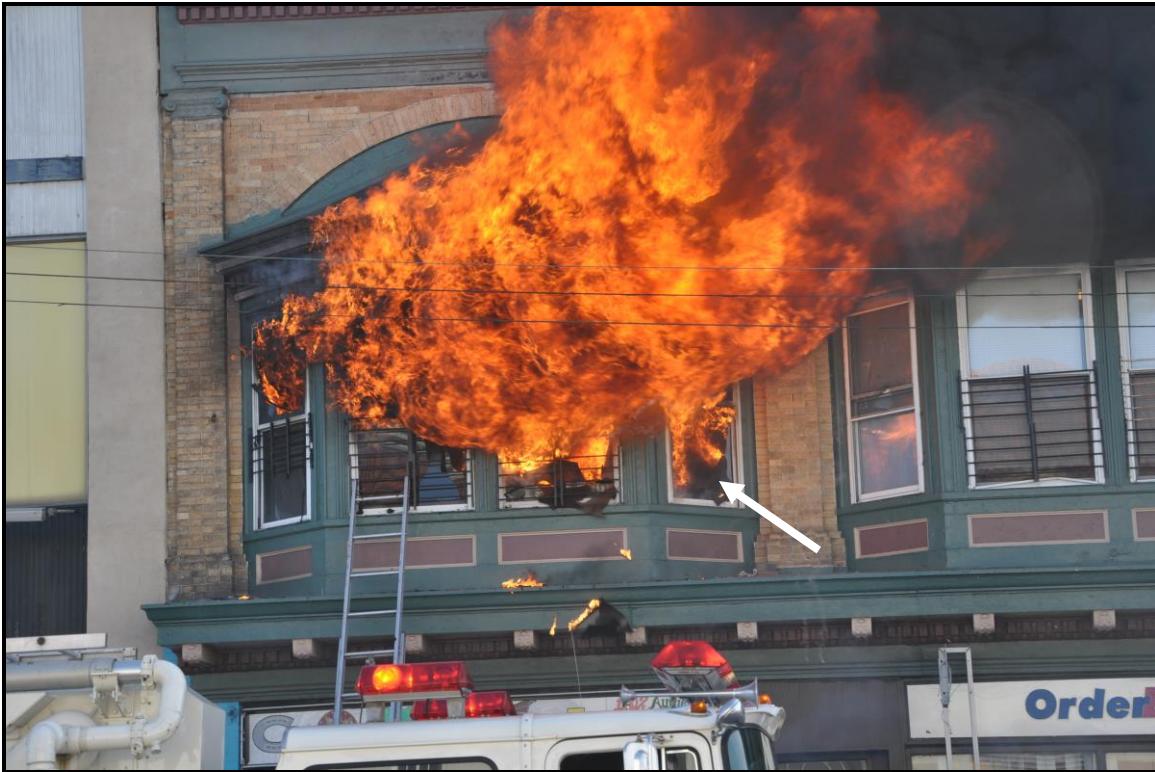
Figure 3 – Photo shows the flashover conditions after ventilation was completed. FF Fazio was still inside the flashover room at this time. He was able to escape by diving out the right side window of the room where flames were emanating (the only one without window guards; see arrow above).
