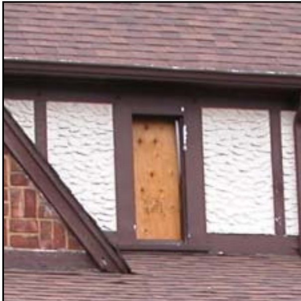
Figure 4 - An exterior view of the same second floor bathroom window where two children and their mother were removed from the home.
