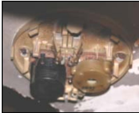
Figure 6 – This photograph shows the smoke detector that was located in the basement. It shows that the battery was missing at the time of the fire. This is evidenced by the uniform discoloration of the unit caused by the fire.
