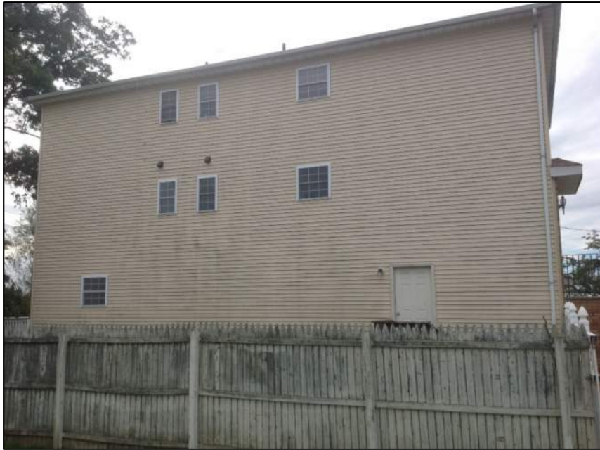
Photo 3: Left Side of House
