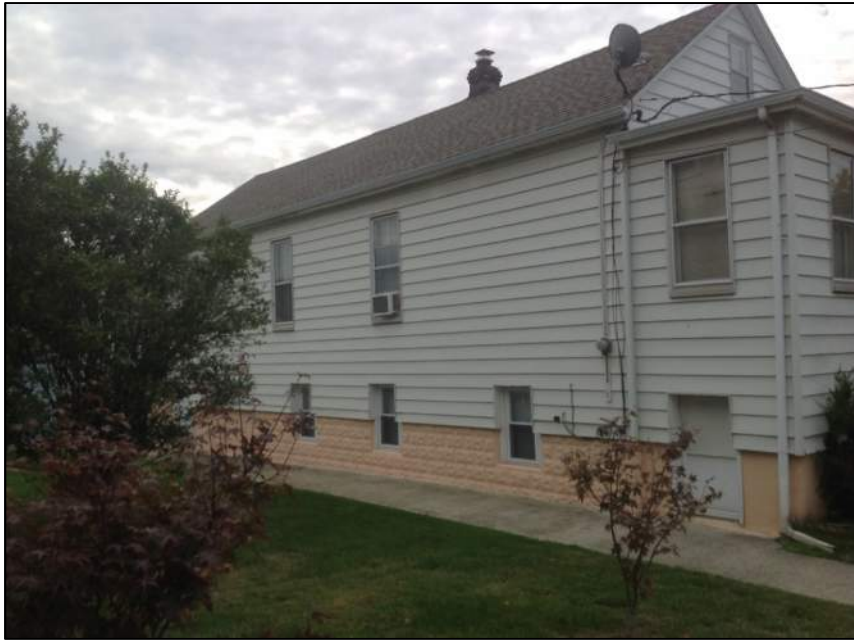
Photo 3: Left Side of House
