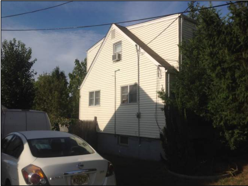
Photo 3: Left Side of House
