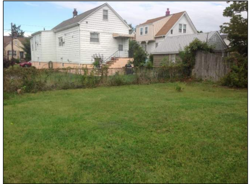
Photo 6: Backyard of Property
