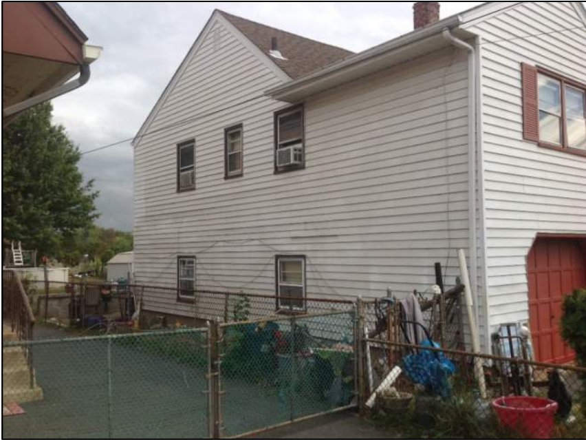
Photo 3: Left Side of House
