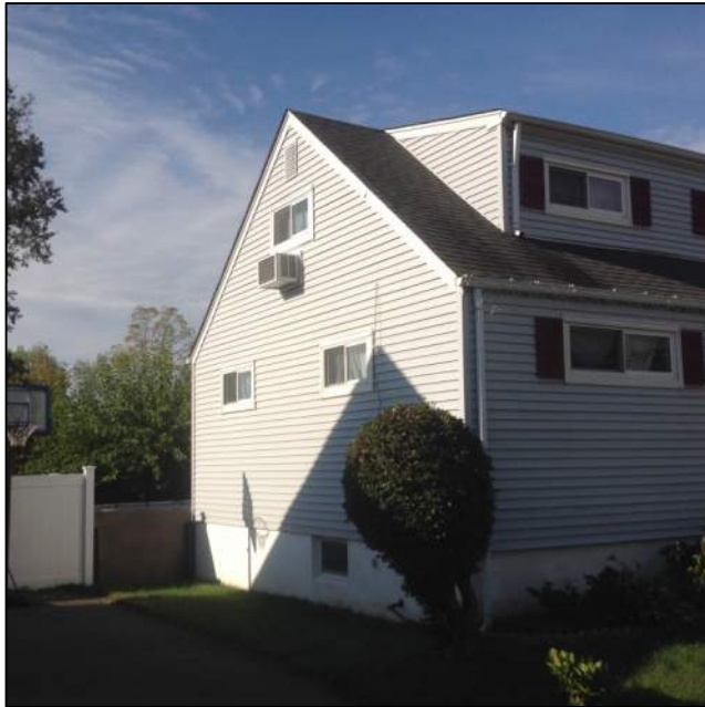
Photo 3: Left Side of House
