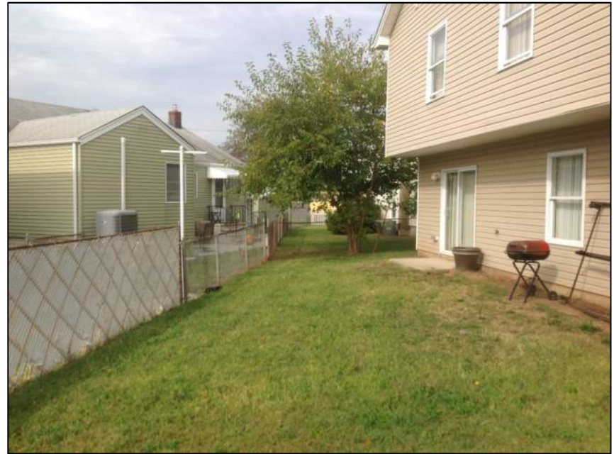
Photo 6: Backyard of Property
