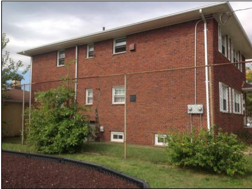
Photo 3: Left Side of House
