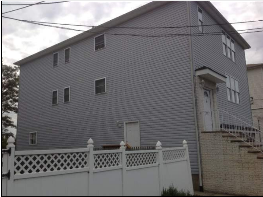
Photo 3: Left Side of House
