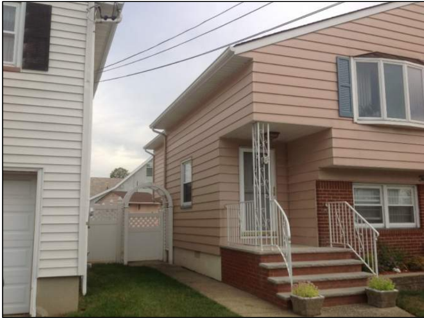
Photo 3: Left Side of House
