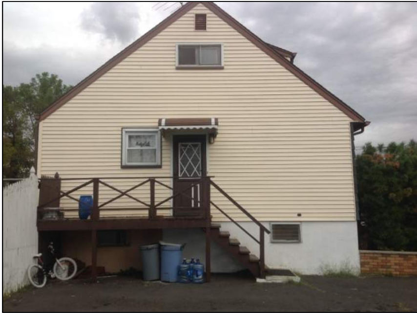
Photo 3: Left Side of House
