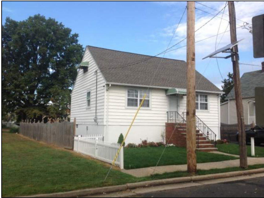
Photo 3: Left Side of House
