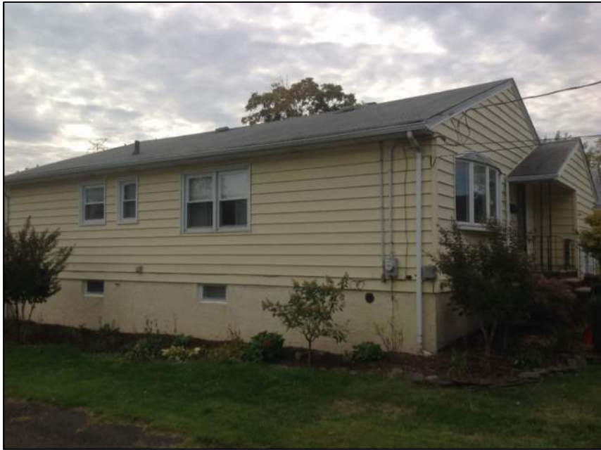
Photo 3: Left Side of House
