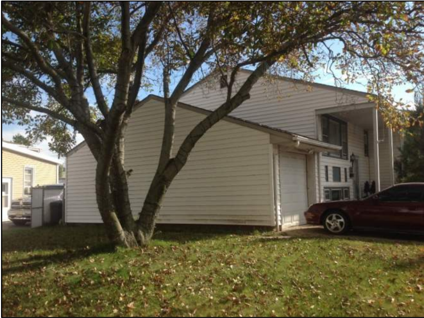
Photo 3: Left Side of House
