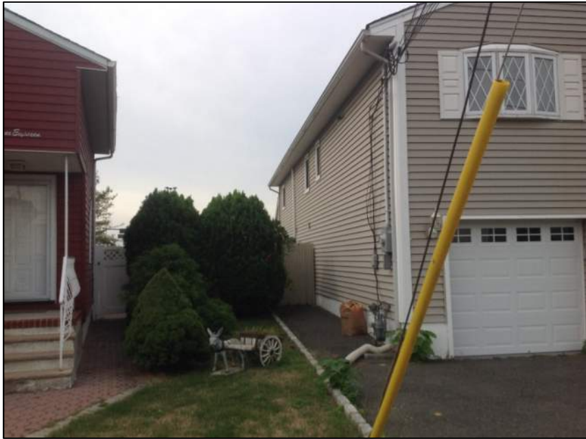
Photo 3: Left Side of House
