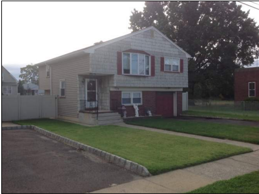
Photo 3: Left Side of House
