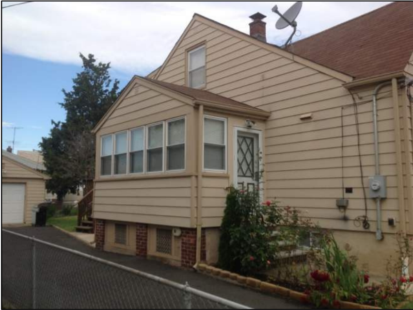
Photo 3: Left Side of House
