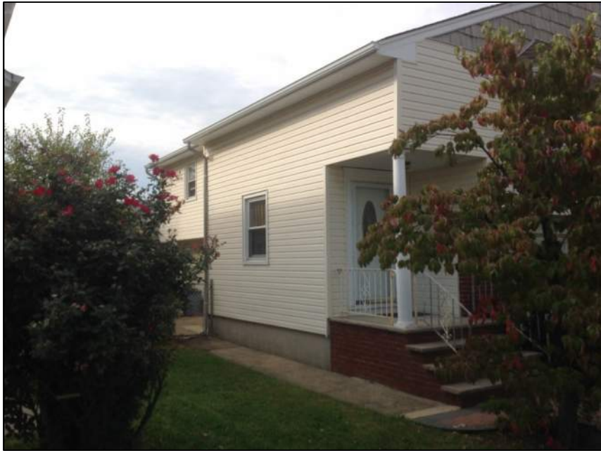
Photo 3: Left Side of House
