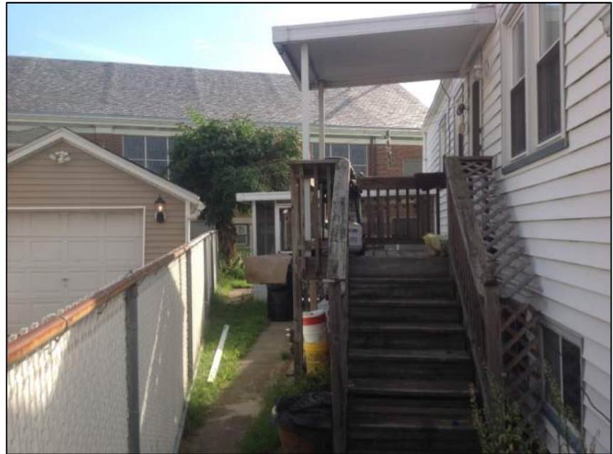
Photo 6: Backyard of Property
