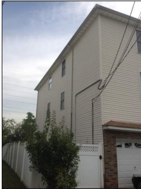
Photo 3: Left Side of House
