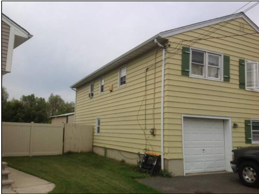
Photo 3: Left Side of House
