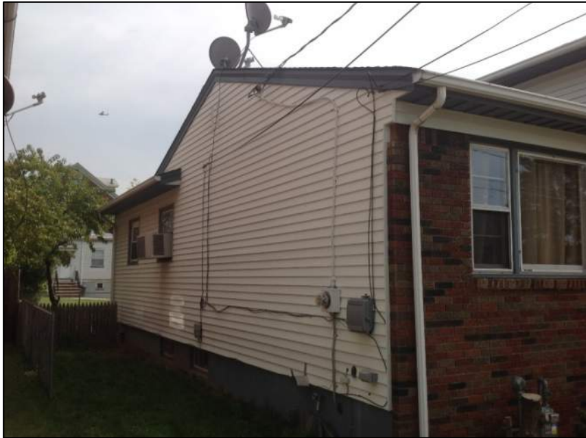
Photo 3: Left Side of House
