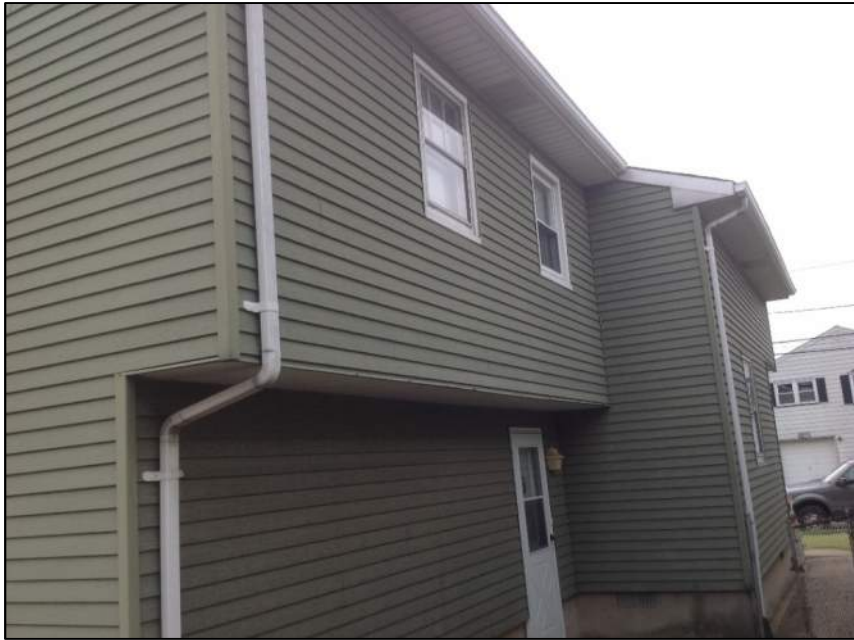
Photo 3: Left Side of House
