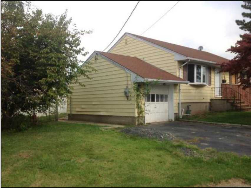
Photo 3: Left Side of House
