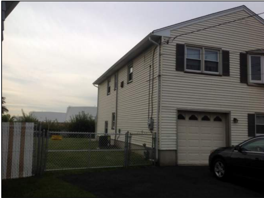
Photo 3: Left Side of House
