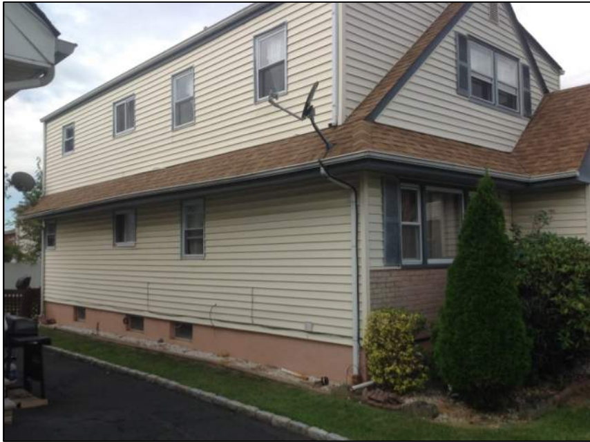
Photo 3: Left Side of House
