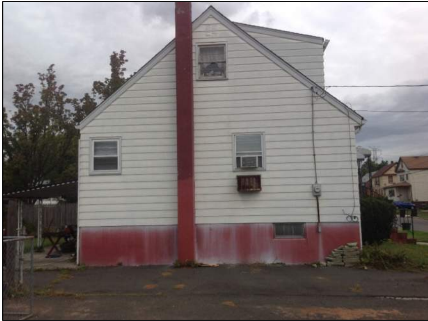
Photo 3: Left Side of House
