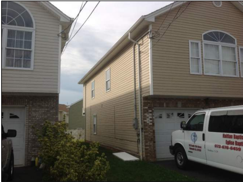
Photo 3: Left Side of House
