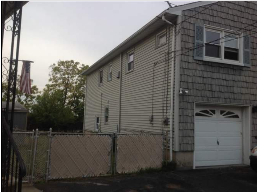
Photo 3: Left Side of House
