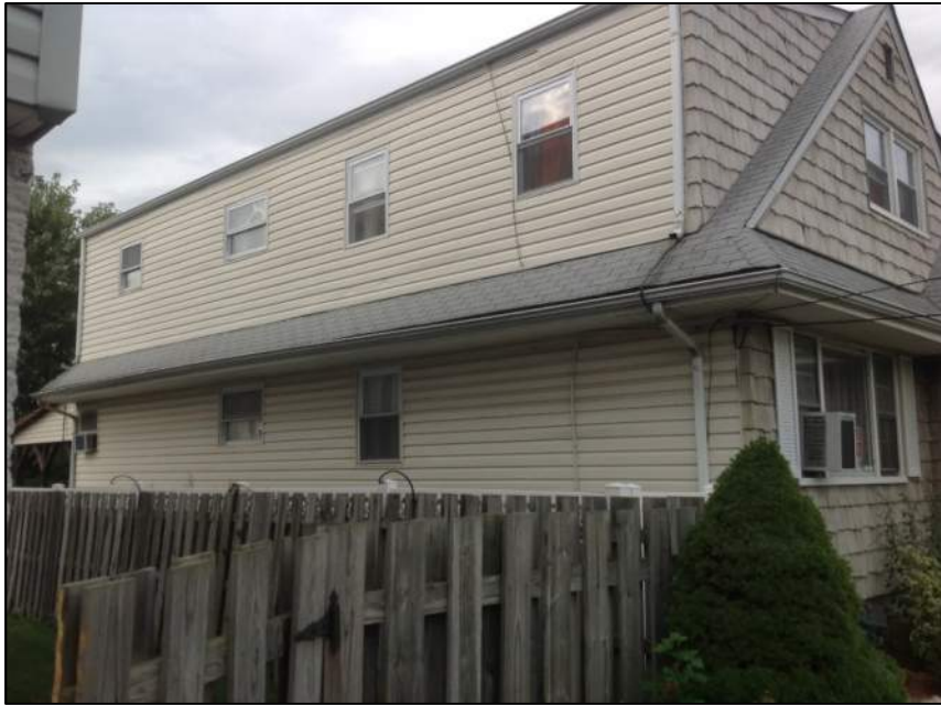
Photo 3: Left Side of House
