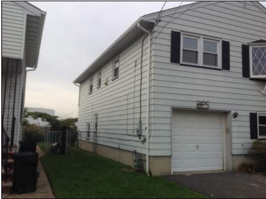
Photo 3: Left Side of House
