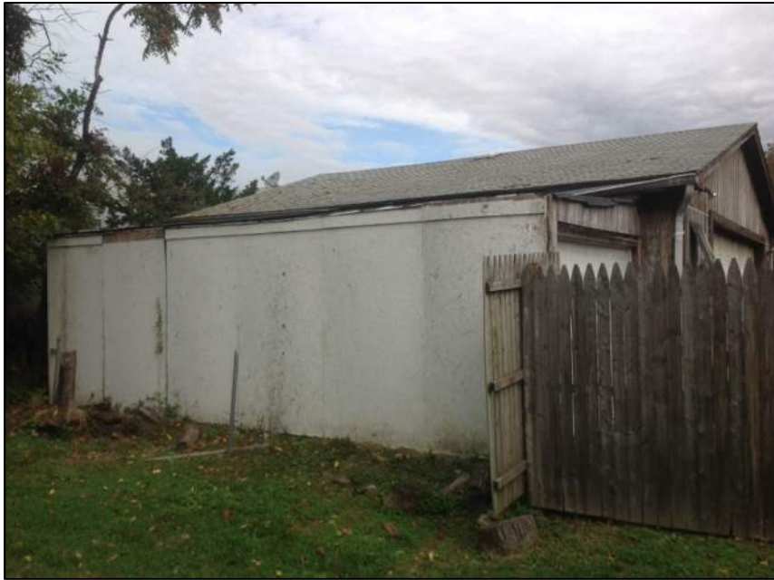
Photo 3: Left Side of Garage
