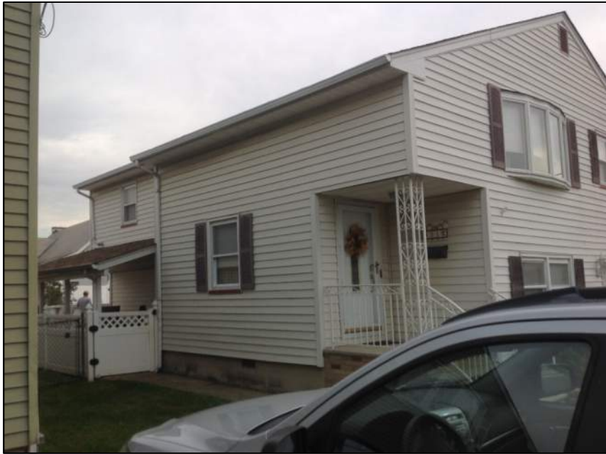
Photo 3: Left Side of House
