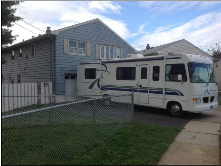
Photo 3: Left Side of House
