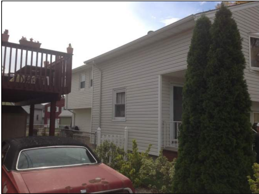
Photo 3: Left Side of House
