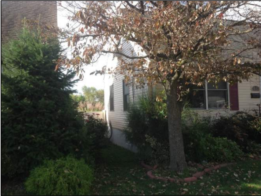
Photo 3: Left Side of House
