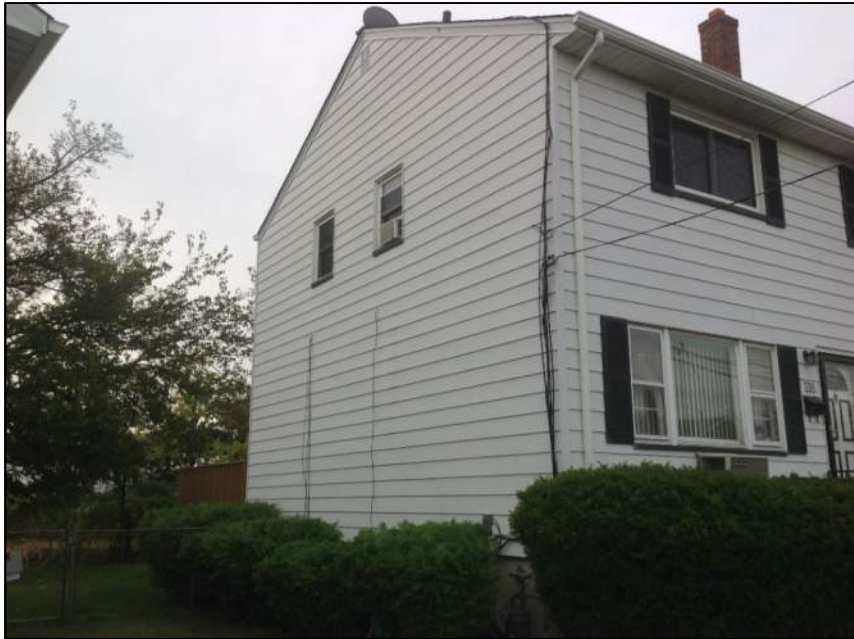
Photo 3: Left Side of House
