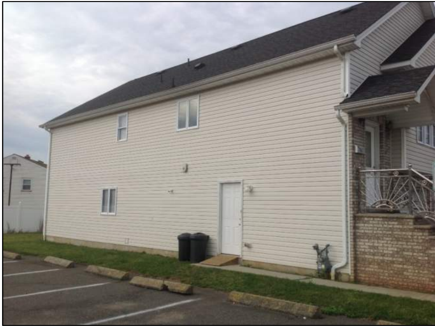
Photo 3: Left Side of House
