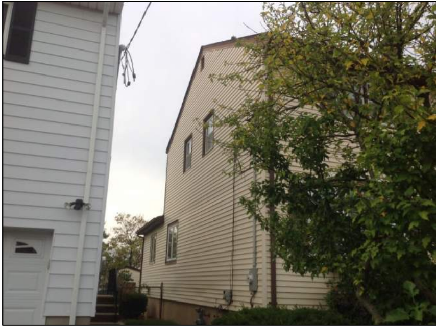
Photo 3: Left Side of House
