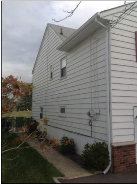
Photo 3: Left Side of House
