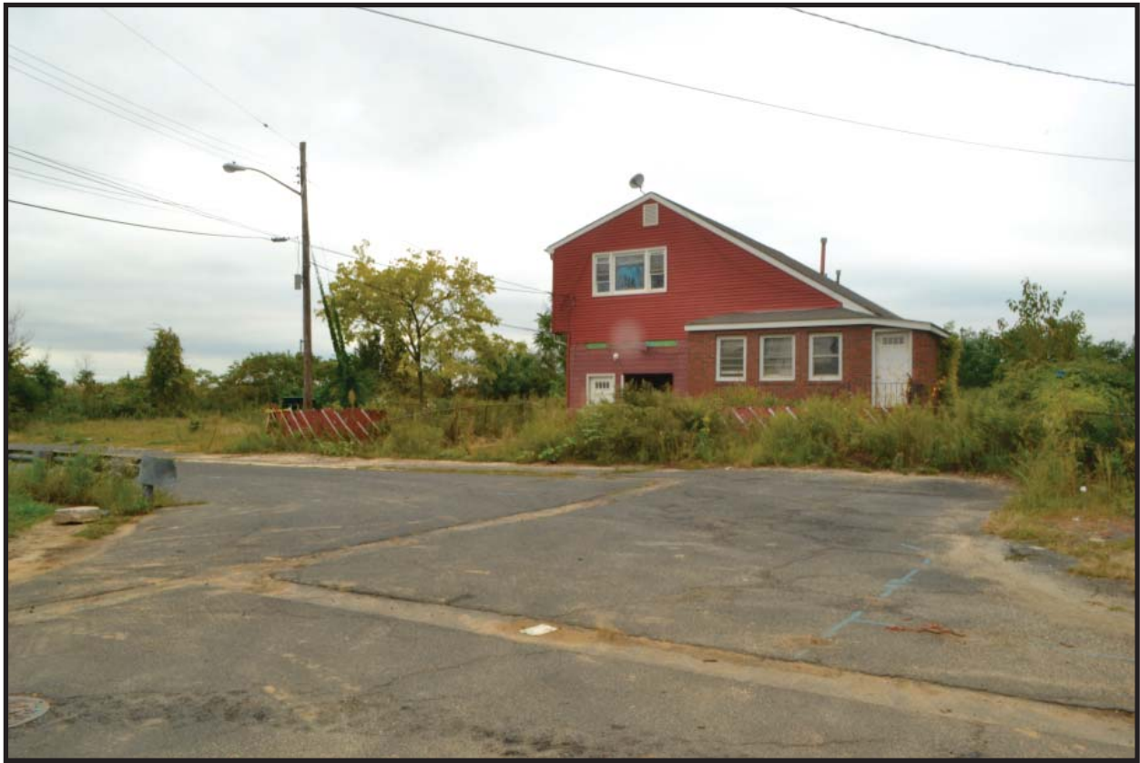
Photograph 3. View looking north from the intersection of Cliffwood Way and Bayshore Avenue, showing 14 Bayshore Avenue at photograph right (Photographer: Alison Haley, October 2, 2014) [HRI Neg. # 14042/D1:022].
