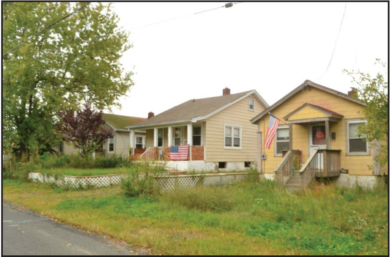
Photograph 1. View looking northeast towards the southeast side of Cliffwood Way, with 7 Cliffwood Way at photograph right (Photographer: Alison Haley, October 2, 2014) [HRI Neg. # 14042/D1:011].
