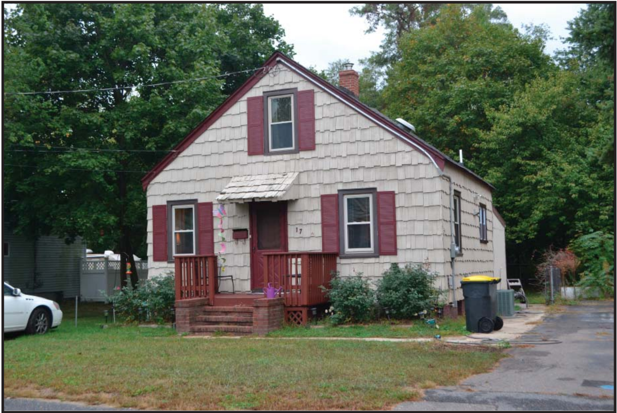
Photograph 12. View looking west towards the front (east) elevation of 17 Appleby Street (Photographer: Alison Haley, October 2, 2014) [HRI Neg. # 14042/D1:001].
