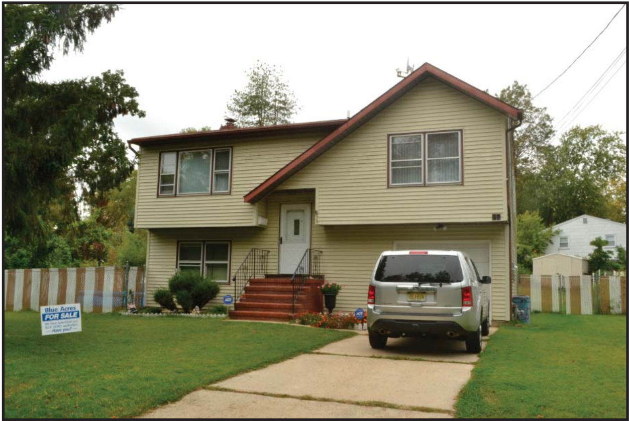
Photograph 9. View looking northwest towards the front (southeast) elevation of 75 Raritan Boulevard (Photographer: Alison Haley, October 2, 2014) [HRI Neg. # 14042/D1:050].
