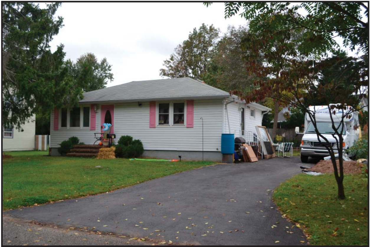
Photograph 8. View looking west towards the front (southeast) elevation of 71 Raritan Boulevard (Photographer: Alison Haley, October 2, 2014) [HRI Neg. # 14042/D1:045].
