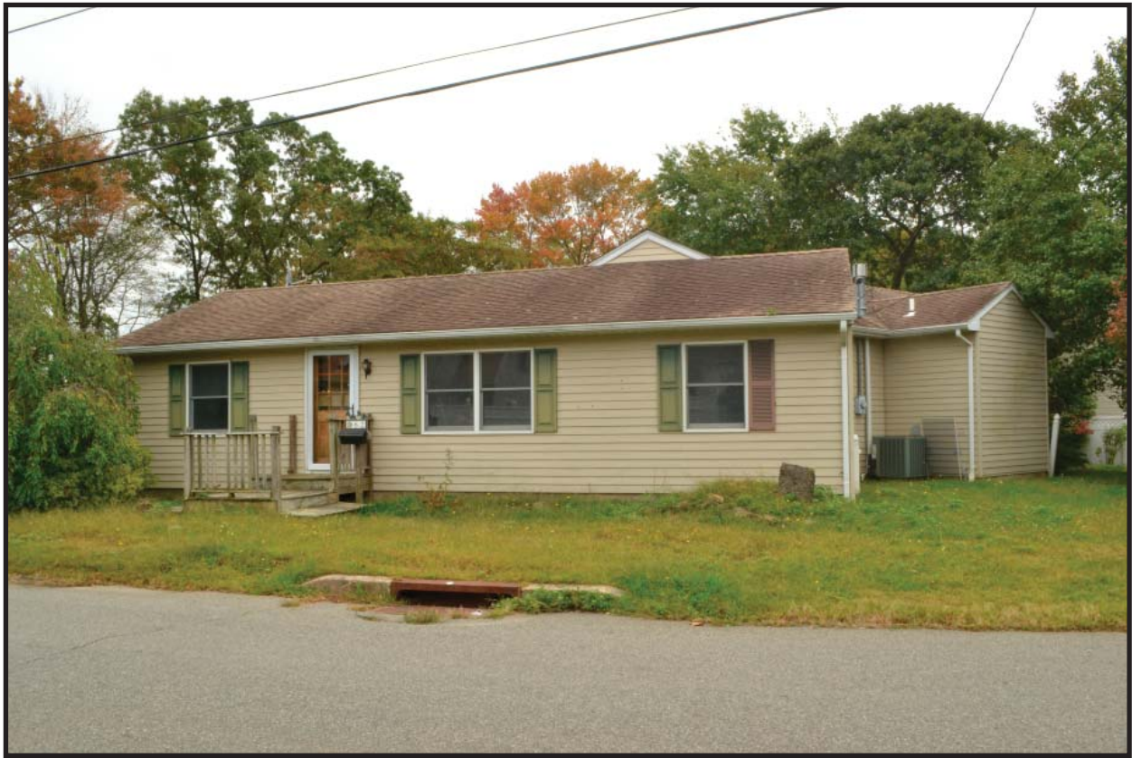
Photograph 10. View looking south towards the front (north) elevation of 62 Pomona Boulevard (Photographer: Alison Haley, October 2, 2014) [HRI Neg. # 14042/D1:051].
