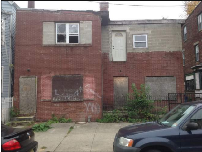
Photo 3: Front View – Building No. 1
