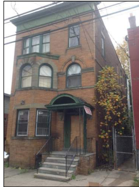
Photo 10: Right View – Building No. 2
