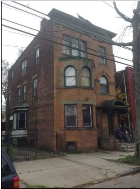
Photo 9: Left View – Building No. 2
