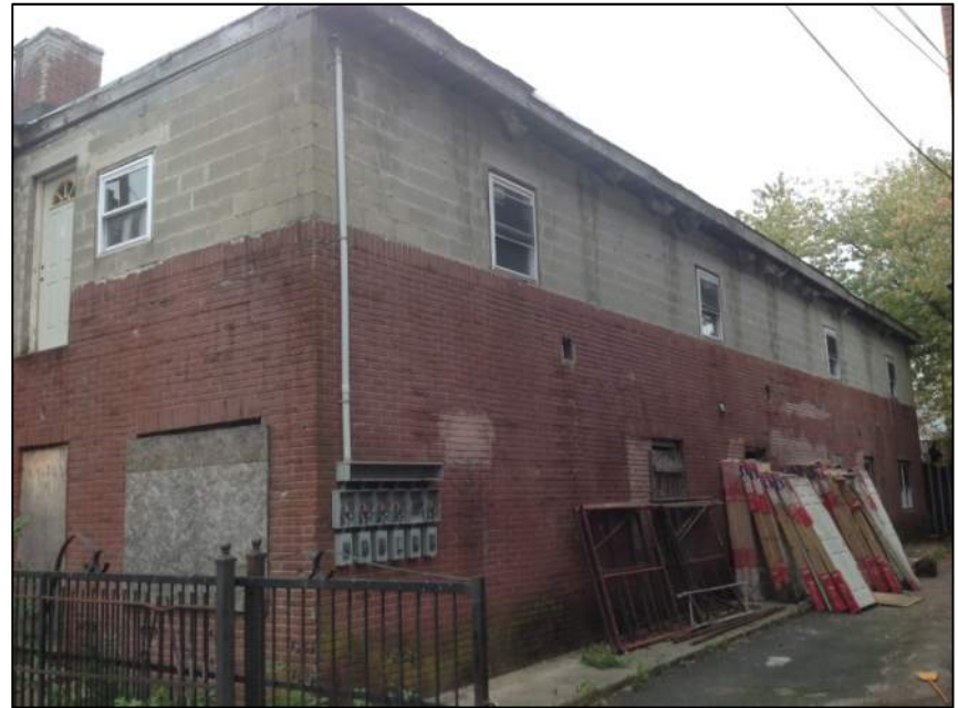
Photo 6: Right View – Building No. 1
