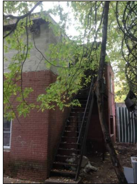
Photo 4: Rear View – Building No. 1
