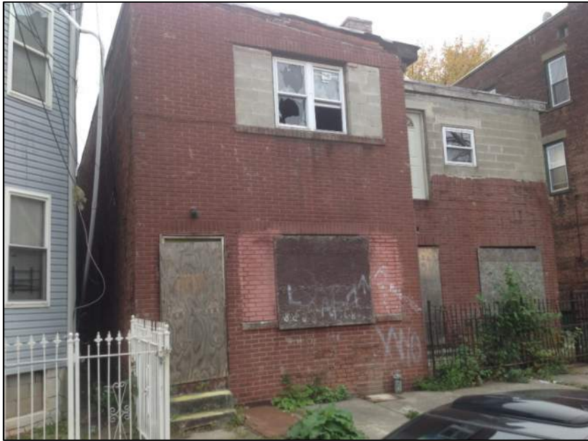
Photo 5: Left View – Building No. 1
