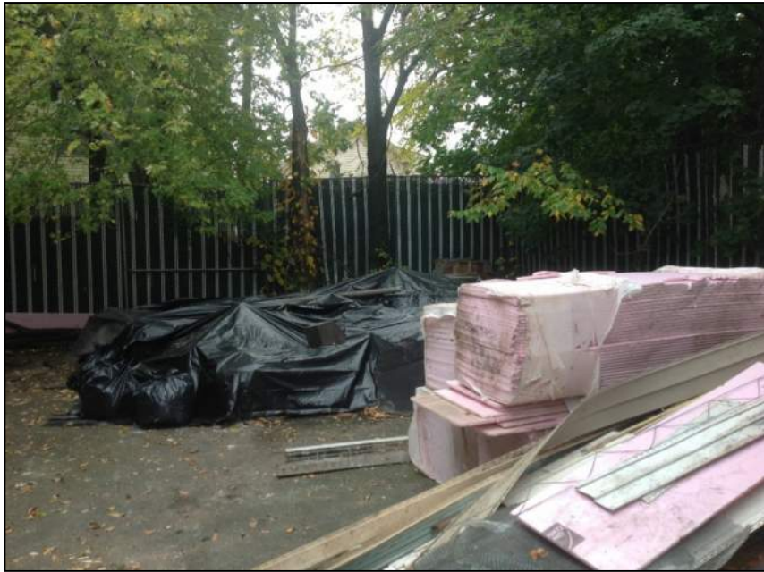
Photo 11: Backyard – Building No. 2
