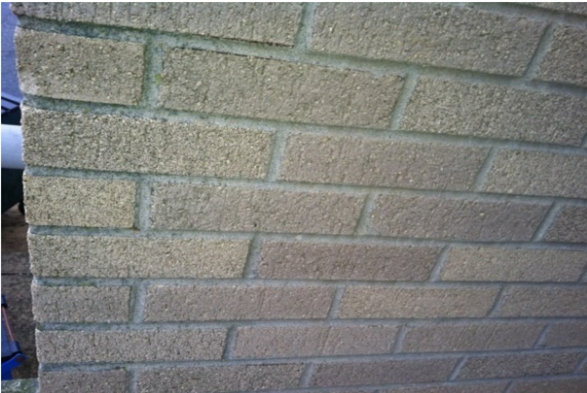
Photo 2: M-10 – ACM Brick Mortar (Court Section, Exterior)
