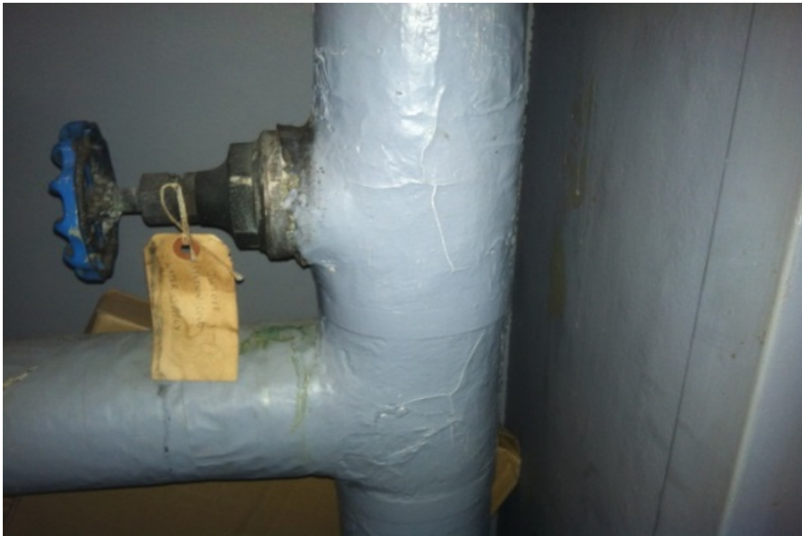
Photo 6: PACM Pipe Insulation – Hard Pack Elbows and Tees (Generator Room and Throughout)
