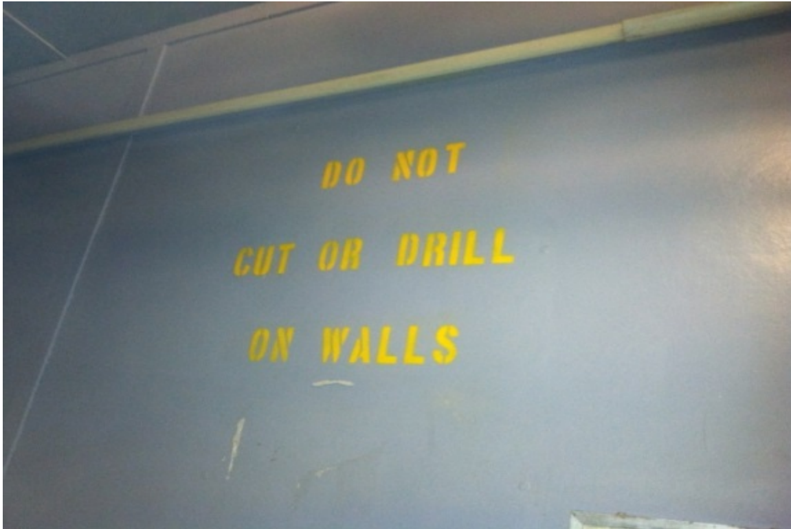
Photo 3: PACM Concrete Board (Generator Room)
