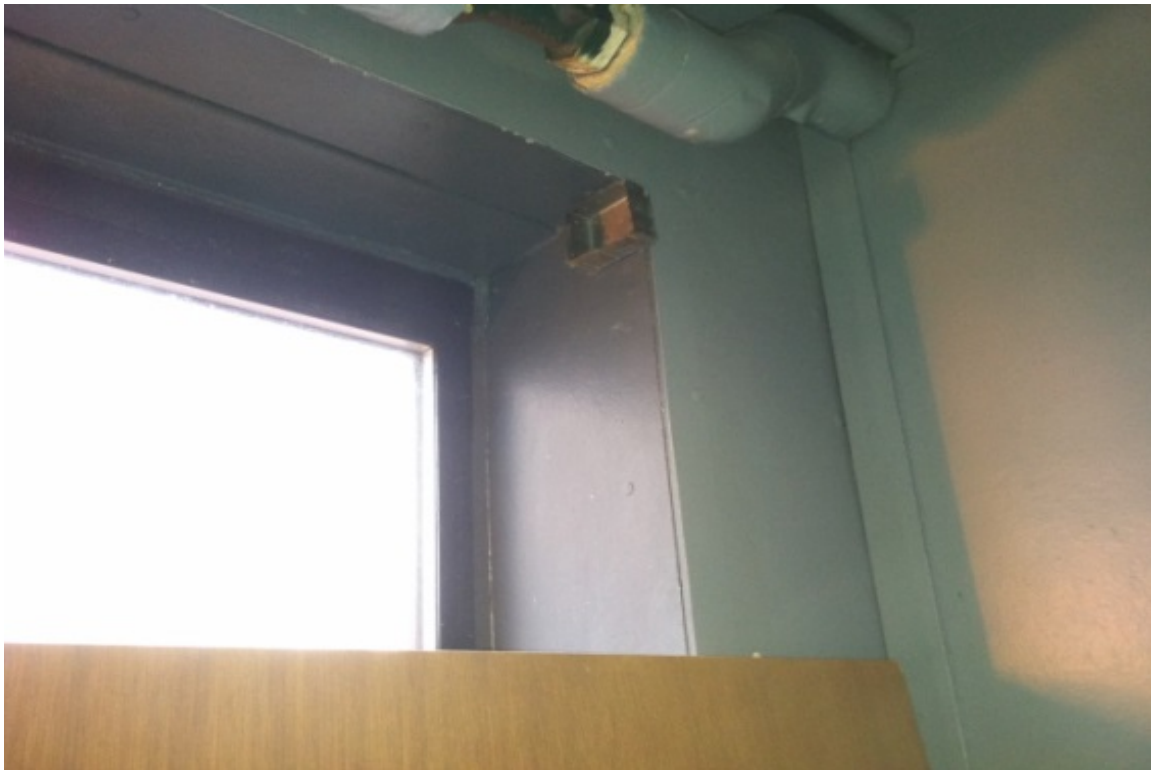
Photo 4: PACM Concrete Board (Generator Room)
