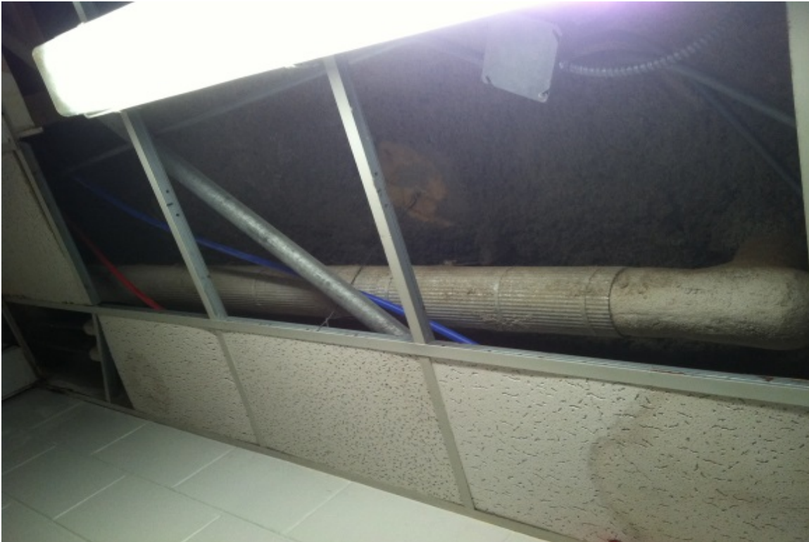
Photo 7: PACM Pipe Insulation – Hard Pack Elbows and Tees (Gym Bathroom and Throughout)
