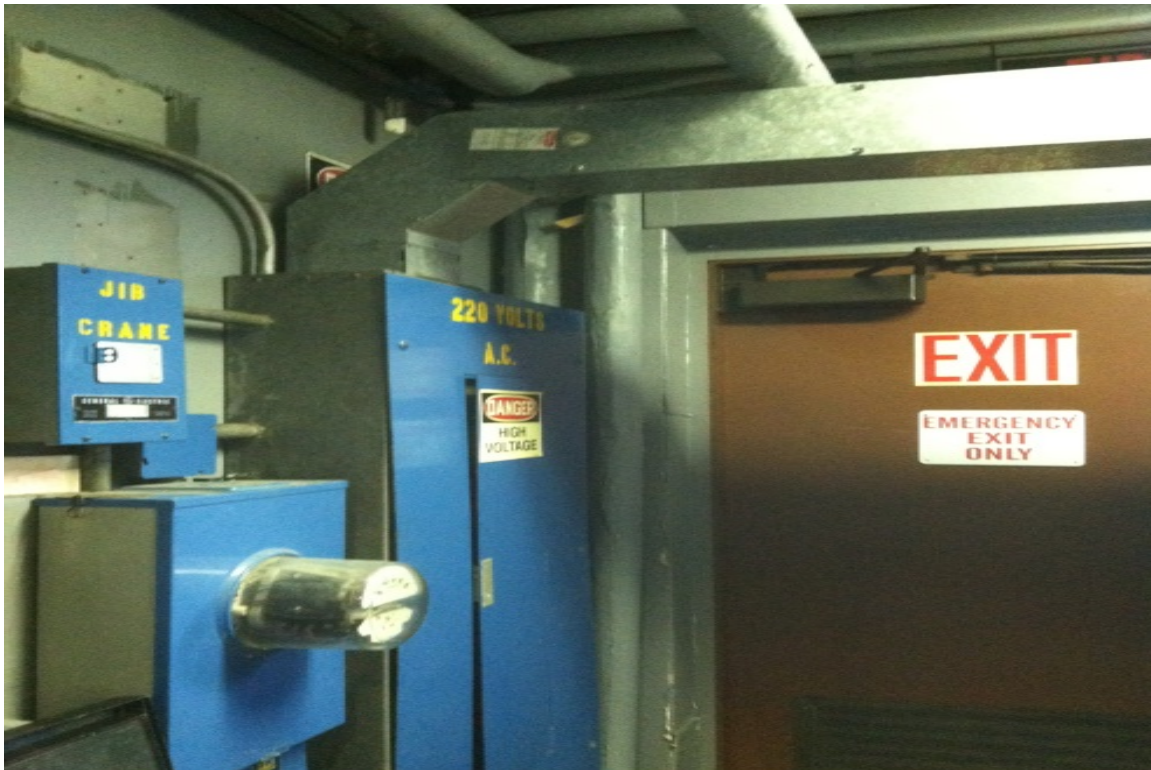
Photo 5: PACM Concrete Board and Pipe Insulation – Hard Pack Elbow and Tees (Generator Room)
