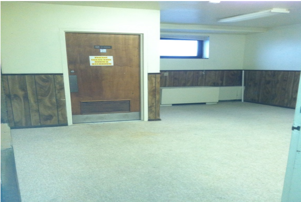
Photo 4: Room W106 – Lead Dust Hazard Location
