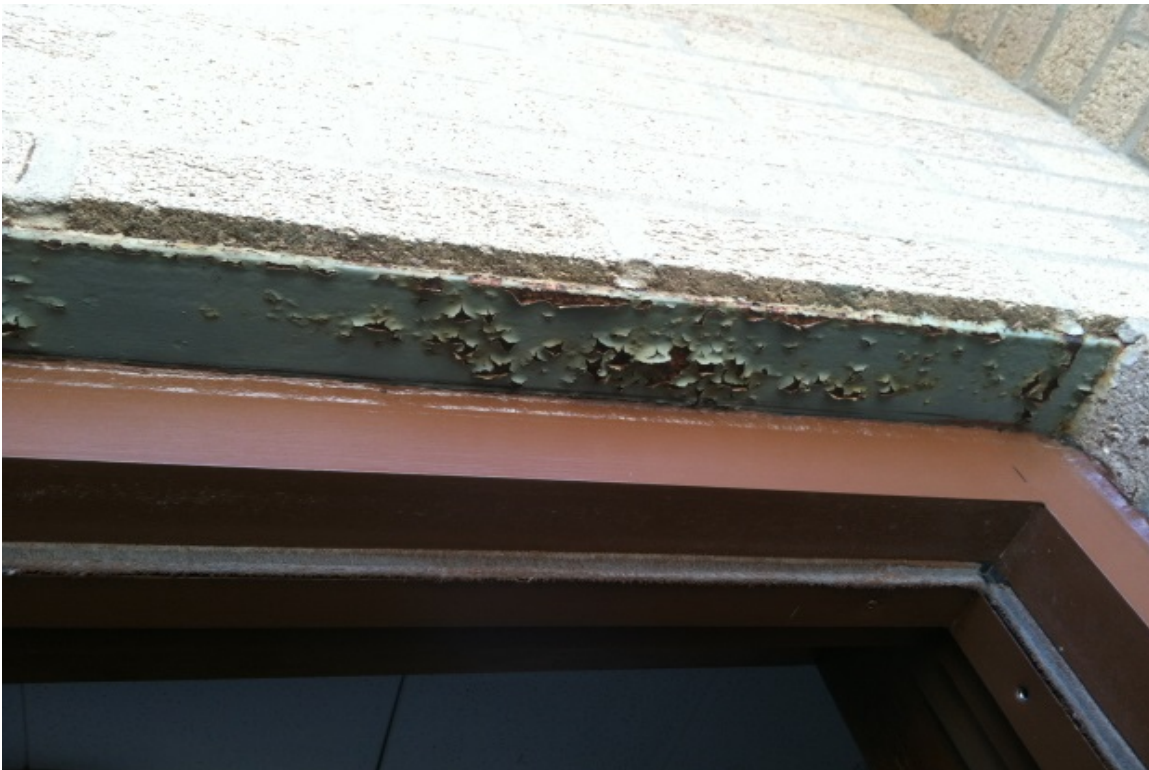
Photo 2: Four (4) LBP Door Lintels on Municipal Court Section
