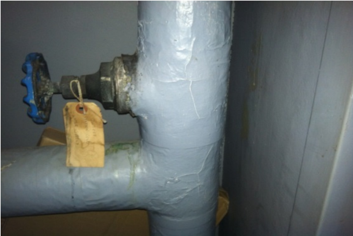
Photo 3: LBP Pipe Insulation
