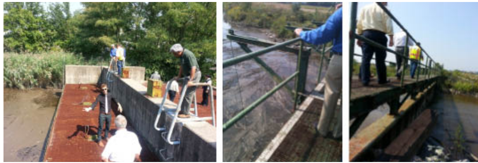
Figure 3-1: Physical Inspection of Existing Risk Reduction Infrastructure. Teams assigned by the New Jersey Department of Environmental Protection have endeavored to catalogue Superstorm Sandy’s impact on berms, tidal gates, and other existing risk-reduction infrastructure. Physical inspection is a key part of the State’s assessment of the current condition of measures to identify necessary repairs as well as opportunities to enhance existing measures to address future extreme weather events and maximize federal investment.
