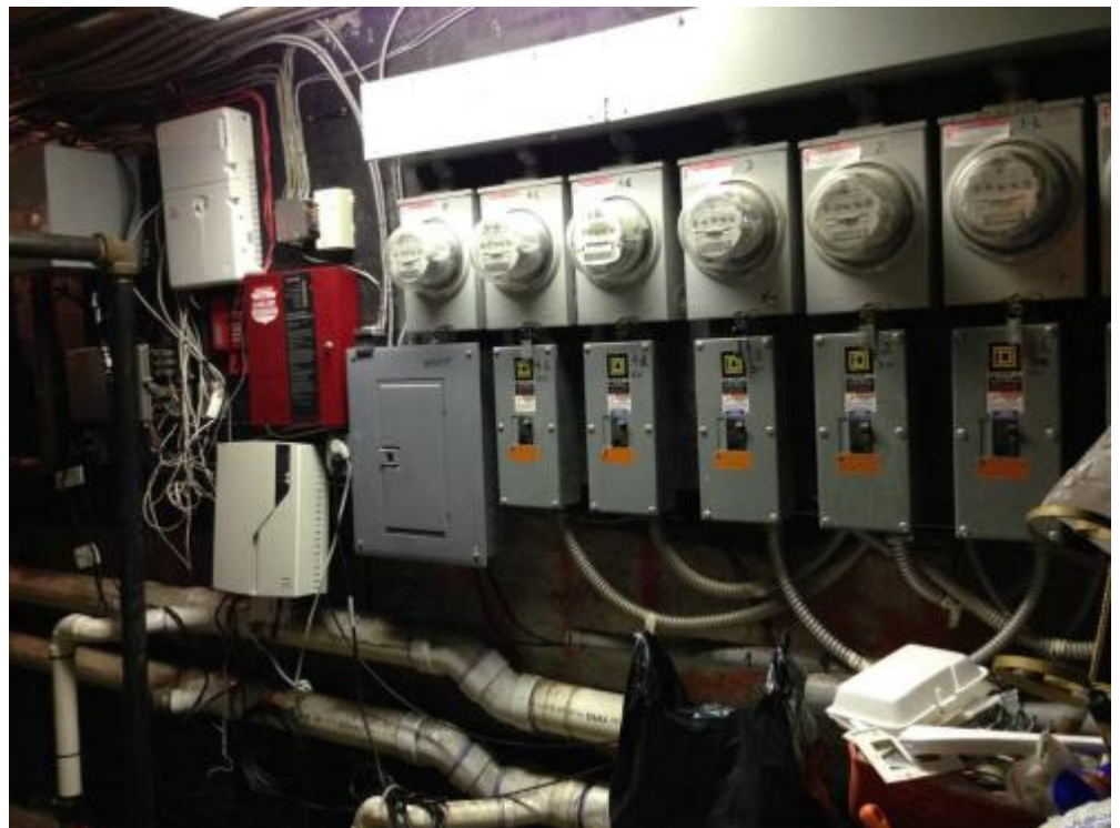
22 Main Level/Common Utility Room - RRE0032126_Common Ut Date Taken: 7/15/2014 Taken By: JLAM
