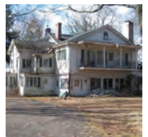
Suydam House , Piscataway Township, Middlesex County
