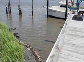
Shorelines are often stabilized with hardened structures. such bulkheads, revetment and concrete seawalls. Ironically, these structures often increase the rate of coastal erosion, remove the ability of the shoreline to carry out natural processes, and provide little habitat for estuarine species. Living shorelines use plants, sand and limited use of rock to provide shoreline protection and maintain valuable habitat.
