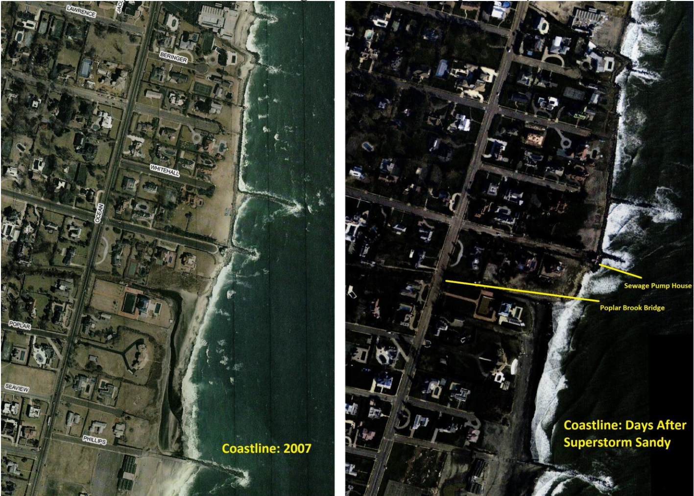
Figure 7: The Deal Coastline (From the Border with Long Branch South to Phillips Avenue) Before and After Superstorm Sandy
