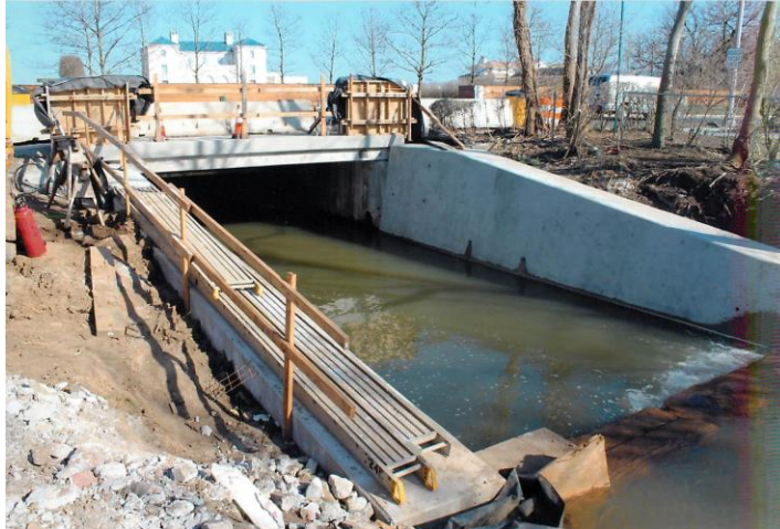
Figure 24: Poplar Brook Bridge during Repairs
