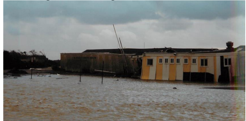
Figure 12: Flooding at the Conover Pavilion
