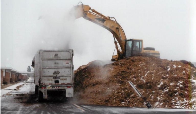
Figure 23: Debris is hauled away from the Deal Casino lot.
