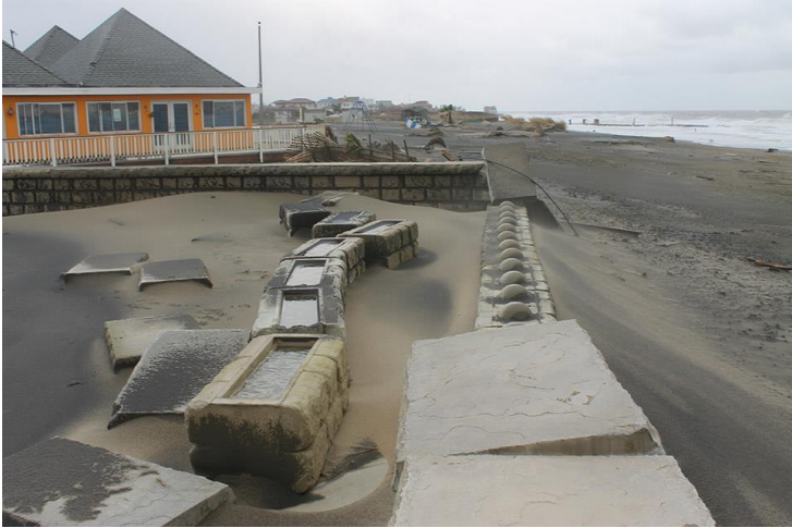
Figure 18: A Concrete Wall at the Deal Casino that was Knocked Over
