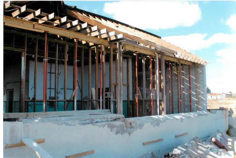
Figure 25: Repairs to the Pump Station Building's Eastern Wall
