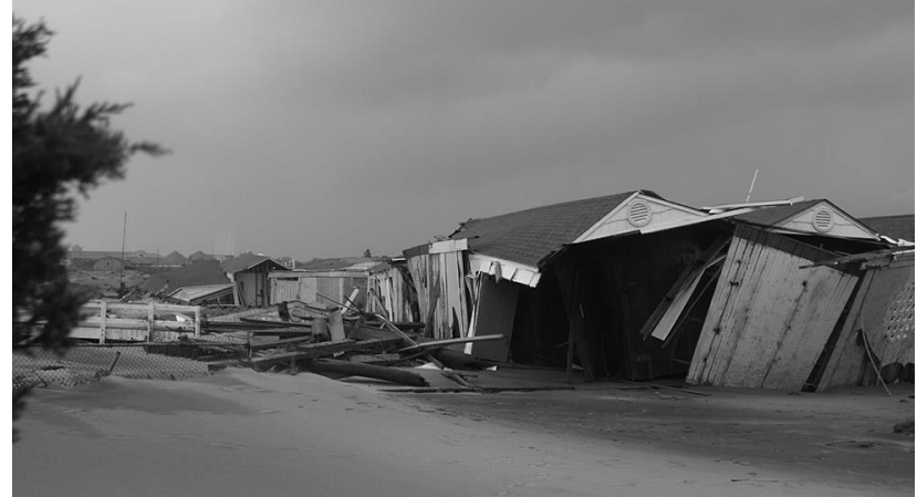
Figure 11: The Destroyed Conover Pavilion
