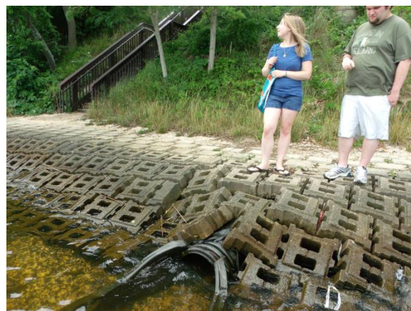
Figure 23: Location 1 Site 4 storm drain pictured with researchers Danielle Clancy and Kevin Dillon.
