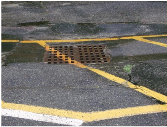
Figure 1: Storm drain located in the Beachwood Beach parking lot.
