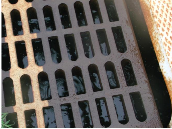
Figure 22: Sludge composition at the bottom of a Pine Beach storm drain.
