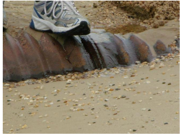
Figure 2: Storm drain with slight infrastructure problem. Water is leaking out of a crack in the drain.
