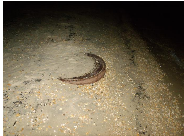
Figure 21: The manhole cover for the pipe at L2S2 at Avon Rd. West Beach.
