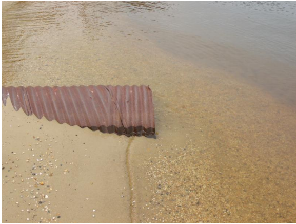
Figure 1: The stormwater pipe at Beachwood Beach.
