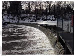
distance upstream, is a 248 foot long concrete arch dam constructed in 1919. The pond encompasses approximately 92 acres and serves as water supply for the City of New Brunswick under the control of the New Brunswick Water Utility.
