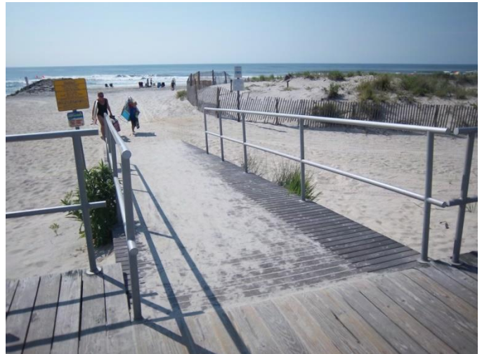
Boardwalk to Beach Access
