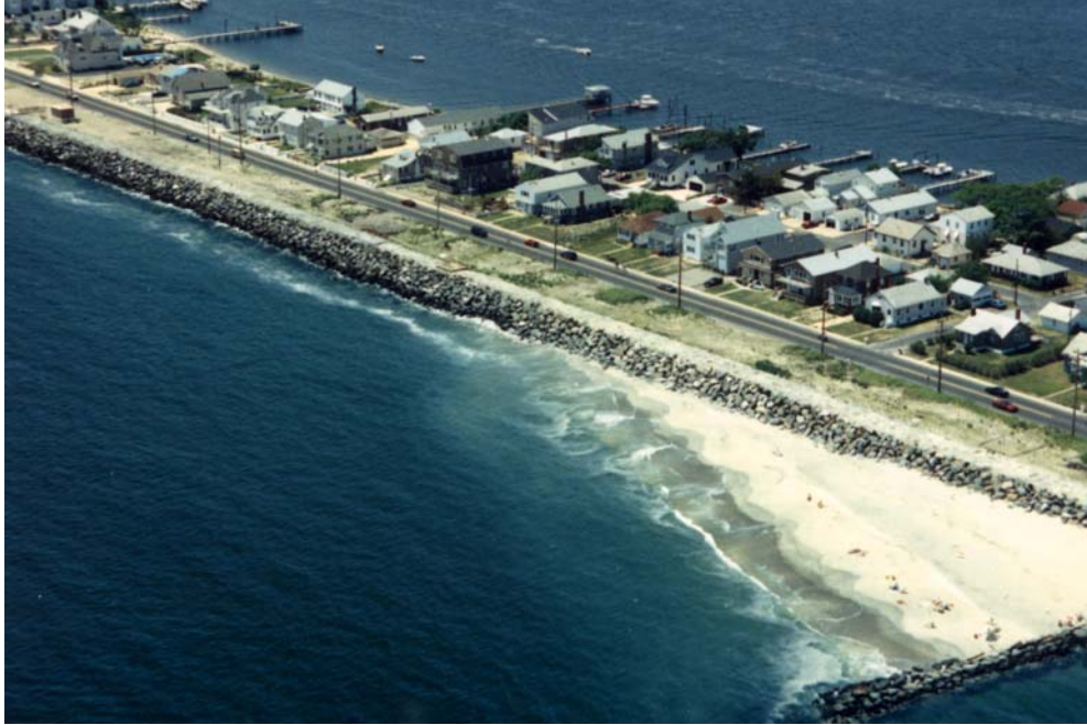
Figure 61. Sea Bright – Monmouth Beach Seawall in Monmouth County, New Jersey. Originally constructed to protect a rail line, the seawall now protects a main evacuation route and local community (Photograph courtesy of the Jersey Shore Partnership).
