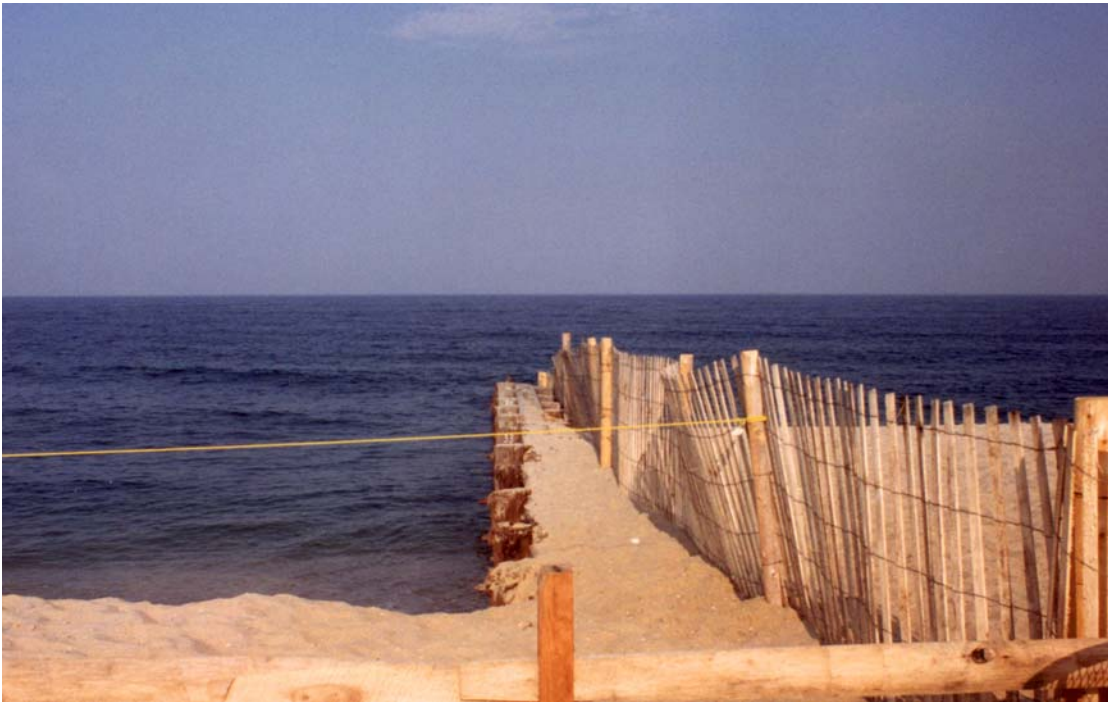
Figure 24. Localized erosion on the downdrift side of a timber groin in Manasquan, NJ, caused by prolonged unidirectional sediment transport (Photograph by Dr. Michael S. Bruno).
