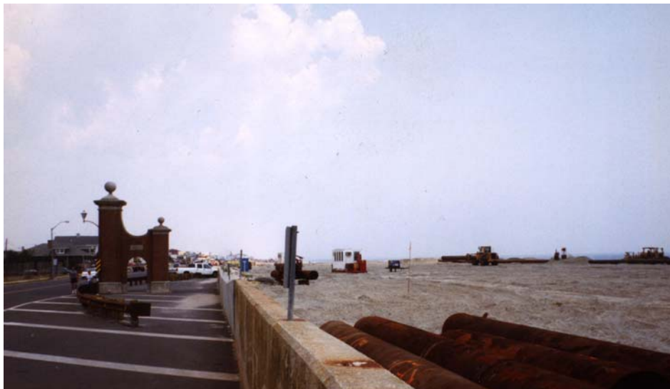
Figure 33. Belmar, NJ retaining wall shown in 1999 after the completion of a beach fill project designed to protect the coast from a 1 in 100 year storm event ( Photograph by Dr. Thomas O. Herrington).
