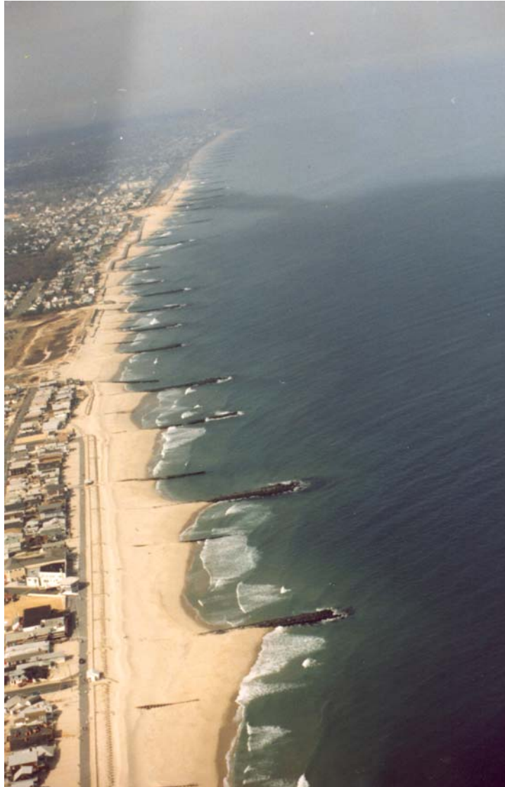
Figure 49. Extensive groin field along the Monmouth County, New Jersey coast. Note the recession of the shoreline from south (bottom of photo) to north as less and less sand is transported around each successive groin (Photograph by Ken Cadmus).
