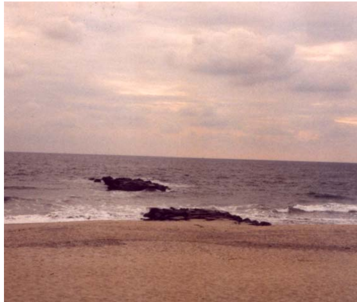
Figure 52. Notched groin – groin with a section removed within the surf zone, in Spring Lake, NJ. Photograph by Thomas O. Herrington.
