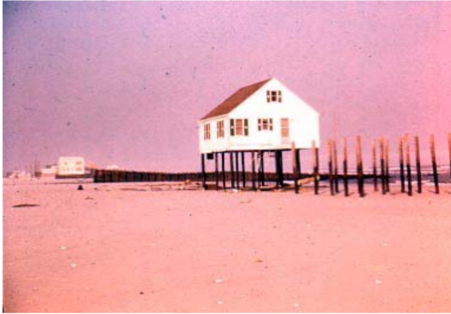
Figure 44. House on pilings left standing after March 1962 northeaster in Holgate, New Jersey. Almost all oceanfront houses not on pilings were either destroyed or heavily damaged as a result of this storm. The pilings to the right of the houses had just been driven in anticipation of building. The comparison between those houses left standing and those destroyed led to changes in FEMA's construction code (Photograph by Lawrence Wagner; courtesy of Dr. Susan D. Halsey)
