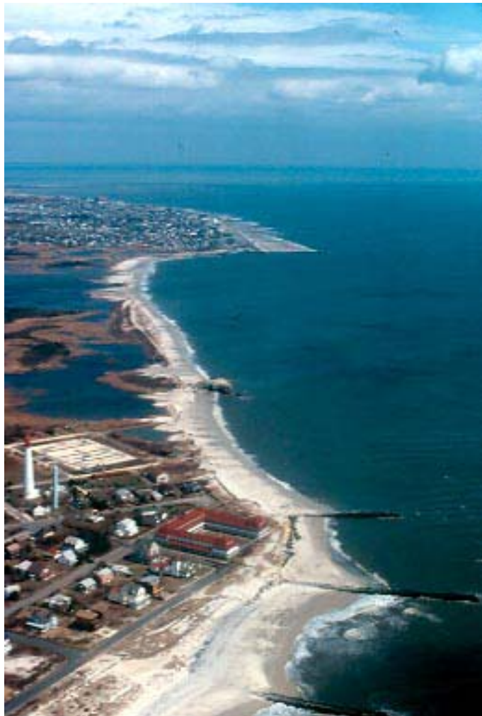
Figure 55. Aerial photograph of the “Cape May Meadows” area, Cape May Point, NJ after the March 1984 storm. Terminal groin effect from Cape May City (in top distance) has eroded the meadows area in the classical arced pattern. Note extensive washover fans with sand reaching into the ponds and salt marsh, and old World War II bunker in surf zone. Originally the bunker was approximately 1000 feet behind the dune line when built. (Photograph by Dr. Susan D. Halsey)
