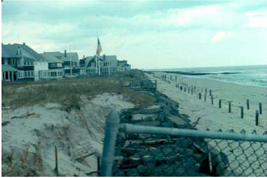
Figure 68. Exhumed portion of small rock seawall under dunes in northern section of Bay Head, New Jersey after a severe storm. Many residents were unaware that this seawall existed because it was completely covered by extensive dunes (Photograph by Dr. Susan D. Halsey).
