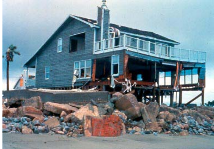
Figure 16. Extensive wind damage to house near Myrtle Beach, South Carolina as a result of Hurricane Hugo. Note loss of not only front plate glass windows, but also loss of side windows (Photo courtesy of Dr. MaryJo Hall).
