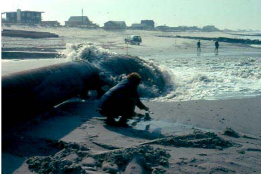
Figure 37. Emergency beach nourishment project underway on Long Beach Island, NJ, March 1979. Sand from Barnegat Inlet was pumped through pipes at two locations; one further up the beach profile and one near the proposed low tide line. Note pipes on upper beach waiting for placement near the dune scarp created by a trio of northeasters in the winter of 1978-1979. After the nourishment project, groins seen in this photograph were not visible. (Photograph by Dr. Susan D. Halsey)
