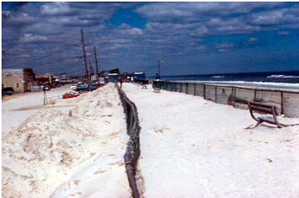
Figure 34. Ortley Beach, New Jersey after a severe storm. Significant erosion of sand from the beach overwashed the boardwalk and was deposited onto local streets. The piles of sand just landward of the boardwalk resulted from post-storm bulldozing of the streets (Photograph by Dr. Susan D. Halsey).
