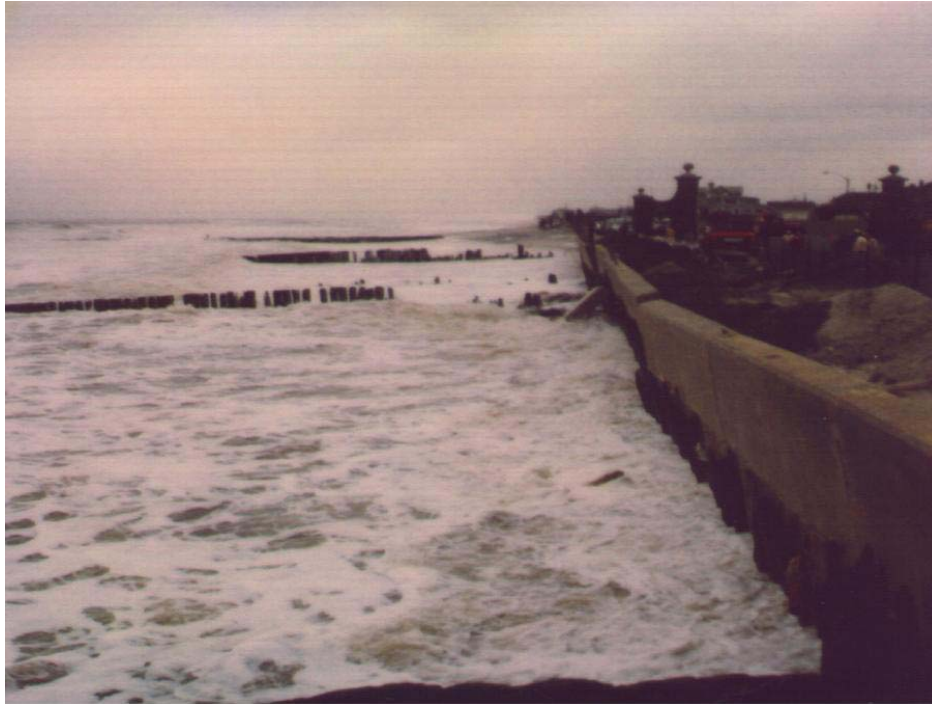
Figure 32. Concrete retaining wall, originally constructed to prevent wind blown sand from depositing on Ocean Avenue, in Belmar, New Jersey, under direct wave attack during the October 31, 1999 northeaster (Photograph by Dr. Michael S. Bruno).
