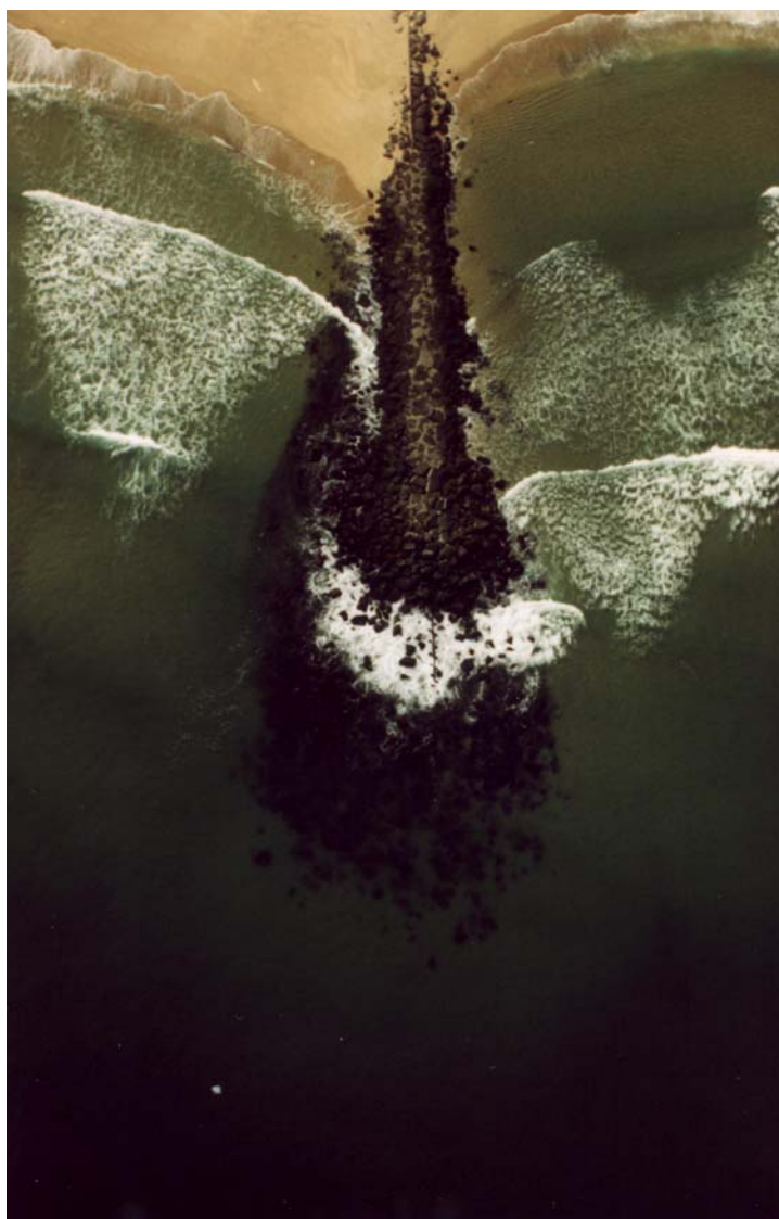
Figure 50. Overhead view of a rock groin showing the underwater extent of the structure (Photograph by Ken Cadmus).
