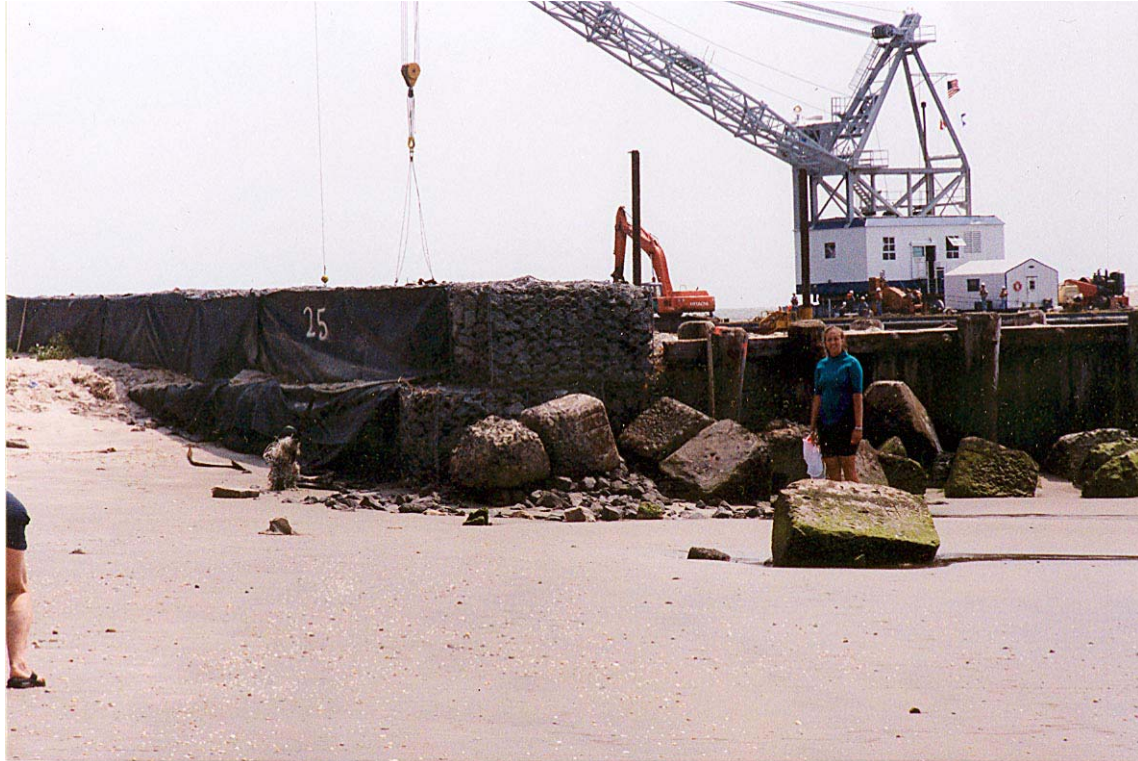
Figure 60. “Flanking” around the end of a gabion revetment in Cape May Point, New Jersey (Photograph by Dr. Thomas O. Herrington).
