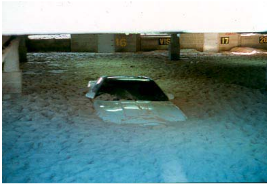
Figure 35. Underground parking garage with partially buried vehicle in Point Pleasant Beach, New Jersey in the aftermath of the December 1992 northeaster. The ripple marks on the top of the sand indicate active water flow (Photograph by Dr. Susan D. Halsey).
