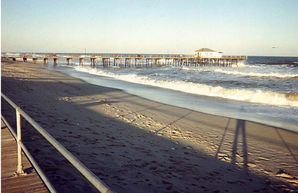
Figure 10. Large waves passing under a piling supported pier in Ocean Grove, New Jersey (Photograph by Dr. Thomas O. Herrington).
