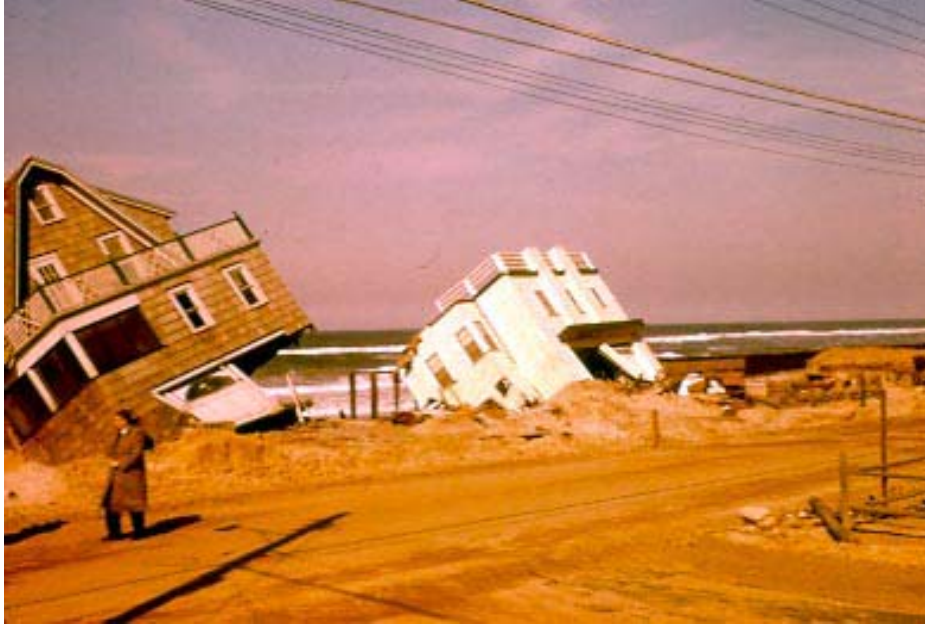
Figure 8. Brant Beach section of Long Beach Island, New Jersey after the March, 1962 storm. Houses with regular foundations undermined by wave scour on the oceanfront, cinder blocks failed and houses tipped down the scarp (cliff) toward the ocean. The number of damaged homes from this storm led to FEMA subsequently requiring houses in specific zones to be built on pilings (Photo by Al Chance, courtesy of Dr. Susan D. Halsey).
