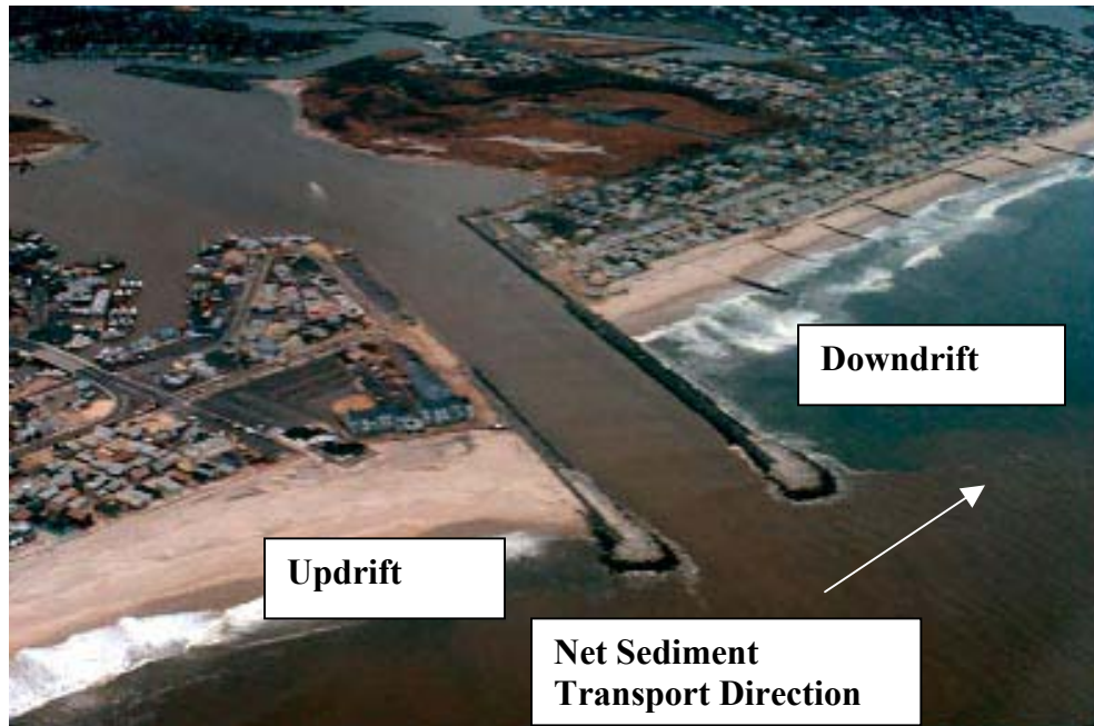
Figure 30. Sediment offset at Manasquan Inlet, New Jersey. Note sediment build-up on south (updrift) side of the inlet along Point Pleasant Beach, and sediment deficit on the north (downdrift) side of the inlet at Manasquan. Average alongshore current direction in this area is to the north (Photo by Dr. Susan D. Halsey).
