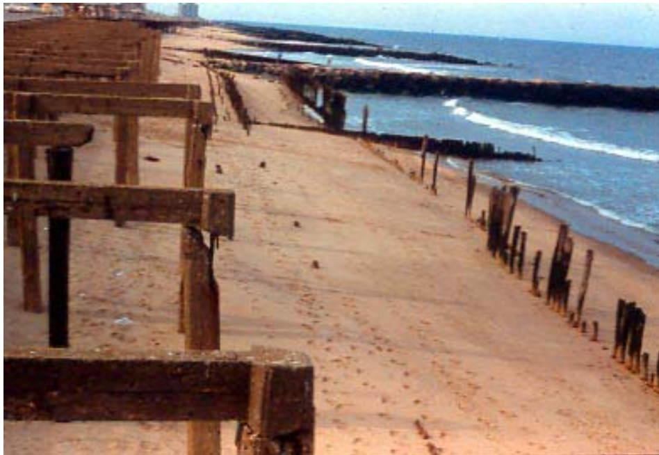
Figure 46. Long Branch, New Jersey in May 1983 showing the location of old shore protection structures exhumed by storm action. (Photograph by Ed Schwartz, Toms River, New Jersey)
