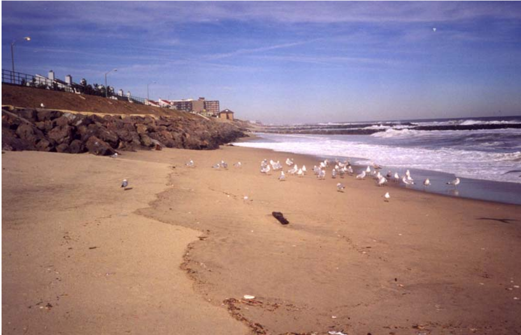
Figure 31. Stone and concrete revetment placed along an eroding bluff in Long Branch, NJ. Although the structure stops erosion, it also reduces the natural sediment supply to the beach (Photograph by Dr. Michael S. Bruno).
