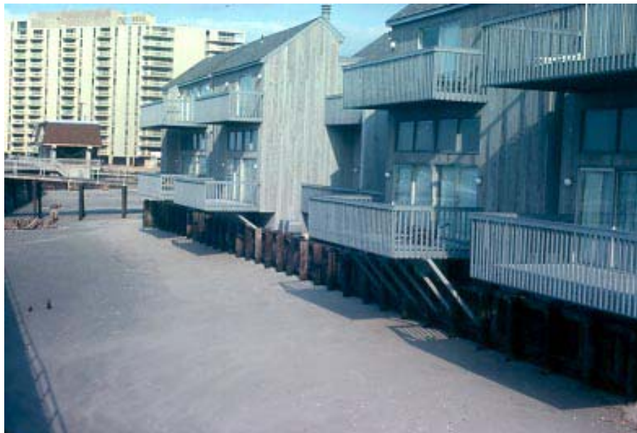
Figure 14a. Brighton Beach Condominiums with decks overhanging primary bulkhead, 5 th Street, Ocean City, New Jersey prior to March 28-29, 1984 northeaster. Storm waves lifted up the decks that had been tied into the interior of the house damaging the entire living rooms. The City condemned the buildings until the structure of the units were repaired, and passed an ordinance that prohibited decks to be tied into the main part of the house. Decks now have to be freestanding (Photo courtesy of Dr. Susan D. Halsey).
