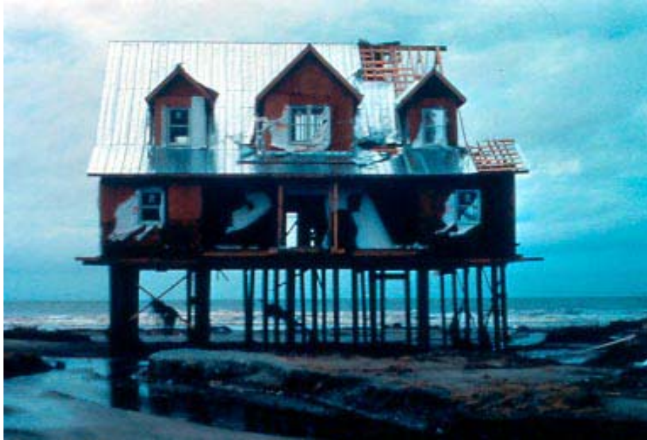
Figure 7. Extensively damaged home south of Litchfield Camp, South Carolina as a result of Hurricane Hugo. In addition to the heavy damage to the structure of the building itself from wind and wave damage, note evidence of wave-induced erosion and scour under the house and around pilings and creation of channels toward the viewer (Photo courtesy of Dr. MaryJo Hall).
