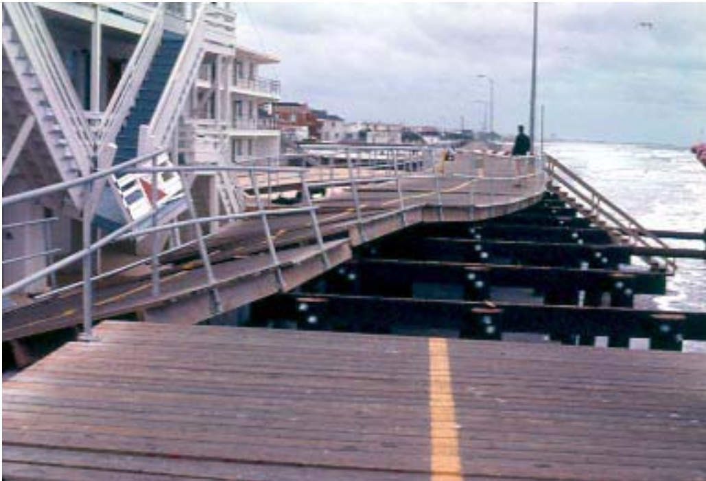
Figure 12. Damage to the Ocean City, NJ boardwalk from Hurricane Gloria, September 1985. This damage was caused by waves reflecting off the adjacent bulkhead, lifting up sections of the boardwalk and moving the loosened section landward (Photo courtesy of Dr. Susan D. Halsey).
