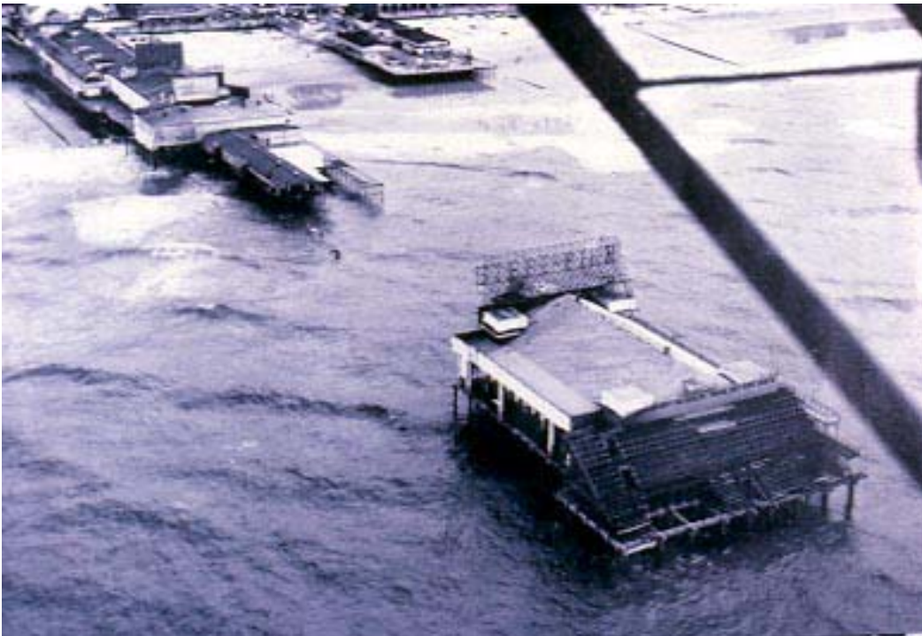
Figure 11. Damage to Atlantic City's Steel Pier from the March, 1962 storm. Note missing center portion removed by wave uplift during the height of the storm (Photo courtesy of Dr. Susan D. Halsey).
