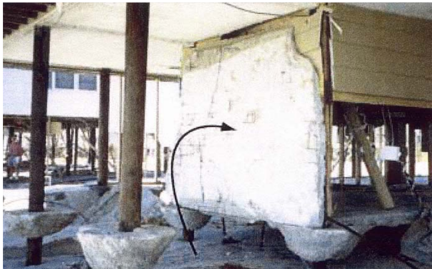
Figure 26. Scour around pilings and under on-grade slab. Notice that the slab broke free of the pilings and flipped up vertically. Poured concrete under a pile supported structure can generate unexpected loads on the structure, if undermined like above. Reprinted with permission from the FEMA Coastal Construction Manual (FEMA, 2000).
