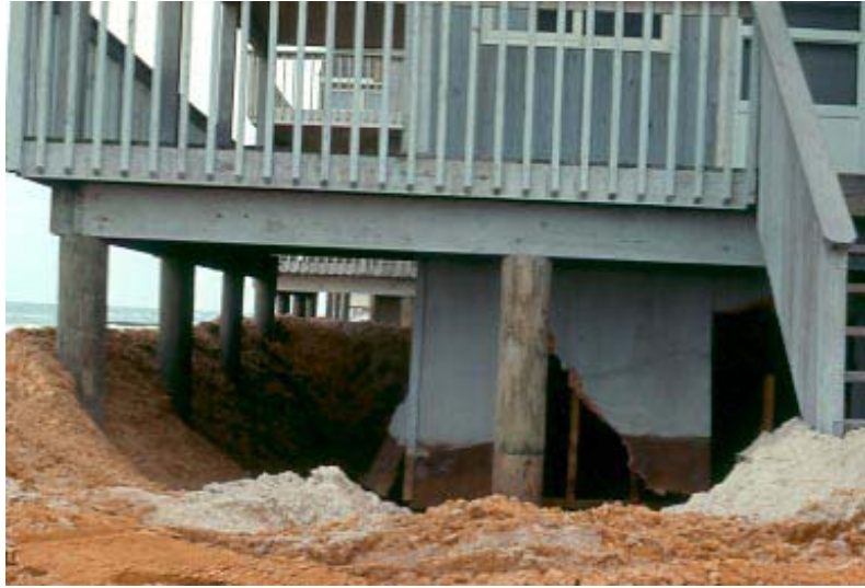
Figure 1. Damage to breakaway walls under an oceanfront house in Brant Beach, Long Beach Island, as a result of a storm in December 1992. Note hole in wall facing the viewer and buckle in wall out to the ocean side due to hydrostatic load (Photo courtesy of Dr. Susan D. Halsey).
