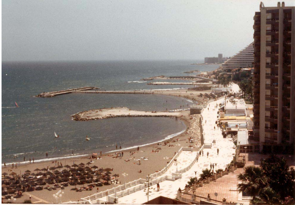
Figure 63. Engineered beachfront in Malaga, Spain. The Spanish provincial government has created beach reentrants with large T-groins and smaller interior bulbous-ended groins tied together by a wide promenade (right) along extensive sections of the Spanish Mediterranean coast. These designs are created to provide protected beaches and bathing areas for recreation, and shops and restaurants for the burgeoning tourist industry (Photograph by Dr. Susan D. Halsey)
