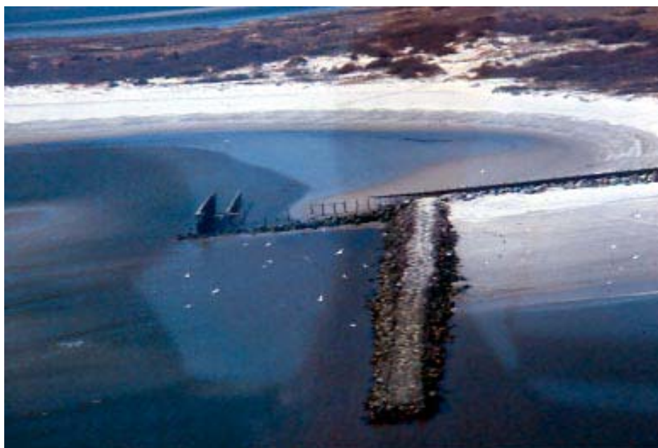
Figure 54. Aerial photograph showing advanced terminal groin effects, Stone Harbor Point, NJ in early March 1984 (before the late March storm). Erosion caused by terminal rock groin in foreground has caused erosion in an arcing pattern behind the structure actually flanking it. Subsequently, the entire Point eroded away (dune field and spit visible in background). (Photograph by Dr. Susan D. Halsey)
