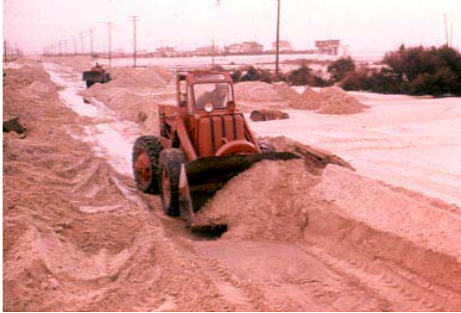
Figure 20. Front end loaders removing extensive storm washover from Long Beach Boulevard, New Jersey, in the Loveladies section of Long Beach Island. At some locations, washover was over four feet deep (Photo courtesy of Lawrence Wagner).
