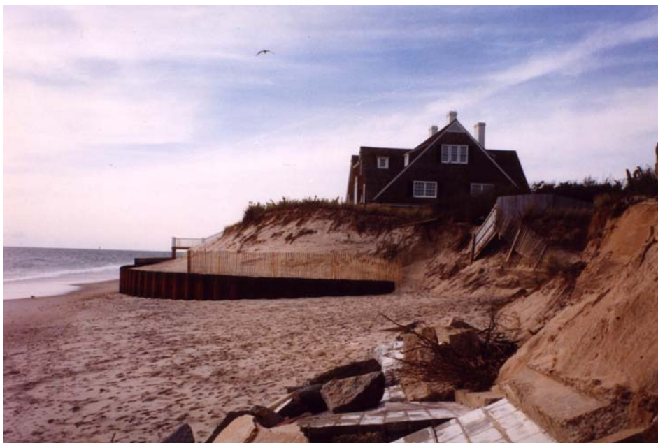
Figure 56. A sheet metal bulkhead installed to prevent the undermining of a dune and adjacent home. Bulkheads exposed to direct wave attack can result in the loss of sediments fronting the structure (Photograph by Dr. Michael S. Bruno).
