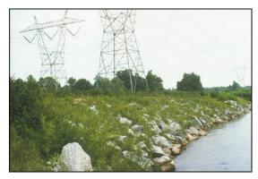
Figure 8: Typical Joint Planted Revetment
