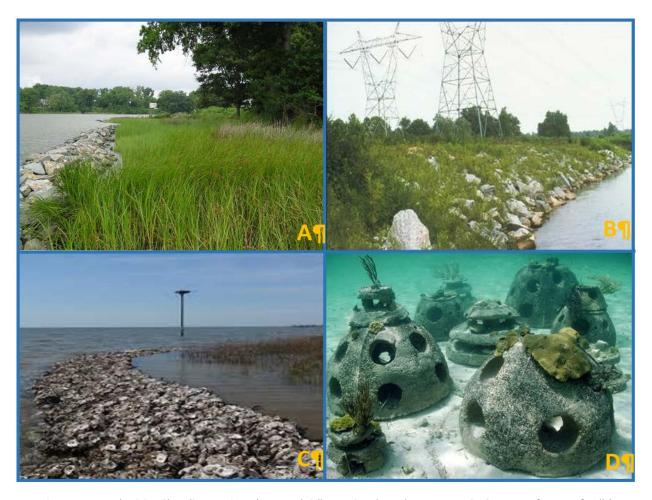
Figure 1: Example Living Shorelines Projects (A - Marsh Sill, B - Joint Planted Revetment, C - Oyster Reef, D - Reef Balls)
