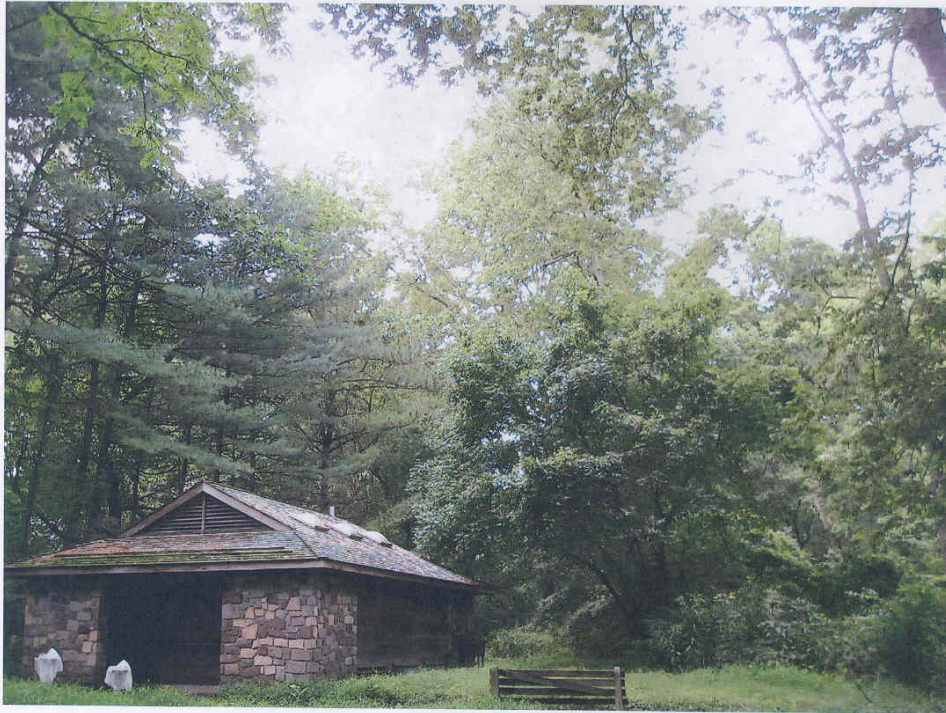
Photo No 3: One of two bath houses to be removed within the campground area.
