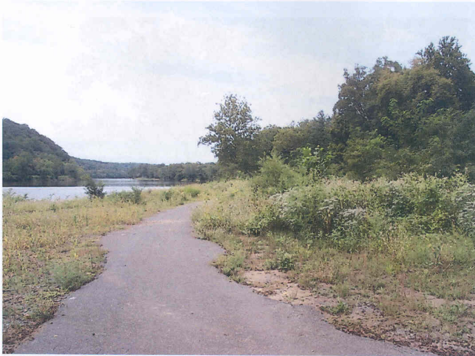
Photo 9: Proposed recreational pathway corridor along the existing roadway along the Delaware River.
