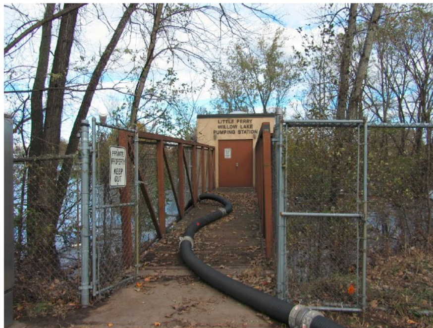
Figure 18. Willow Lake Pumping Station
