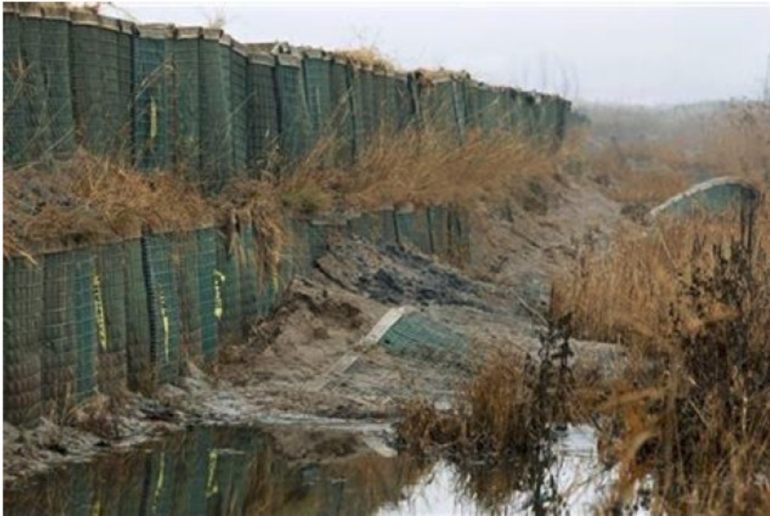
Figure 17. Sandy-damaged berm and contiguous ditch (Carlstadt, Meadowlands)
