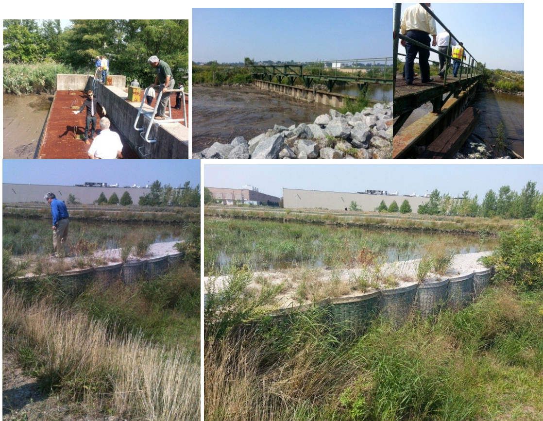
Figure 20. FMERC Team surveying flood protection structures (tide gates and berms at various Meadowlands locations)
