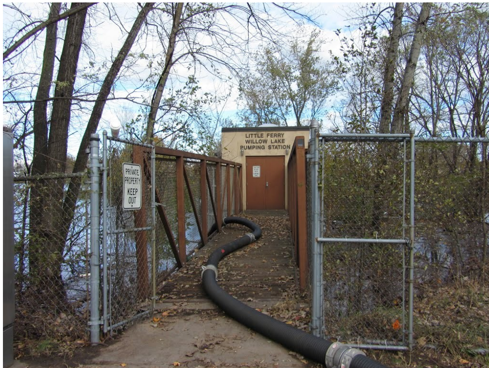
Figure 10 Willow Lake Pump Station
