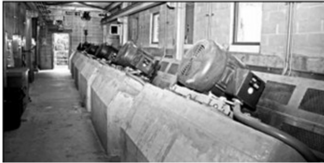
Figure 11 Teterboro Pump Station (Gazette, 2008)
