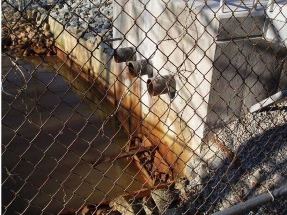
Figure 3 Outfalls of DePeyster Creek Pump Station (NJMC 2006)
