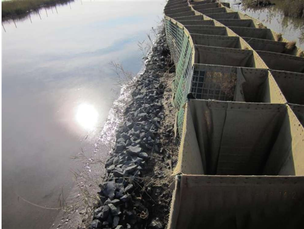
Figure 26 Failed Berm cleared of stone due to Sandy (NorthJersey.Com Meghan Grant)
