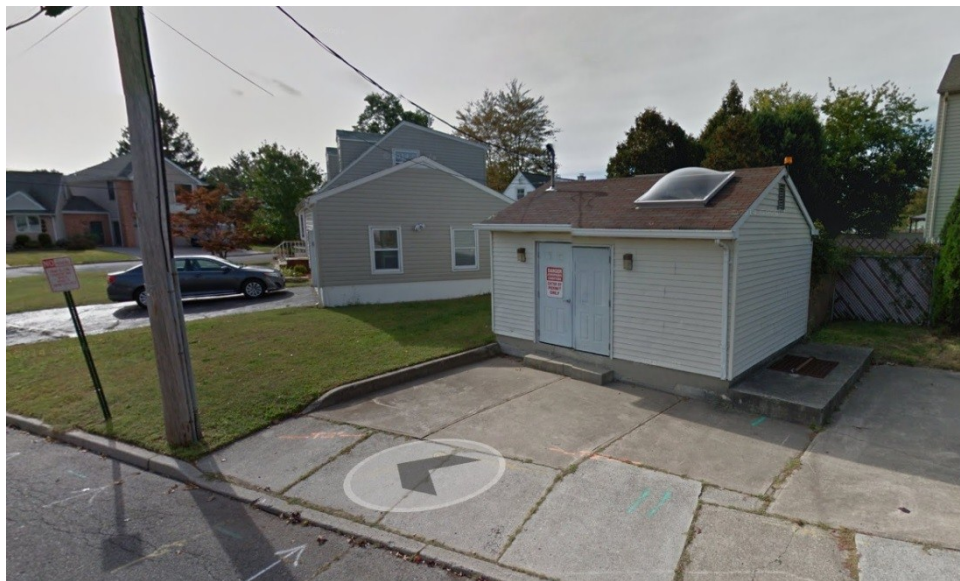
Figure 12: Lincoln Place stormwater pump station (courtesy Google maps)
