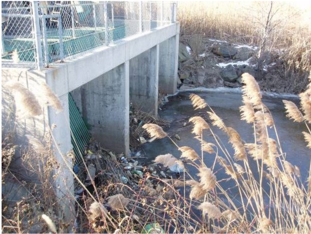
Figure 8 View of trash racks at in-take structure (NJMC 2006)
