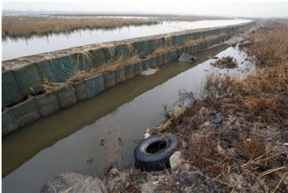
Figure 21 Typical View of the Berm with two Layers (AP Photo/Mel Evans)
