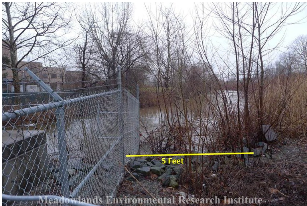
Figure 6 Downstream of the DePeyster Pump Station (NJMC 2012)
