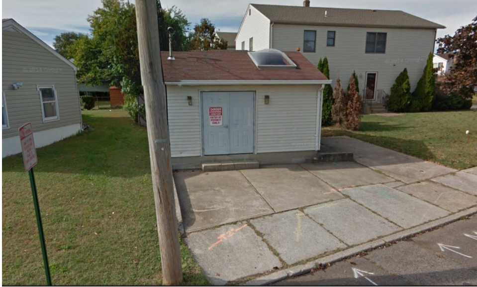
Figure 13: Lincoln Place stormwater pump station (courtesy Google maps)
