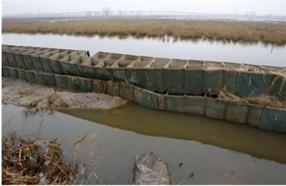
Figure 22 View of the failed two layer Berm due to Sandy (AP Photo/Mel Evans)
