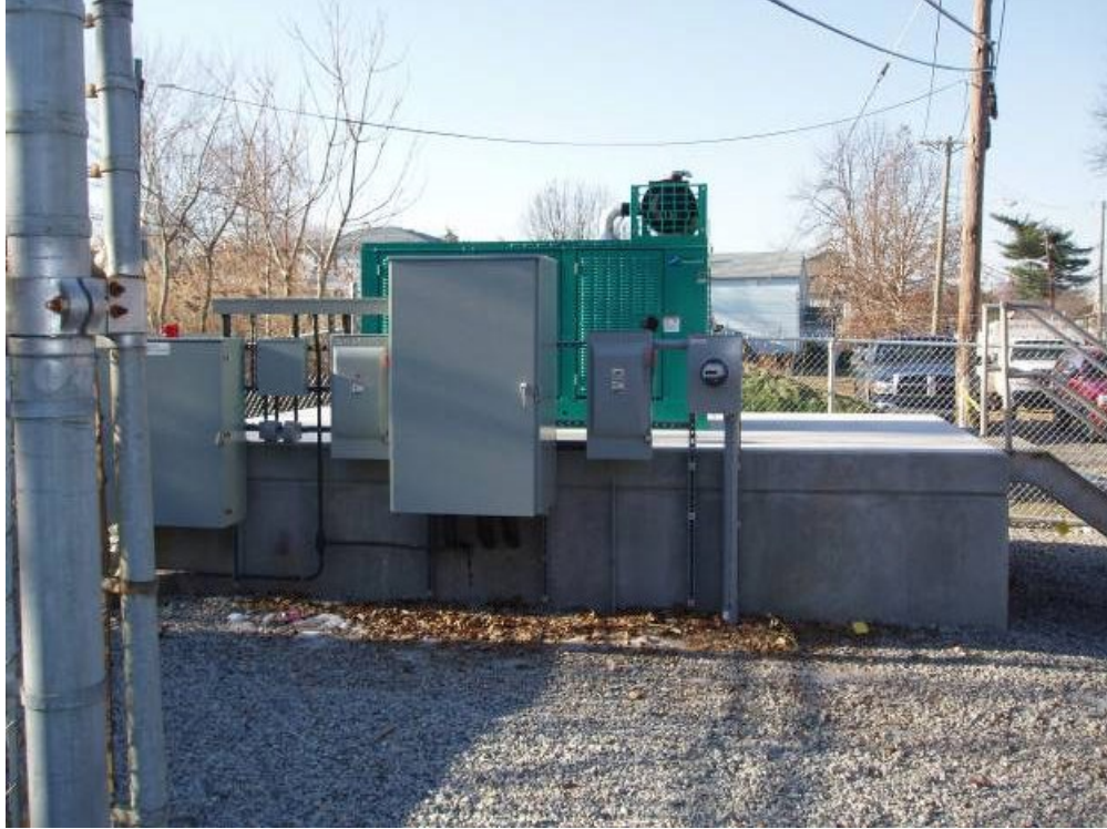
Figure 5 DePeyster Pump Station (NJMC 2006)
