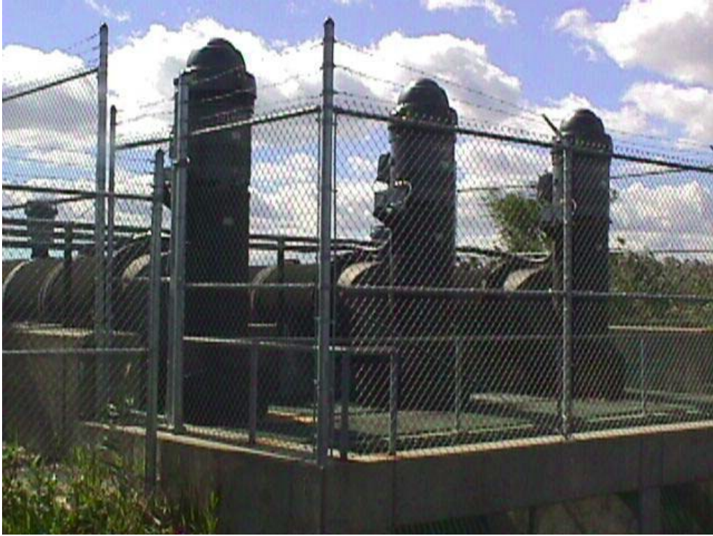
Figure 7 Losen Slote Creek Pump Station (FEMA 1999)
