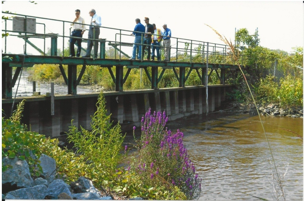
Figure 17 Looking Upstream of West Riser Tide Gate.
