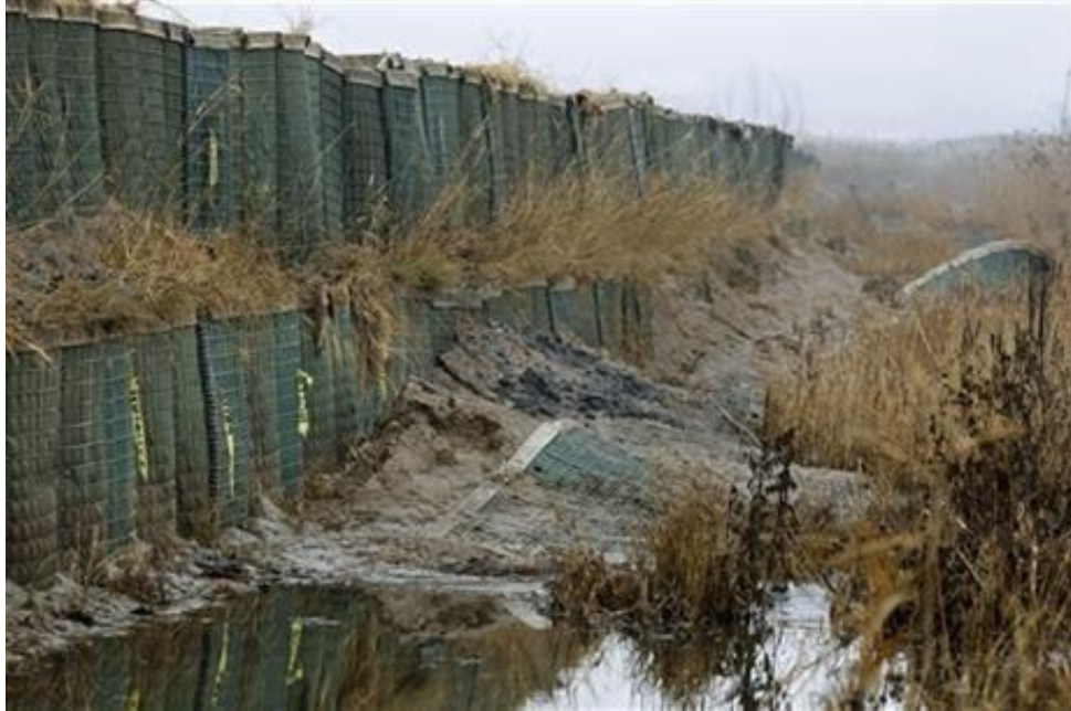
Figure 24 Close-up View of the Berm with a failed section due to Sandy (AP Photo/Mel Evans)
