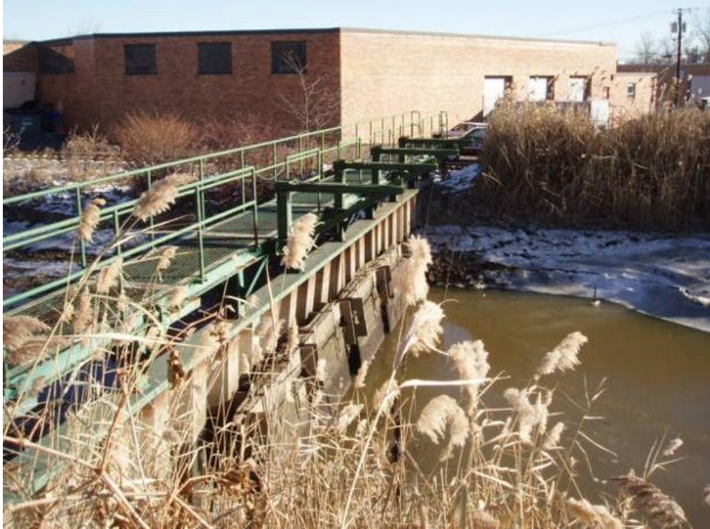
Figure 16 Looking Upstream of West Riser Tide Gate (NJMC 2006).
