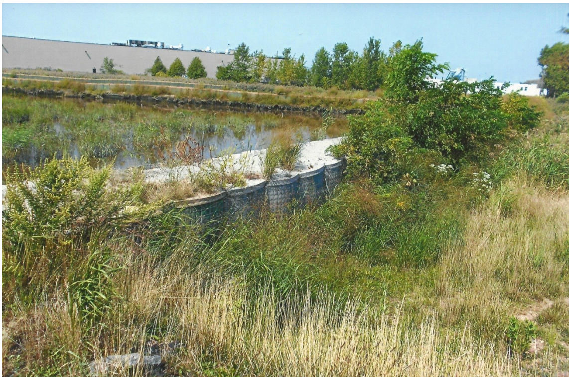
Figure 28 A section of intact Berm after Sandy
