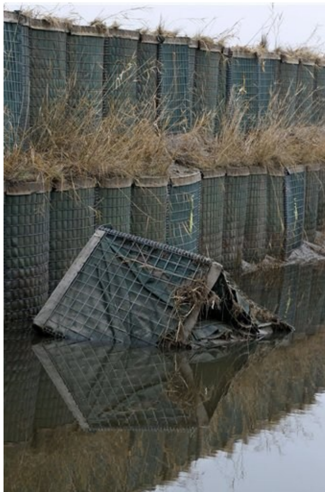
Figure 23 Close-up View of the Berm with a failed section due to Sandy (AP Photo/Mel Evans)
