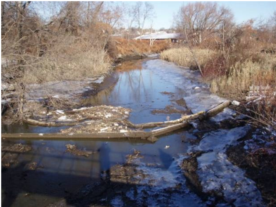
Figure 15 Upstream of West Riser Tide Gate (NJMC 2006).
