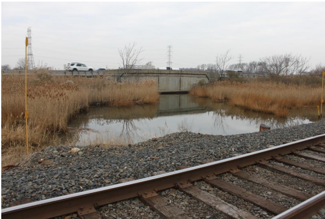
Figure 31-Marshes Creek Crossing Under NJ Turnpike
