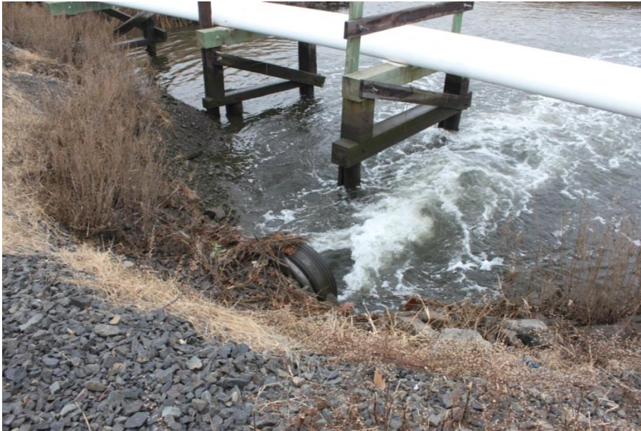
Figure 33-Marshes Creek Downstream of Railway Line
