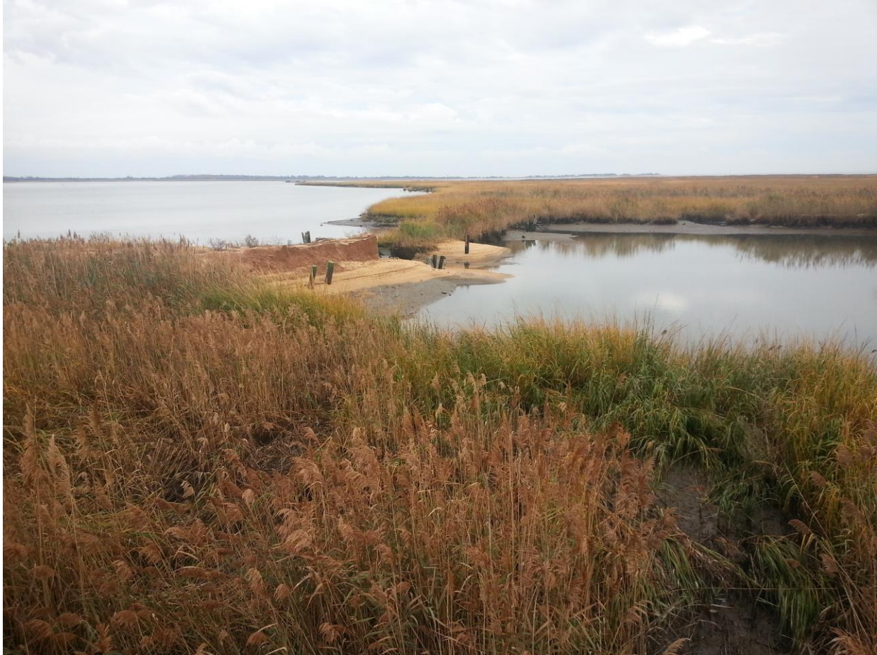
Figure 33-Failure of Peak of the Moon dike within Bivalve community, Port Norris, NJ
