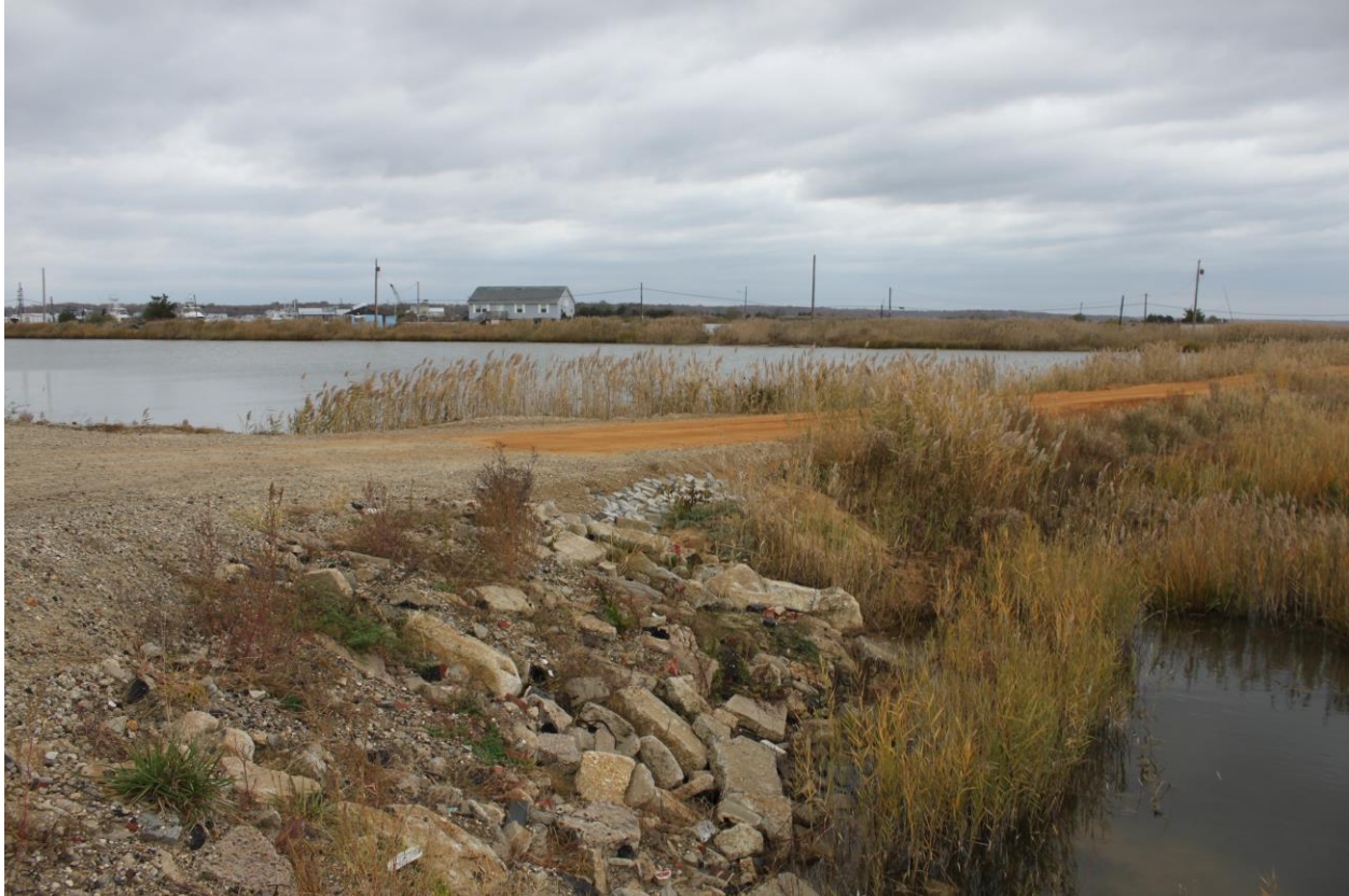
Figure 49- Heislerville Dike breached and subsequently repaired in Maurice River Township, NJ
