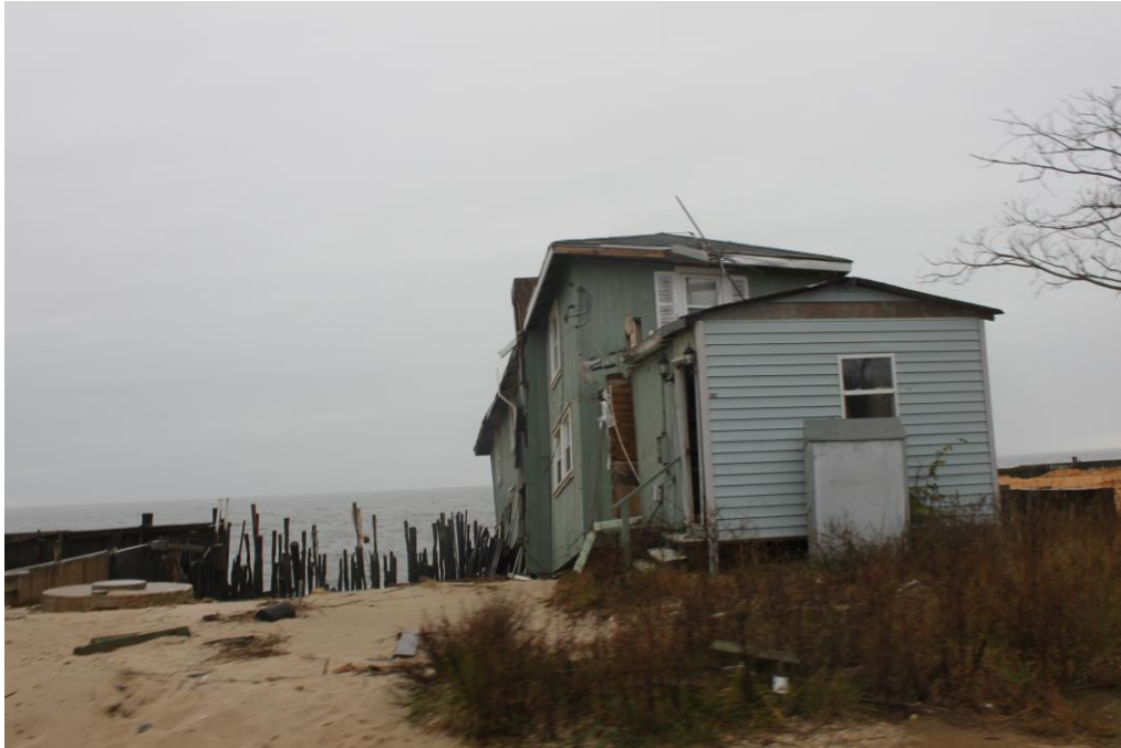
Figure 39-Damaged house in Fortescue, Downe Township, NJ
