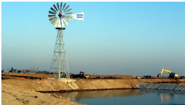
Figure 29 - The 6m dia. windmill tower (Ironmanwindmill, 2014)
