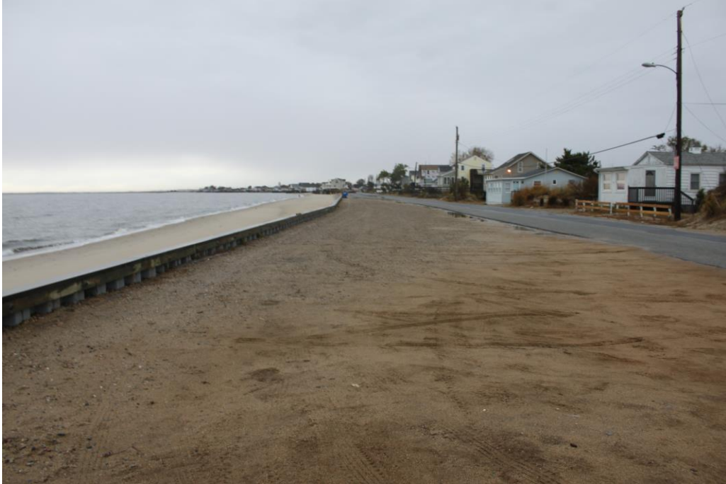
Figure 38-Jersey Ave road severely damaged but largely repaired with vinyl sheet pile in Fortescue, Downe Township, NJ
