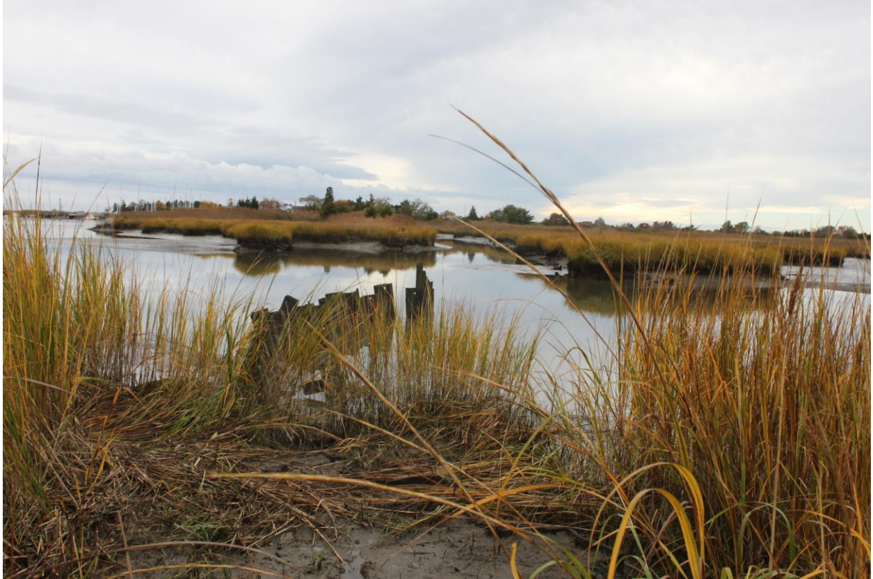
Figure 44-Failed Pile Mount Dike looking across from Greenwich Boat Works Marina in Greenwich, NJ
