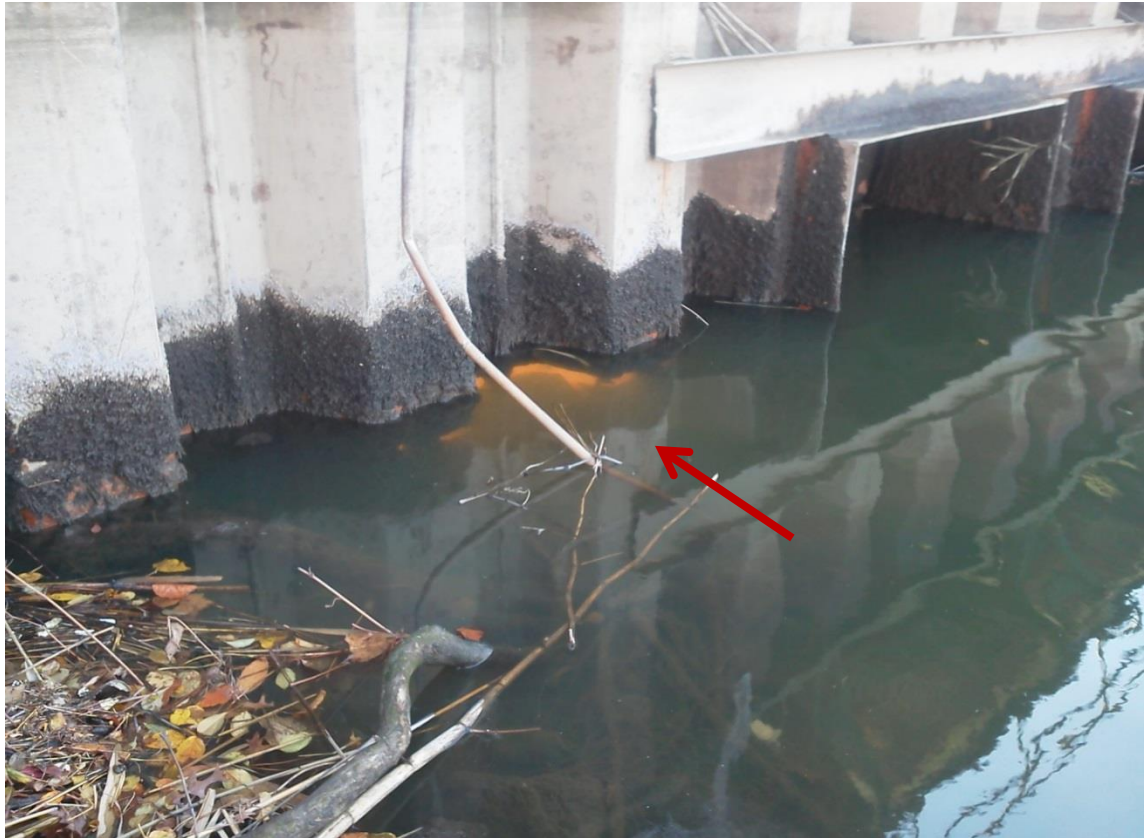
Figure 15: A hole in the West Riser Tide Gate below the waterline is shown.
