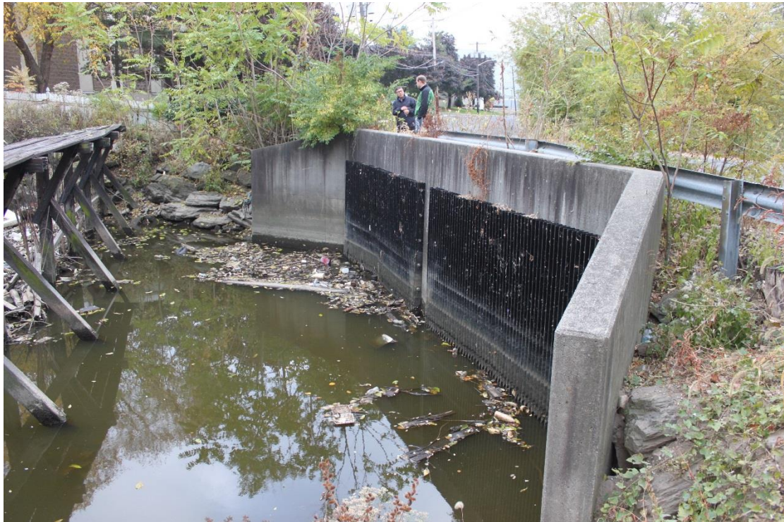
Figure 10: View of trash racks at intake structure, East Riser tide gate
