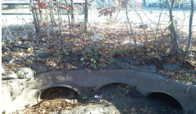
Figure 13: Headwall in Moonachie with three drainage pipes of unknown origin
