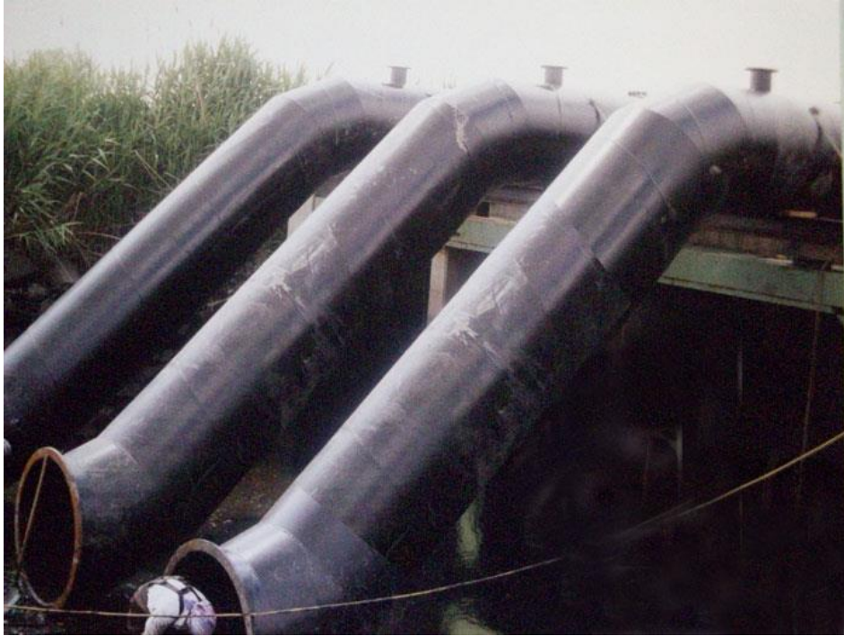
Figure 7: Losen Slote Tide Gate is equipped with high volume pumps, and a diesel generator backup power supply
