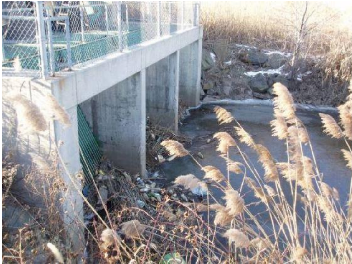
Figure 8: View of trash racks at intake structure, Losen Slote tide gate
