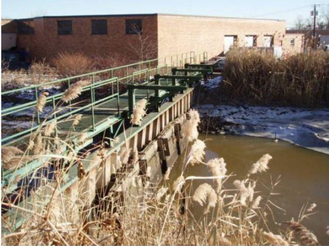
Figure 9: Four timber tide gates, West riser tide gate.
