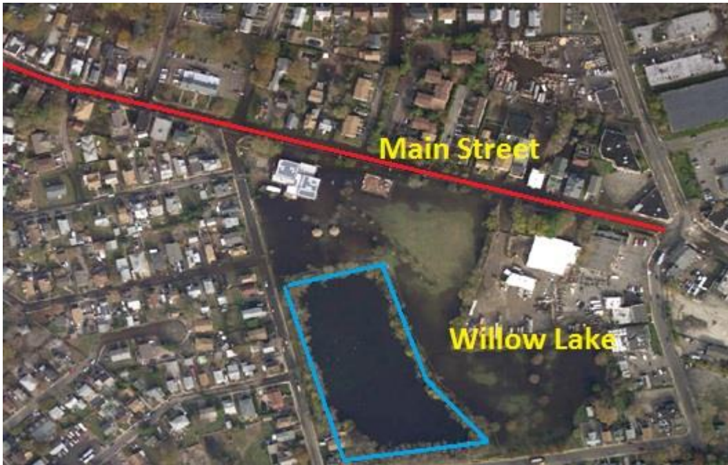
Figure 4: Main St., Little Ferry. This area remained flooded for 5 days following Sandy because Main Street and Willow Lake pump station were without power and there is no gravity drainage. (Photo from NOAA flyover November 1, 2012.)
