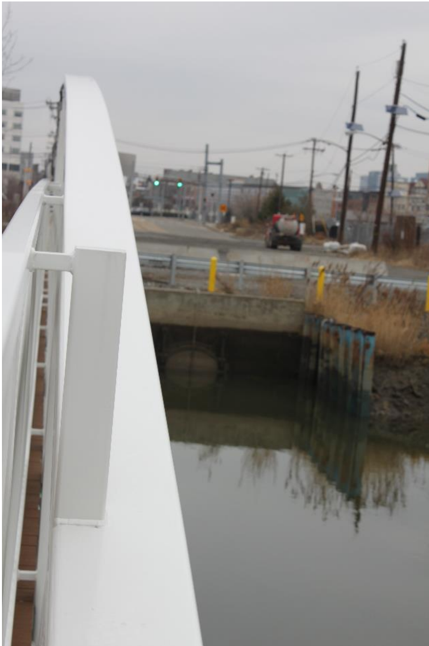
Figure 16: Flap Gate at Morris Marina, Jersey City, NJ
