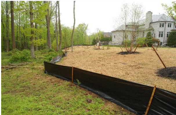
Soil Stabilization utilizing seed, straw mulch, and silt
