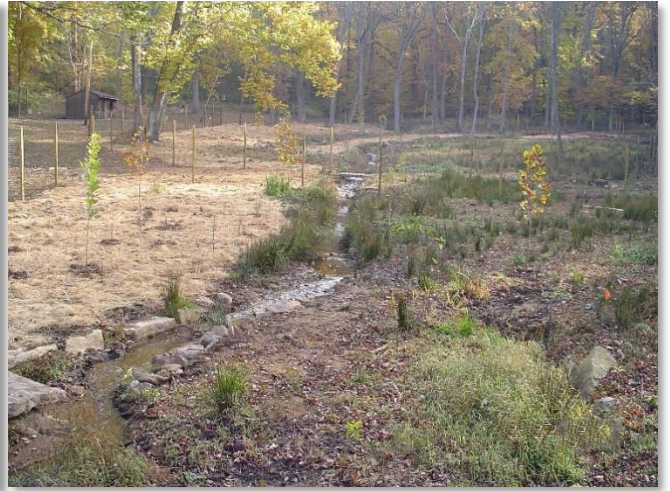
Restoration reestablished a meandering channel and recreated riffle and pool habitat for trout. Plantings included trees that will in time provide much needed shade to help keep water temperatures cooler.
