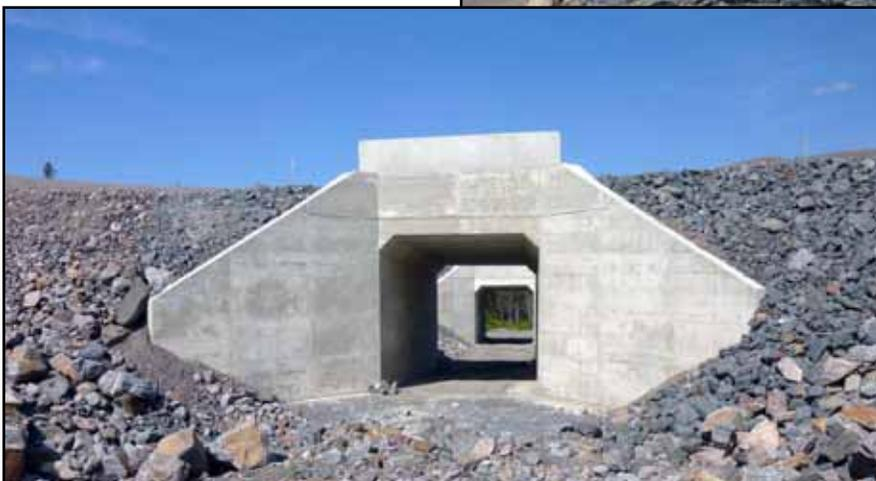
*Wildlife crossing structures under construction in Ontario. The highway was realigned/twinned and this overpass (above) is the first of its kind in Canada east of the Rockies, 2011. The 5m X 5m underpass (left) is intended to be a joint wildlife/forest access structure. Photos by Ontario Ministry of Natural Resources.*
