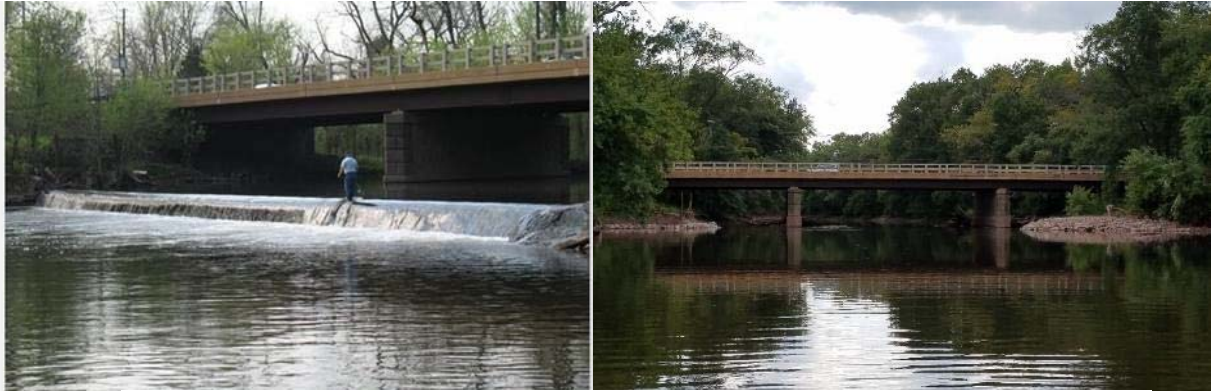
Weston Mill Dam (photo by John Jengo) (left) and after removal of dam (right).
