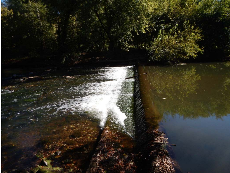
Blackwells Mills Dam, located approximately 4.5 miles upstream of former Weston Causeway Dam. Low flows conditions during fall of 2017
