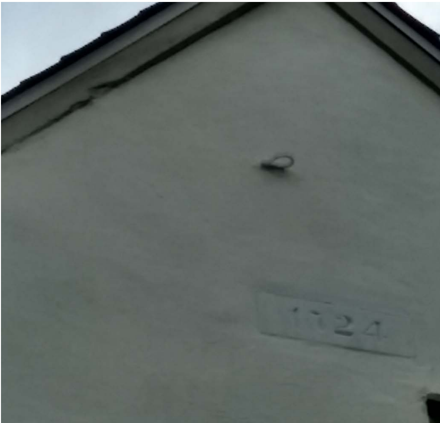
Figure 39 The datestone was carefully carved to send a message; was it what the stucco is covering up?
