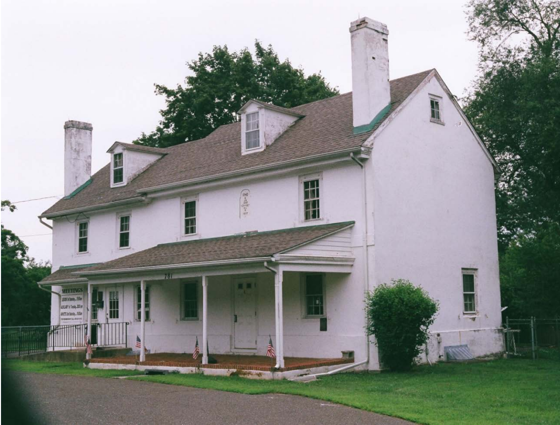
Figure 34 A stuccoed house from the 1740s, likely to be hiding patterned brickwork.
