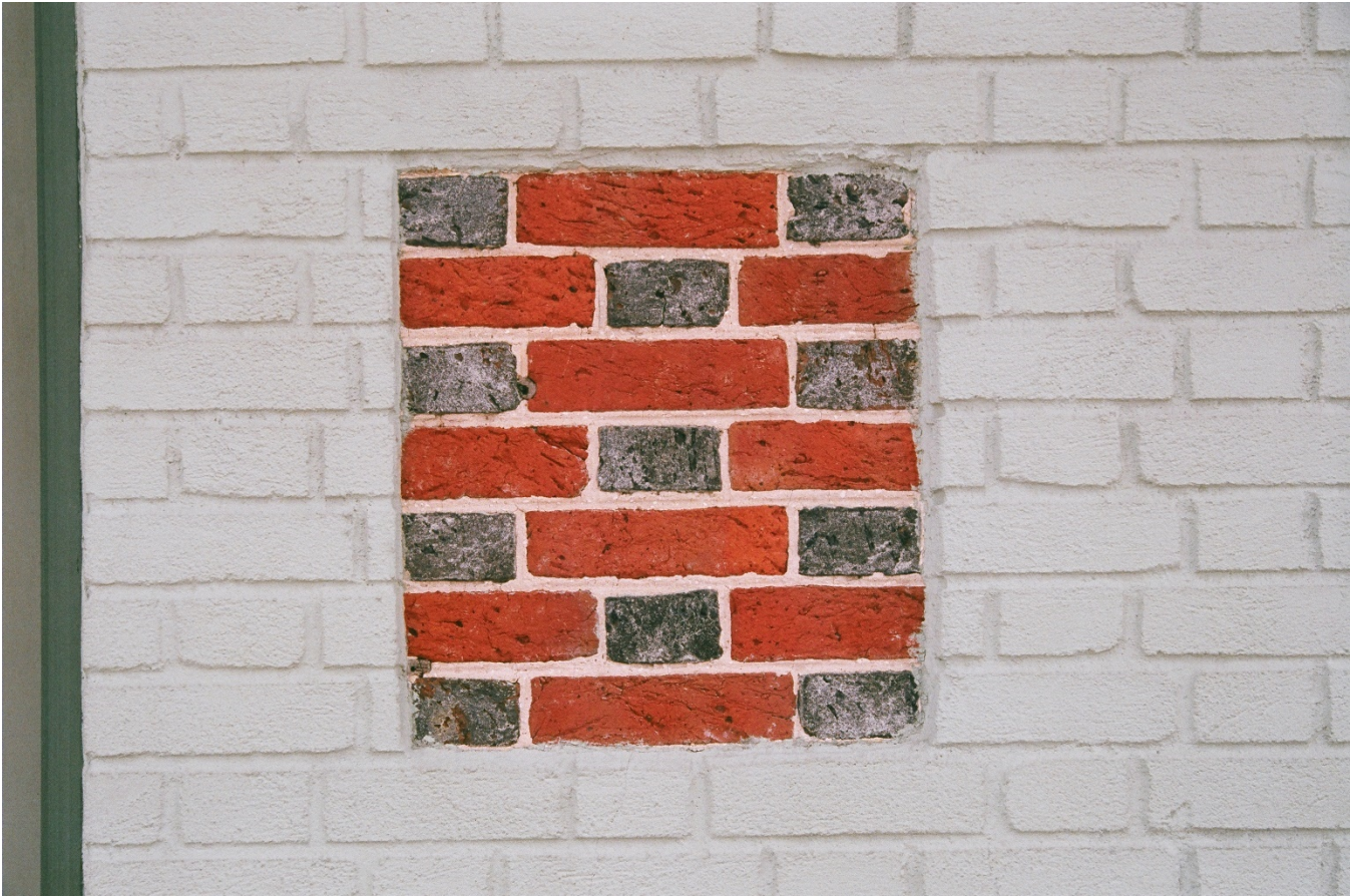
Figure 36 This building has Flemish checker lurking under brickface.
