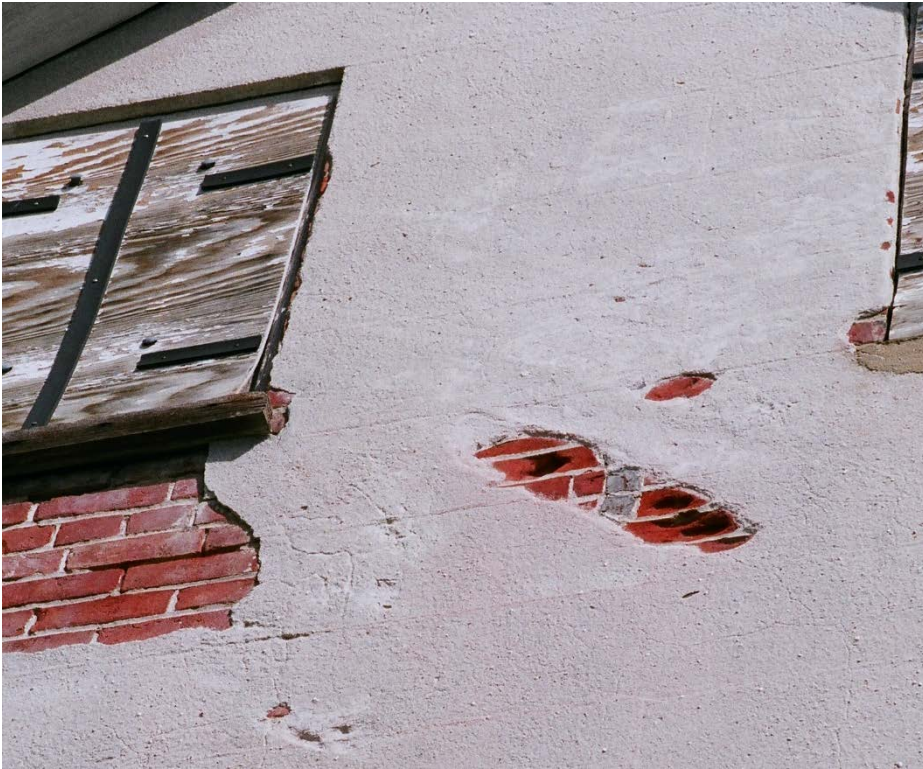
Figure 38 Stucco spalling, slowly revealing a date.
