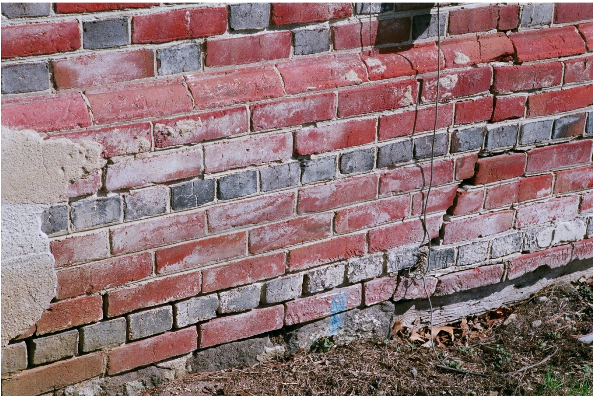
Figure 22 Banding, below the water table.
