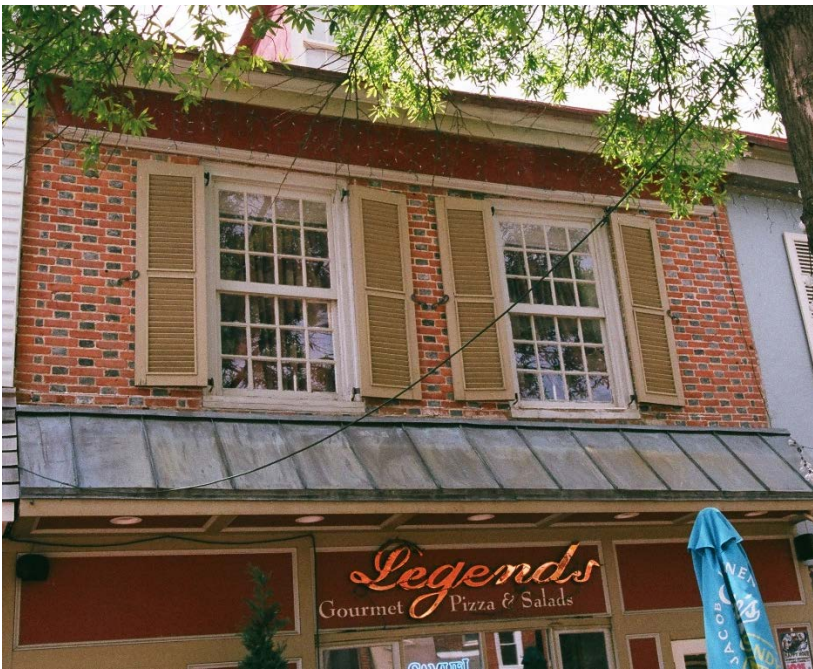
Figure 2 Some patterned brickwork townhouses abutted their neighbors.
