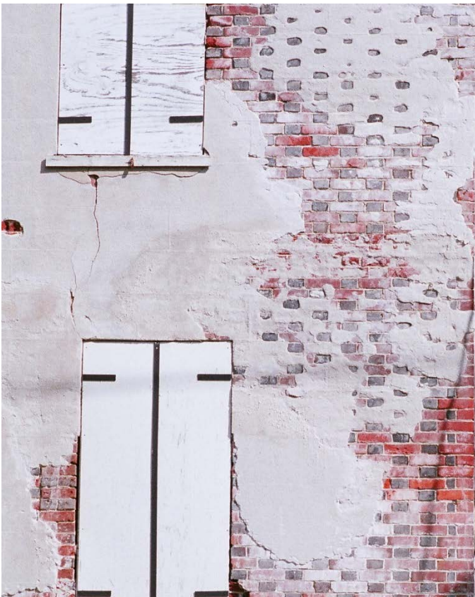
Figure 37 Stucco eroding away...
