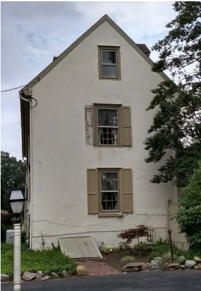
Figure 32 This part of the Abbott house was built in 1704; what patterned work is the stucco hiding?
