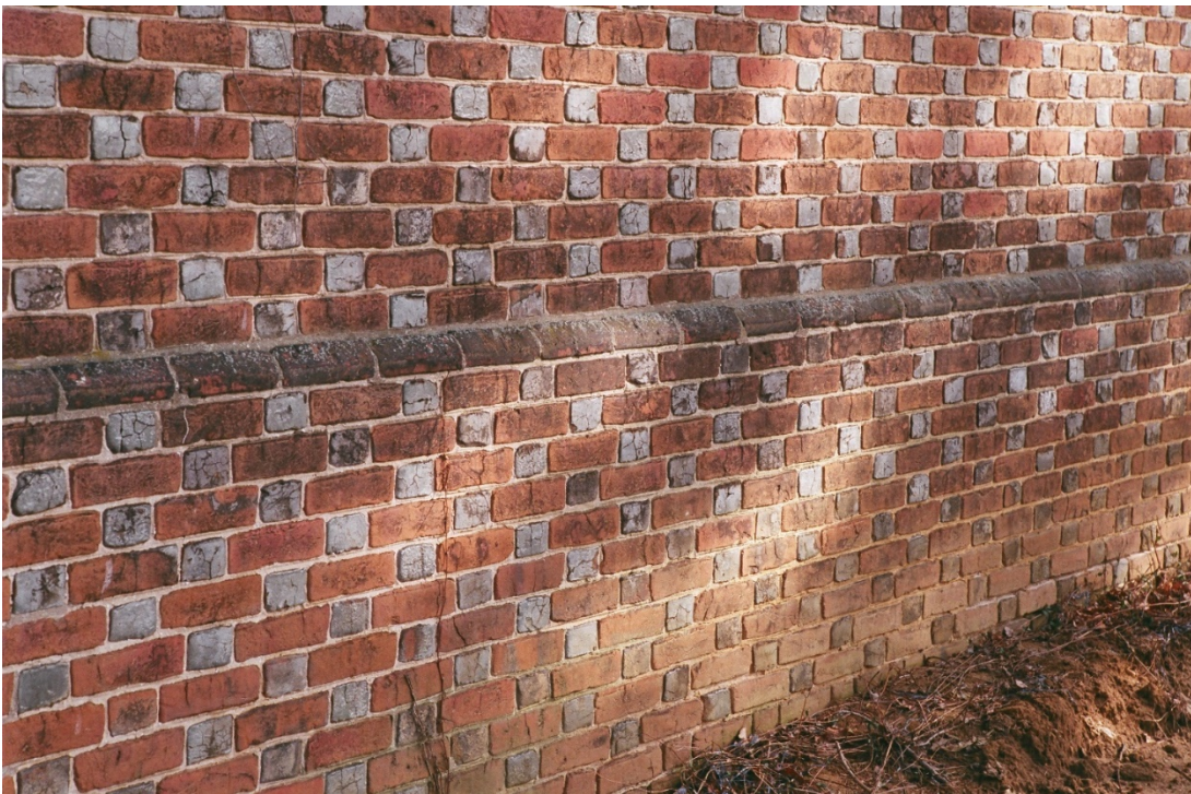
Figure 17 Flemish checker, above and below the water table, an unusual practice.
