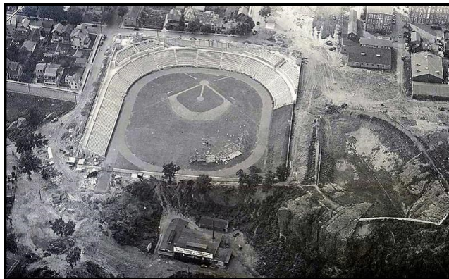
Hinchliffe Stadium 1932 | Photo: Paterson Museum
