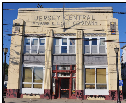
Jersey Central Power & Light Keyport
