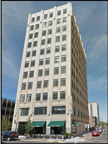
Electric Company Building Asbury Park
