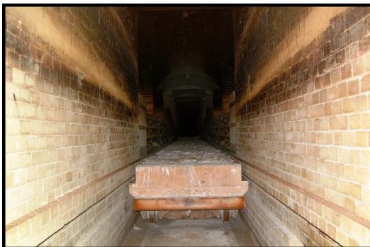
American Standard Line Kilns, 2003 Credit: NJ SHPO
