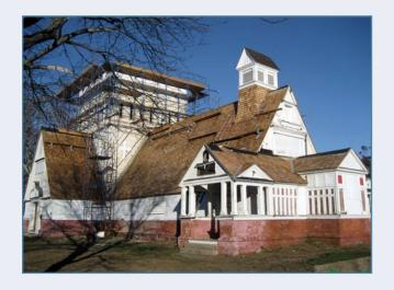
In 1955, the building opened as the Long Branch Historical Museum and remained open until 1999, when structural concerns forced the building's closure for safety reasons. The building's structural instability is associated with the construction of the massive tower in 1895.
