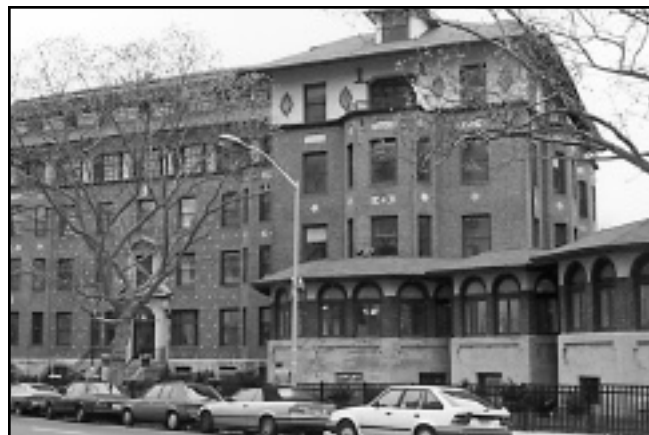
FAIRMOUNT APARTMENTS, JERSEY CITY
