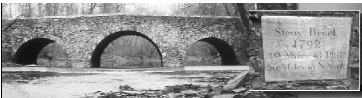
STONY BROOK BRIDGE, KING'S HIGHWAY HISTORIC DISTRICT
