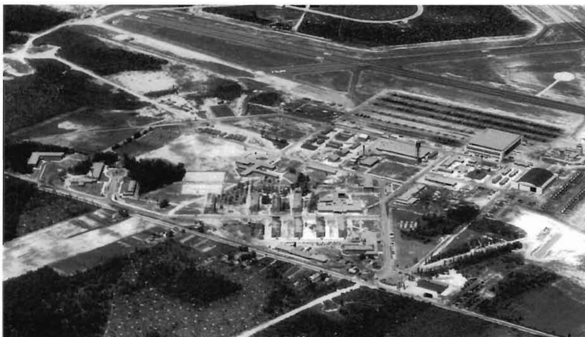
Figure 6 (above): 1945 aerial view of Naval Air Station Wildwood, looking northwest. Hangar No. 2 is seen at the far right. [National Archives, as found in Shettle, Naval Air Stations of WWII , Vol. I, p. 226]
