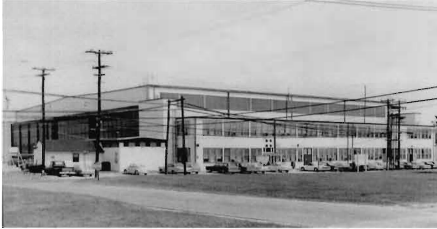
Figure 10 (left): Hangar at Naval Air Station Atlantic City, ca. 1960. This structure shows the similarity in hangar design with those at USNASW.
