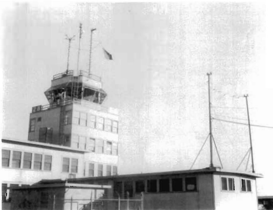
Figure 2: close-up photograph of the control tower with the sewage pump house shown in the foreground. Ca. 1946? View northeast.
