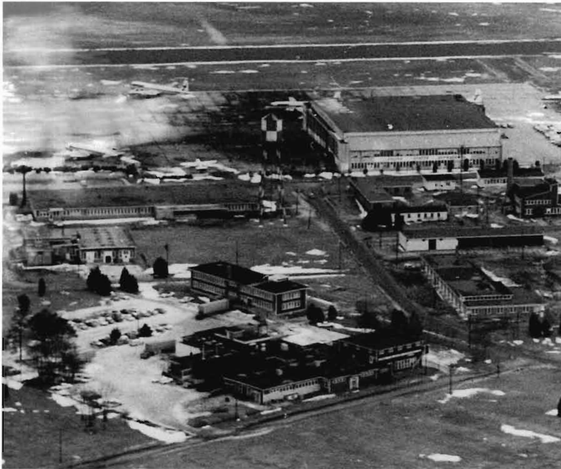
Figure 13: ca. 1960 photograph, looking north. Hangar No. 1 is seen in the upper right and the mess hall, with a second story added to its southeast corner is at the bottom center of the photograph. [courtesy of Naval Air Station Wildwood Aviation Museum]
