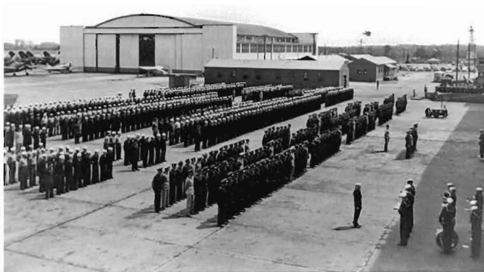
Figure 4: Hangar No. 2 as it appeared in 1945, view southeast. Note the wood frame buildings, mostly “ready rooms,” to the right of the hangar; only the hangar is extant today.
