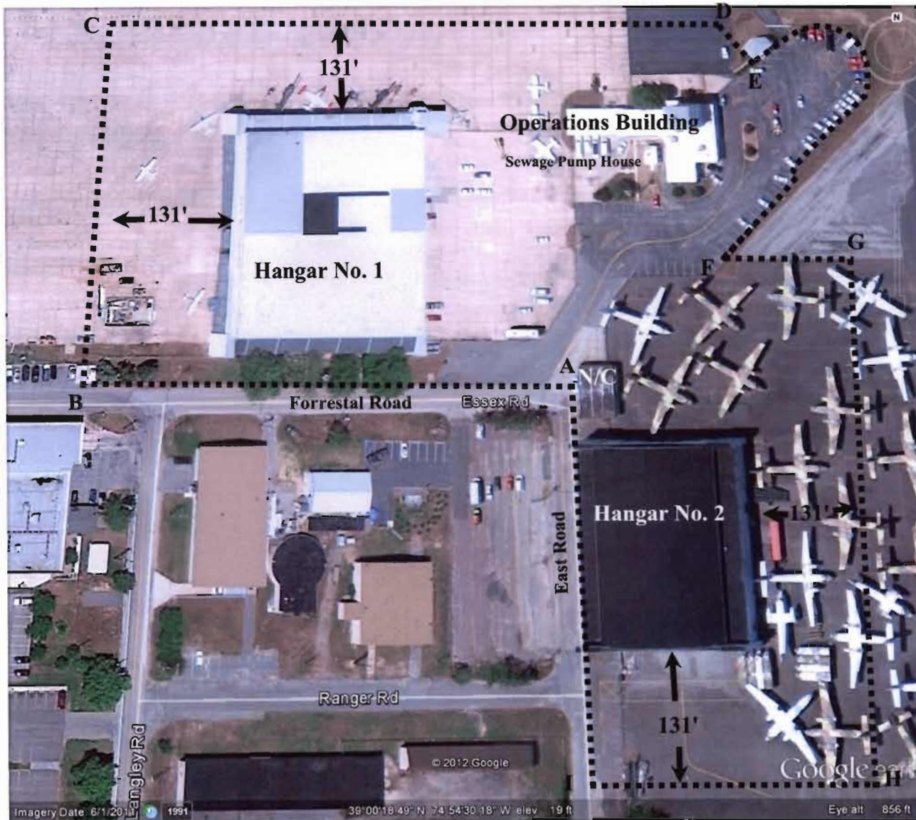
Naval Air Station Wildwood Historic District Aerial Photograph Annotated for Boundary Points
