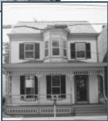
Alexander Coryell House, 39 N. Main St., Lambertville, New Jersey before and after successful rehabilitation .
