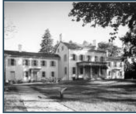
A view of the newly restored exterior of Historic Morven
