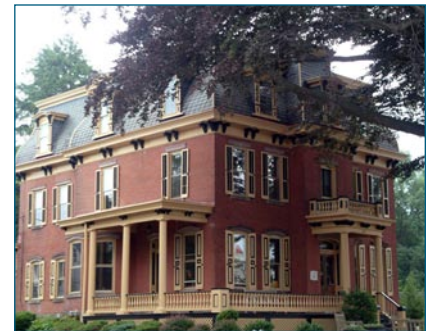
The John Hopkins House at 10 W. Main Street in Moorestown has been fully rehabilitated to serve as a real estate office.
