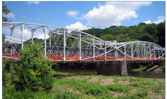
Elm Street Lenticular Truss Bridge
