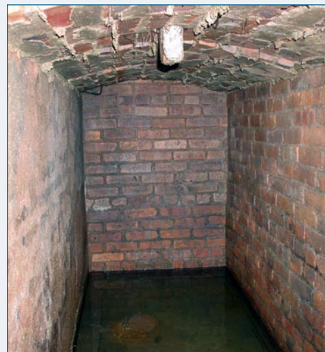
Antechamber adjoining the inner chamber of Edison's Menlo Park Patent Vault
