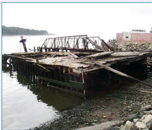
3/4 view of the starboard side of the MARICOPA taken from the bow
