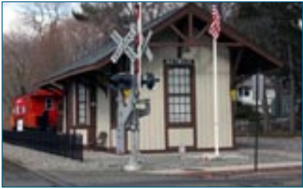
Maywood Train Station Restoration
