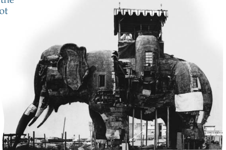
Lucy in her seriously deteriorated condition c. 1970.
