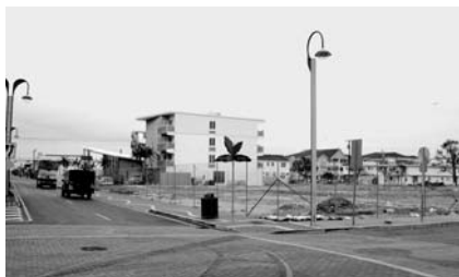
Site of Rio Motel after demolition.
