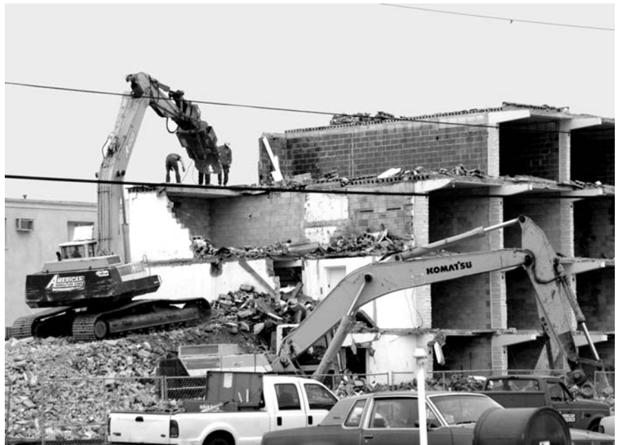
Demolition in progress at the Palm Beach.
