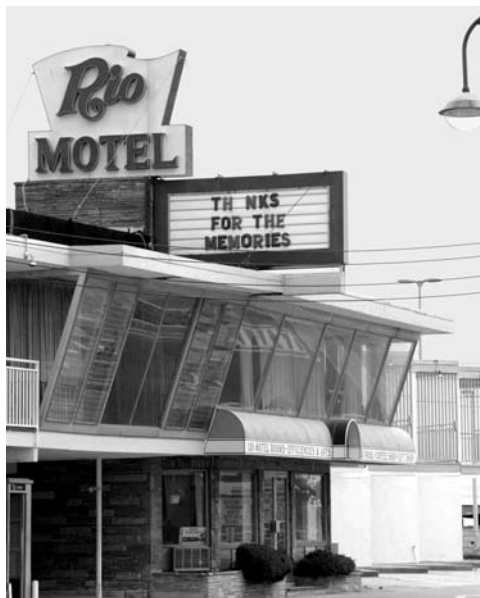
Rio Motel, prior to demolition.
