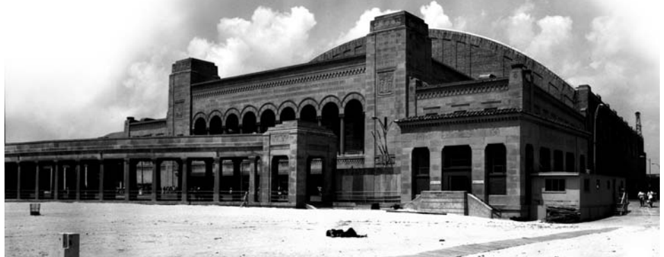
Beach front view of the Atlantic City Convention Hall, 1982
