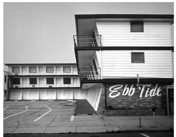
Angled walls of the Ebb Tide Motel, Wildwood Crest. The first motel built on the island. Now demolished. Photo courtesy of HABS
