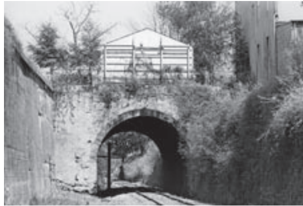
Railroad Underpass, Farnsworth Avenue, Bordentown, Burlington County
