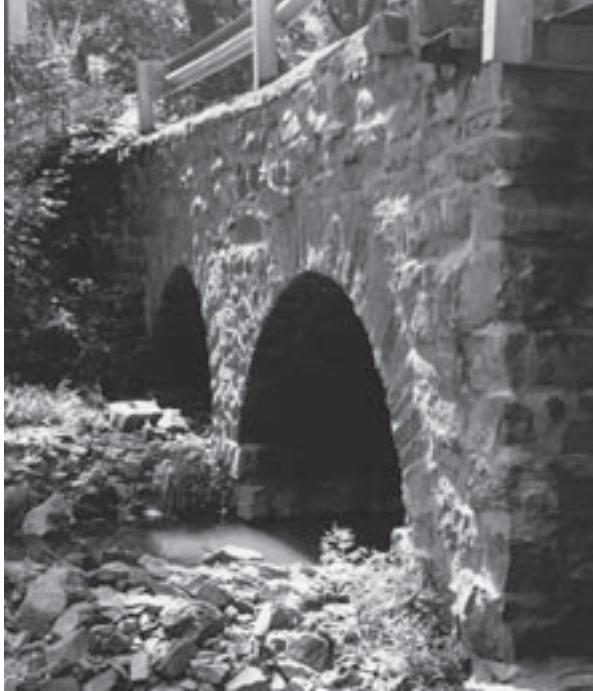
Rock Brook Bridge, Montgomery Township, Somerset County
