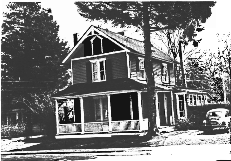
1308-12 612 Union Ave.; Block 24, Lot 2; Point Pleasant Quad; Neg File No. 1-23 c. 1870's vernacular Victorian frame residence. 2 story, 1 over 2 bay rectangular plan with side and rear ell. Gable roof with ridge and side wall chimneys and vergeboard in peak. Clapboard siding. Pointed head window in gable, paired 1/1 sash windows on front facade, 2/2 sash on side wall windows. Doorway is in side ell section and has a small transom light. Two sided porch is supported by smooth classical columns. Brick foundation. Modern stovepipe in rear ell. Owned by C.E. Pearce in 1889. The building has been well preserved.
