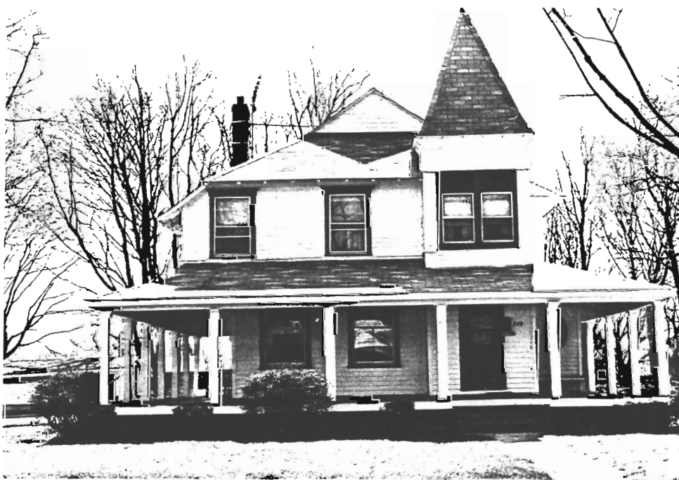
1308-2 329 Fisk Ave.: Block 47, Lot 4; Point Pleasant Quad; Neg. File # 1-27,28,29. Early 20th century frame residence with Free Classic elements. 2 story, 3 bay asymmetrical fenestration with irregular plan. Hipped gable roof with steep pyramidal tower roof. Clapboard siding; with cross-hatched shingles below bracketed tower eaves. 1/1 sash windows; three sided porch supported by squared columns. Foundation is not visible
