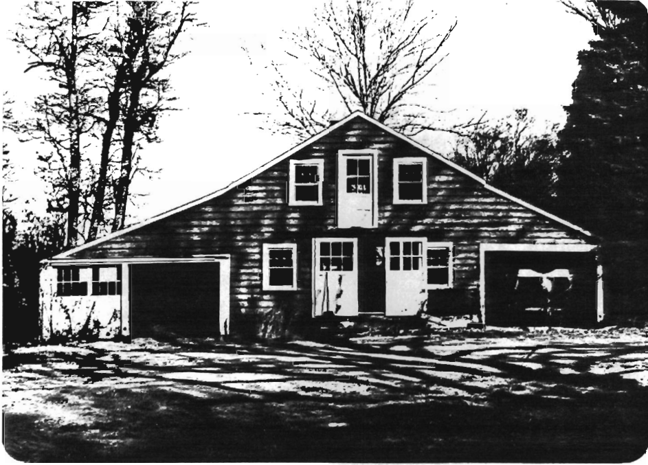
Wagon shed, view to NE.
