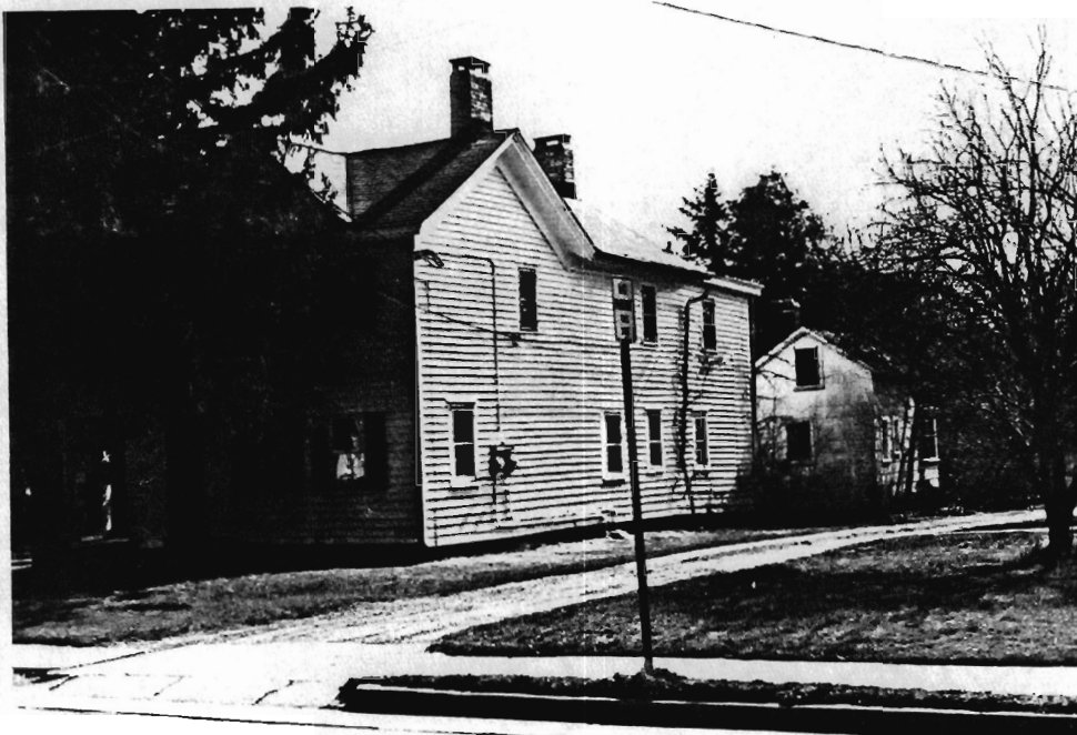
1327-1-6 27 Main St.; Block 27, Lot 19; Asbury Park Quad; Block 27, Lot 19. c. 1850's-1860 frame vernacular Victorian residence. 2½ story, 3 bay form with rear 2½ story wing. Intersecting gable roof with overhanging eaves. Internal end wall chimneys on main block and rear wing. Clapboard siding. 6/6 sash windows in simple frames. Doorway is in a simple frame. Brick foundation. Owned by A. Longstreet in 1873 and 1878. A small 1 story frame shop is behind the house.
