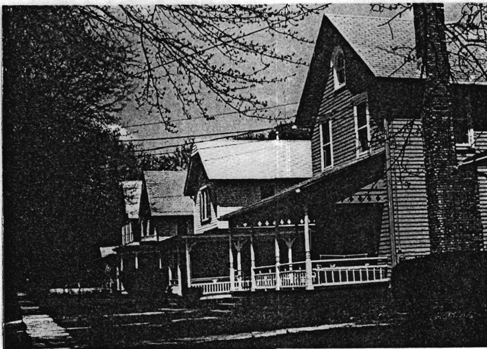
Streetscape: N. side Morris Ave., view to NW. (outside district).
