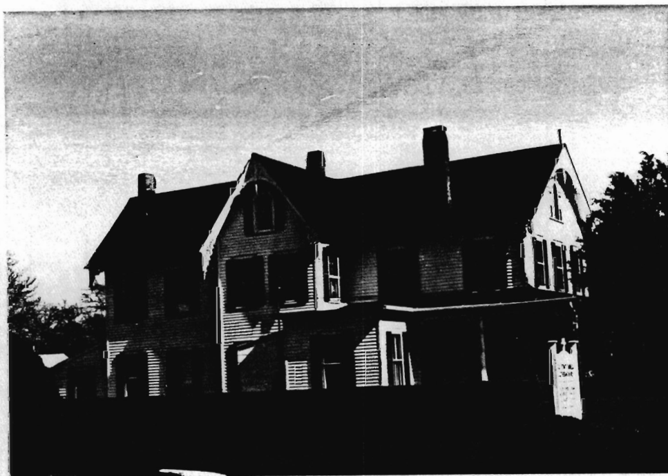
1327-1-7 Dr. A.A. Higgins House 38 Main St.; Block 35, Lot 4; Asbury Park Quad; Neg. File No. 1-2,3. Between 1873 and 1878 frame vernacular Victorian residence. 2½ story, 3 bay by 6 bay T-plan with 1 story additions. Intersecting gable roof with 2 ridge chimneys and 1 side wall chimney. Vergeboard is in gable peak and pendants hang from corners of roof. Clapboard siding. 2/2 sash windows. A Palladian window is in the front gable peak. Double doorway has a 2 light transom and shouldered architrave. Two-sided porch is supported by squared posts with millwork brackets. Owned by Dr. A.A. Higgins in 1878 and 1880. He owned the property in 1873.
