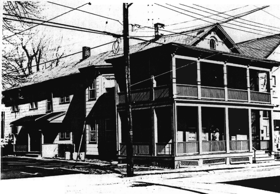
1327-1-9 68 Main St.; Block 35, Lot 11; Point Pleasant Quad; Neg. File No. 1-8,9. c. 1870's frame residence with Italianate elements. 2½ story, 2 over 3 bay by 7 bay form, the rear section being a later addition. Gable roof with bracketed, overhanging eaves. Asbestos shingle siding. 2/2 sash windows with projecting lintels. Two front doorways/ Two story porch is supported by squared posts and has bracketed eaves. Brick foundation. The building is currently an apartment house. The building appears to have been owned by P. Curtis in 1873, 1878 and 1889, though the historic maps are somewhat ambiguous in this area.
