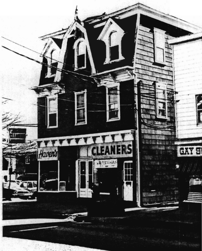
1327-1-10 81 Main St.; Block 27, Lot 7; Point Pleasant Quad; Neg. File No. 1-7. Between 1878 and 1889 frame Second Empire commercial building. 3 story, 3 bay rectangular form. Mansard/flat roof with central gambrel section on front facade. Slat roofing on mansard slope. Round headed windows on third floor. 2/2 rectangular sash on second floor. Large, single light storefront windows on first floor. Bracketed cornice is above storefront. Simulated brick siding on front facade, asbestos shingle over clapboard on side walls. Brick foundation. Owned by Friedlander in 1889.
