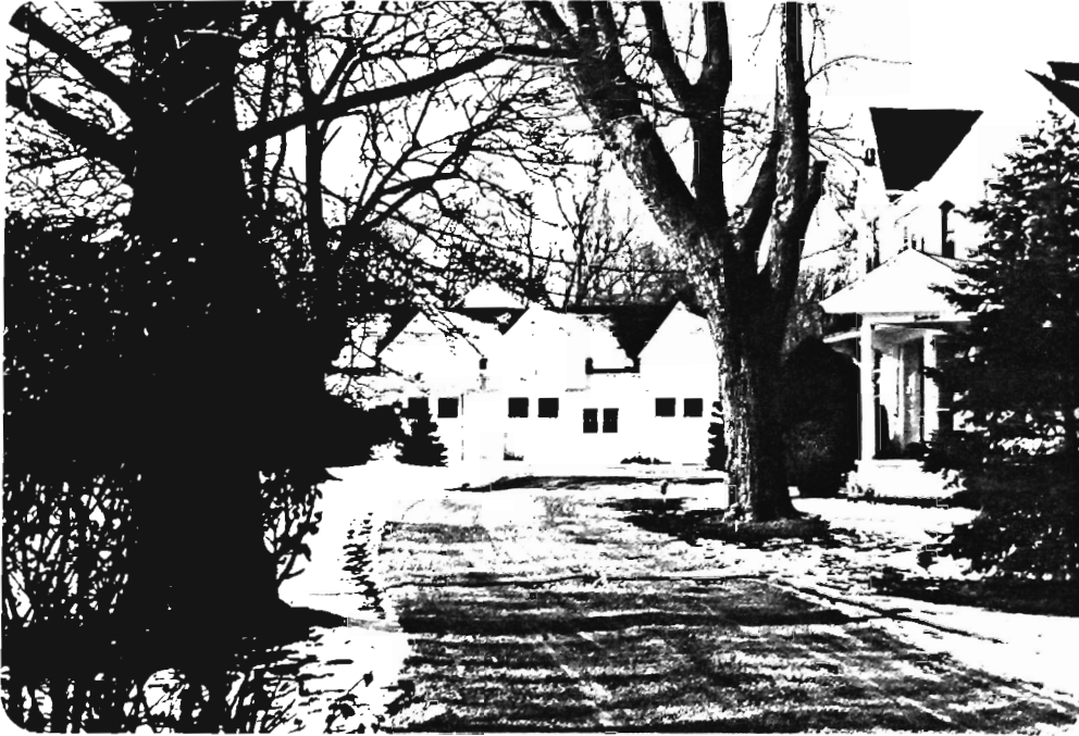
Carriage House, view to W.
