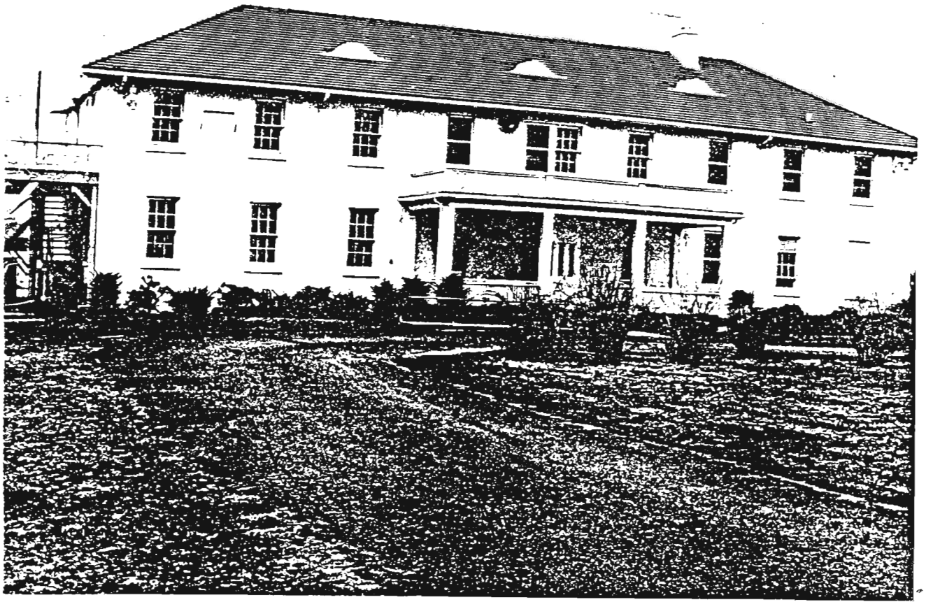
BUILDING A - East facade
