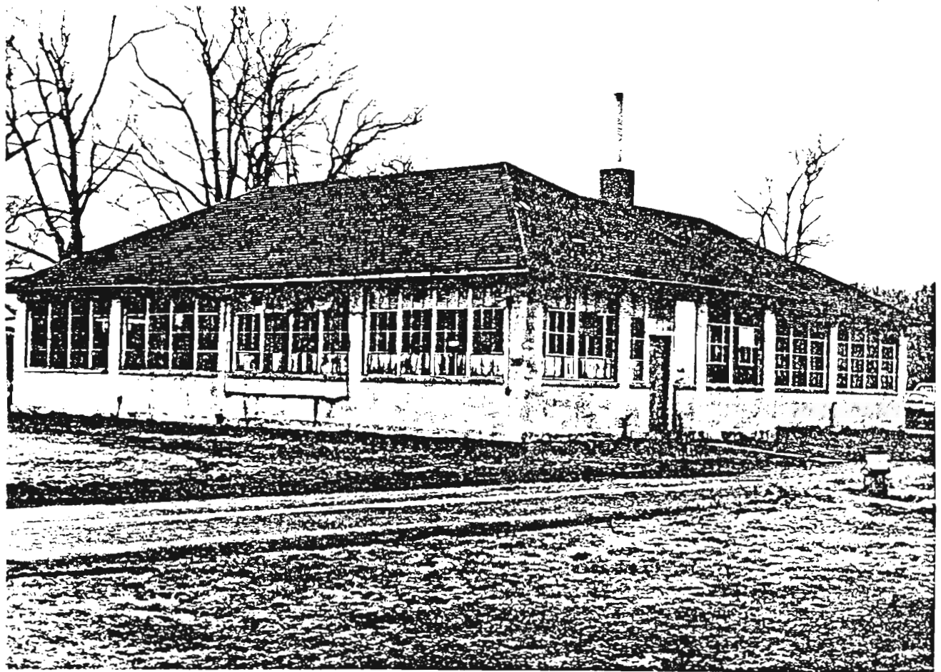
BUILDING C - (North facade)
