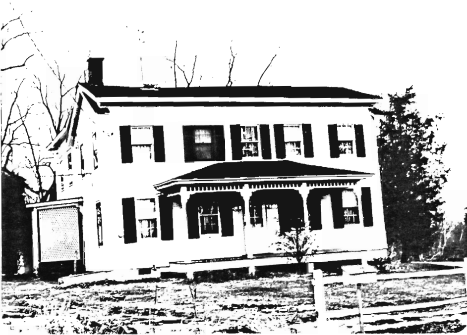
House A, view to NE.
