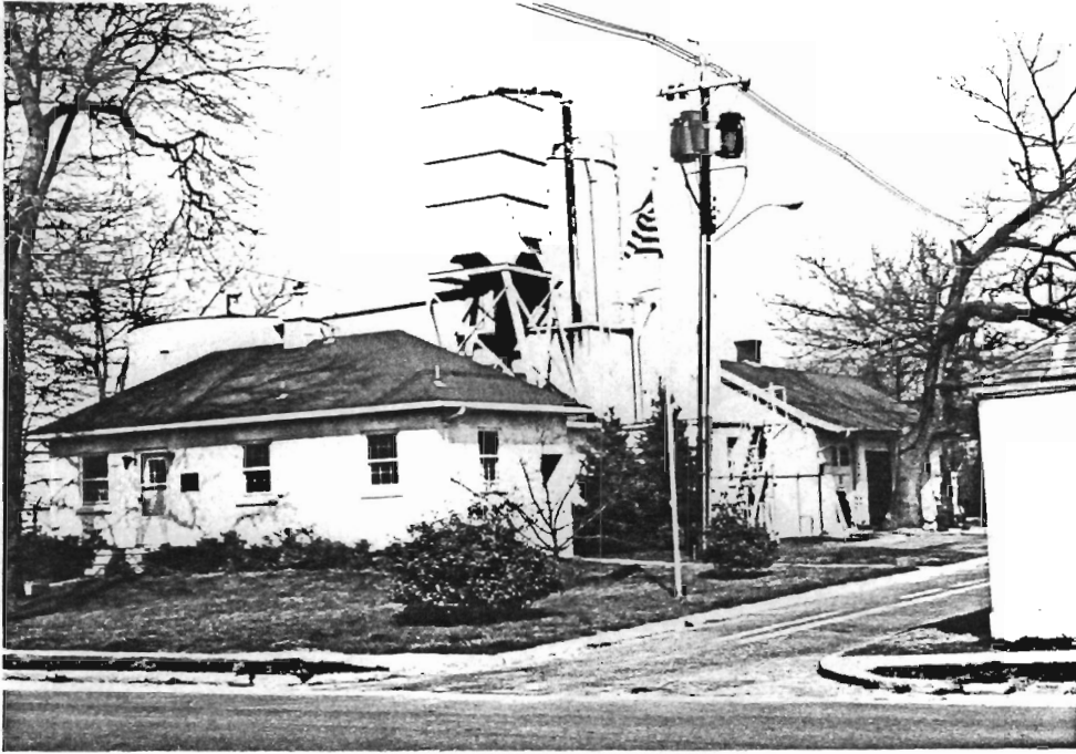
Utility and water processing buildings; view to NE.
