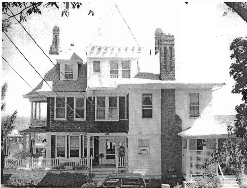
Rear of the house, facing north. 2006 photograph.
