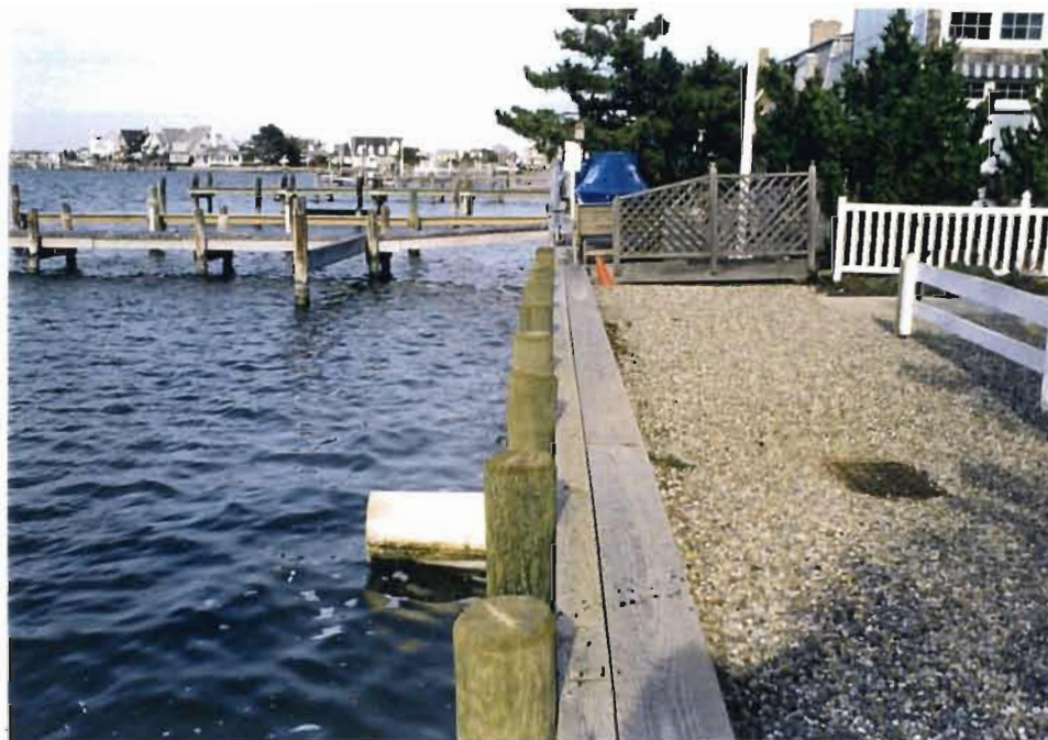
Photo 28: Lyman Street at Barnegat Bay facing north.
