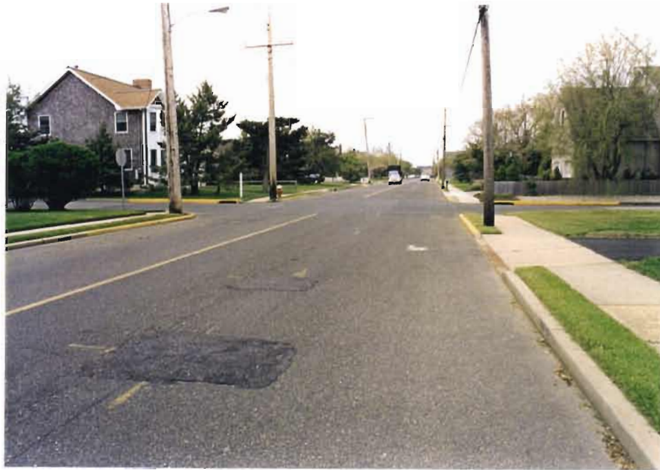
Photo 31: Lake Avenue at Forsyth Street facing south.
