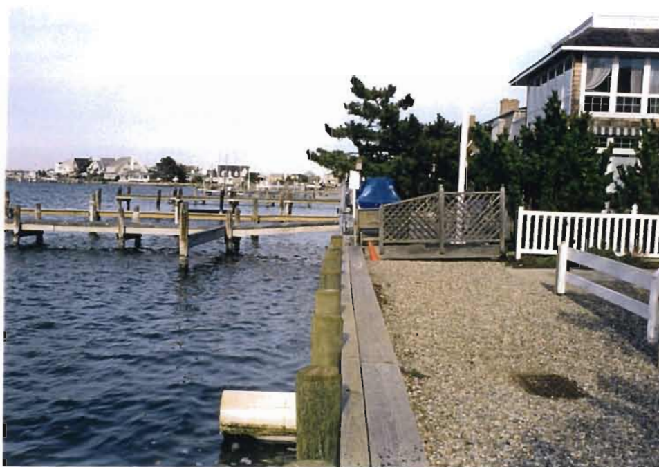
Photo 1: Lyman Street at Barnegat Bay facing north.
