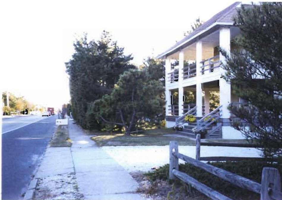
Photo 8: NJ Route 35 in vicinity of No. 1216 facing south in Mantoloking Borough. This photo shows a graveled and grass buffer between the sidewalk and curb; it also features a wood post and beam fence. This fencing is similar in materials and style to the fencing that lined NJ Route 35 historically and is a recommended option for use along the corridor.
