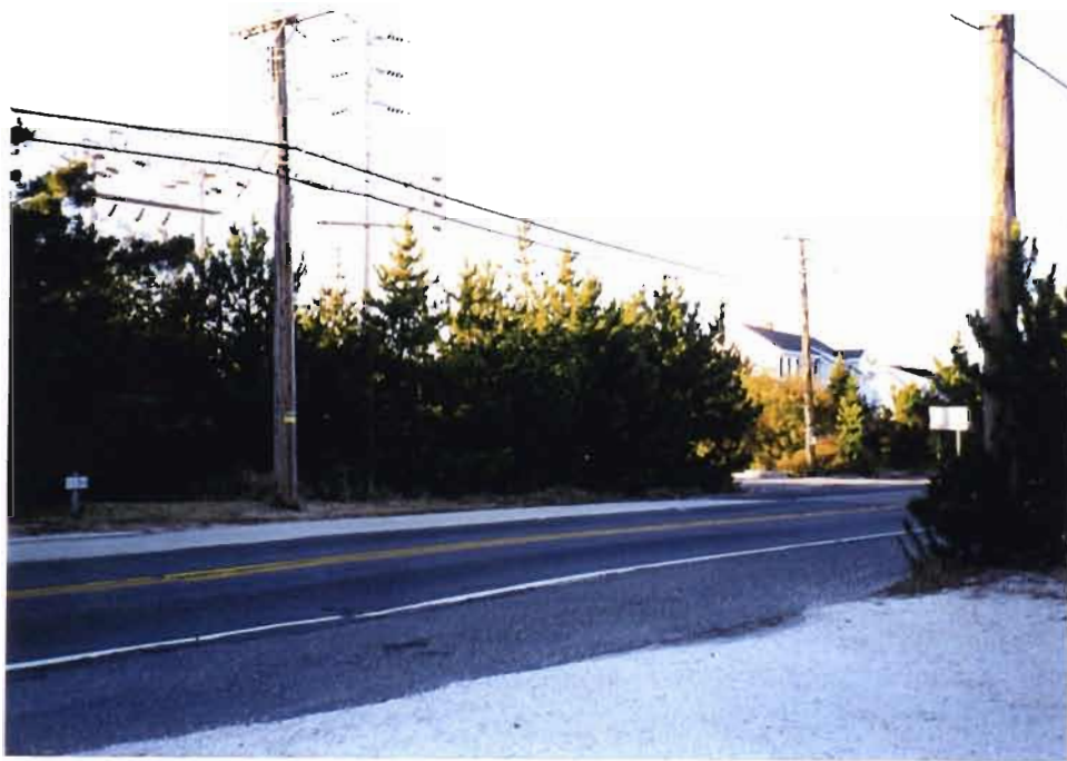
Photo 1: NJ Route 35 in vicinity of No. 1530 facing northwest.
