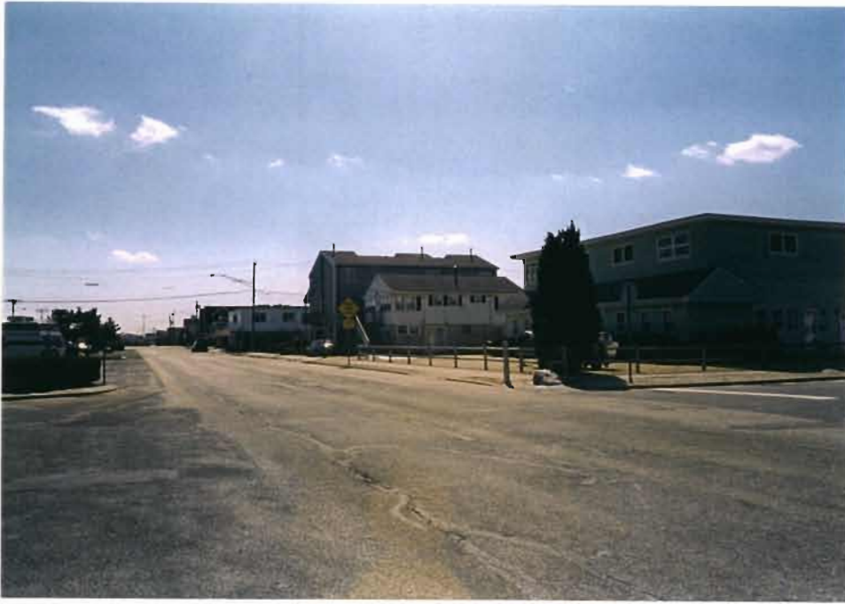
Photo 1: At intersection of NJ Route 35 and 11 th Avenue in Seaside Park facing southwest. This photo shows the conditions of the roadway and features an example of wood post and beam fencing. This fencing is similar in materials and style to the fencing that lined NJ Route 35 historically and is a recommended option for use along the corridor.
