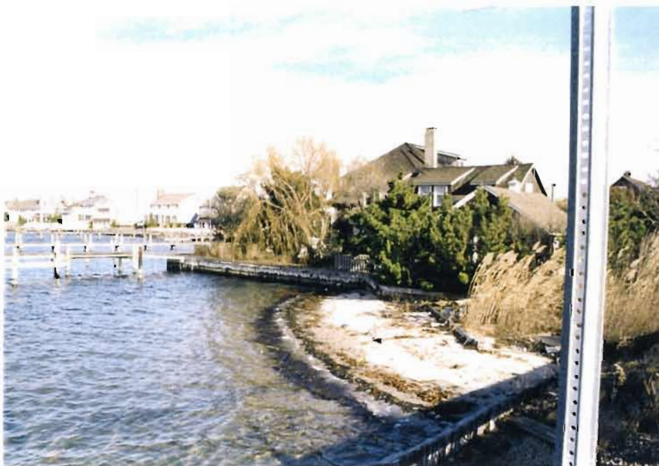
Photo 6: Herbert Street, east of Mantoloking Bridge, facing northeast.
