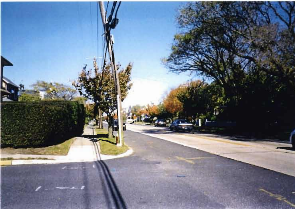
Photo 20: NJ Route 35 at Howe Street facing north.
