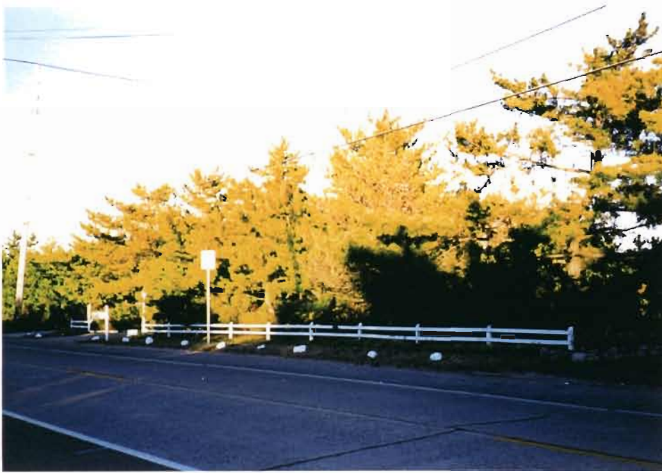
Photo 5: NJ Route 35 in vicinity of No. 1521 facing northeast in Mantoloking Borough. This photo features an example of wood post and beam fencing. This fencing is similar in materials and style to the fencing that lined NJ Route 35 historically and is a recommended option for use along the corridor.
