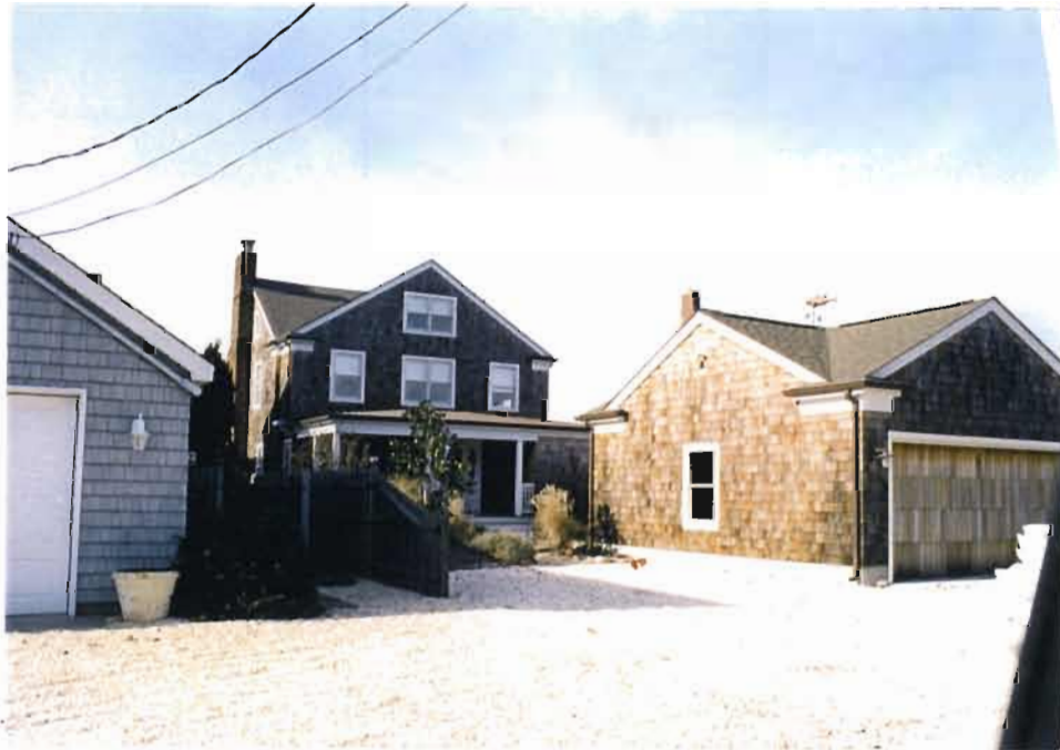
Photo 3: At 976 Barnegat Lane facing west.
