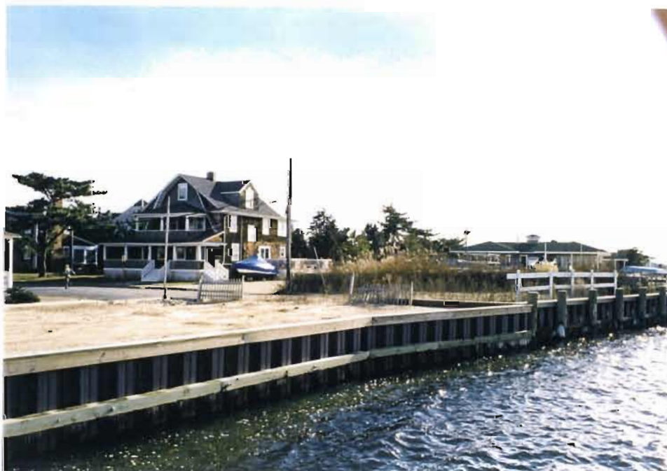
Photo 8: At Old Bridge Road and Barnegat Bay facing southeast.
