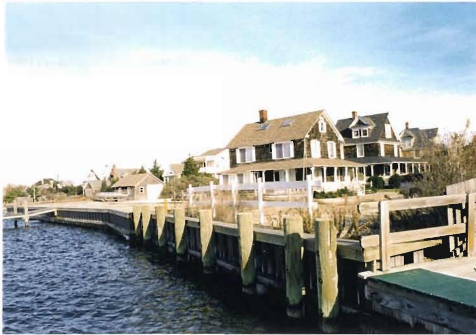
Photo 7: At Old Bridge Road and Barnegat Bay facing northeast.
