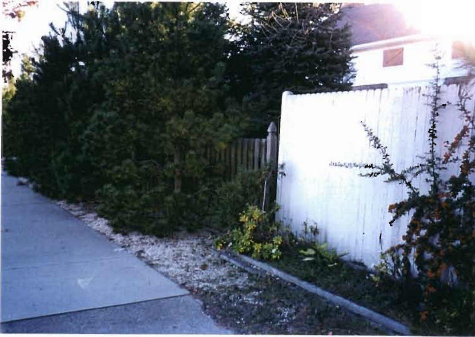
Photo 11: NJ Route 35 at Stephens Place facing south in Mantoloking Borough. This photo juxtaposes two types of fencing along the corridor. The natural wood fencing on the left may be an option for use along the corridor owing to its low height and more rustic quality, whereas the painted fencing on the right is not a similar style to the fencing that lined NJ Route 35 historically.
