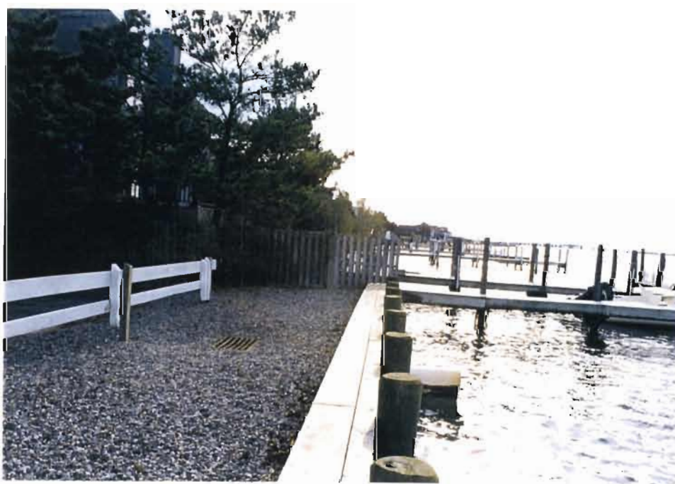
Photo 2: Lyman Street at Barnegat Bay facing south.
