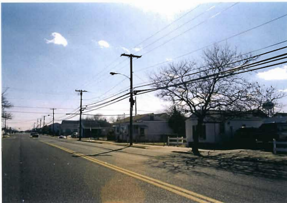
Photo 4: At intersection of NJ Route 35 and Fremont Avenue facing south in Dover Township. This photo shows the roadway conditions and cobrahead light attached to a utility pole; it also features an example of wood post and beam fencing. This fencing is similar in materials and style to the fencing that lined NJ Route 35 historically and is a recommended option for use along the corridor.
