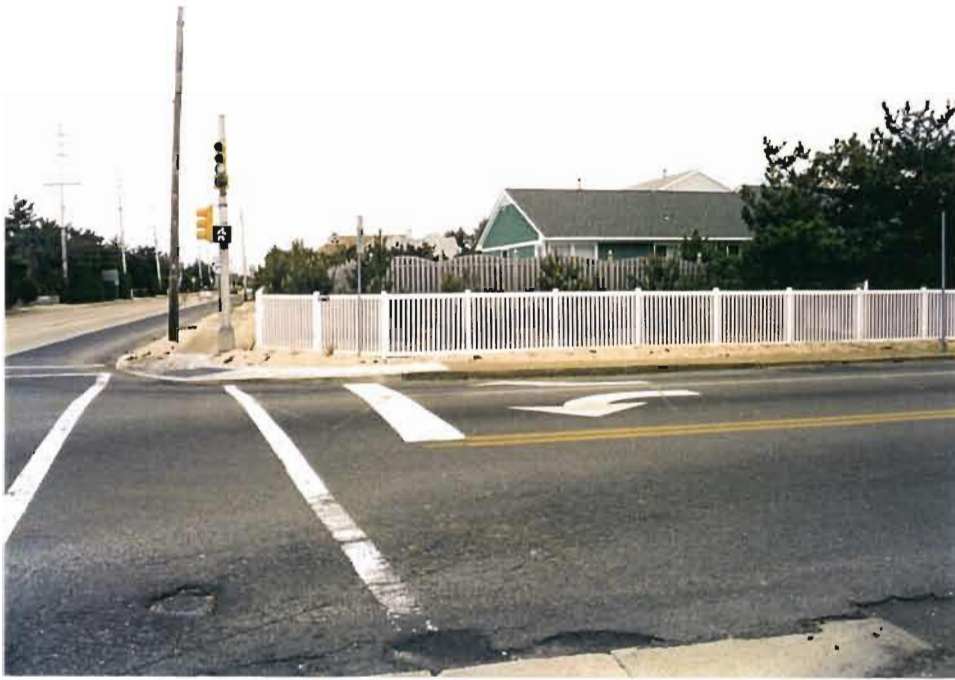
Photo 9: NJ Route 35 at Herbert Street facing west in Mantoloking Borough. This photo shows another variety of plastic picket fencing along the corridor. This fencing is not similar in materials or style to the fencing that lined NJ Route 35 historically and is not a recommended option for use along the corridor.
