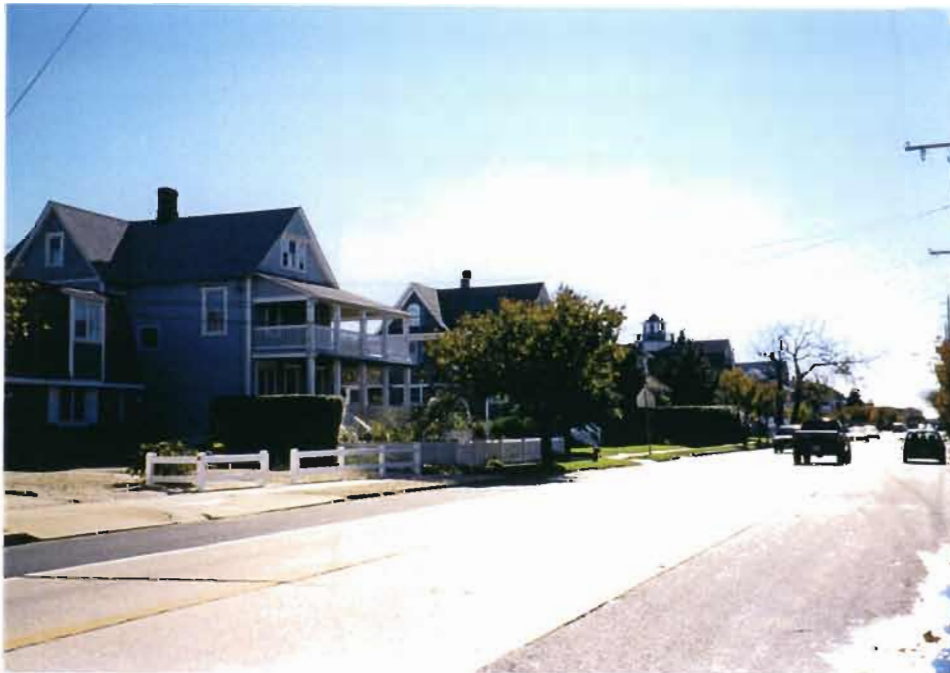
Photo 14: NJ Route 35 south of Mount Street facing southeast in Bay Head Borough. This photo shows the asphalt shoulders with the concrete vehicle lanes as well as wood post and beam fencing. This fencing is similar in materials and style to the fencing that lined NJ Route 35 historically and is a recommended option for use along the corridor.
