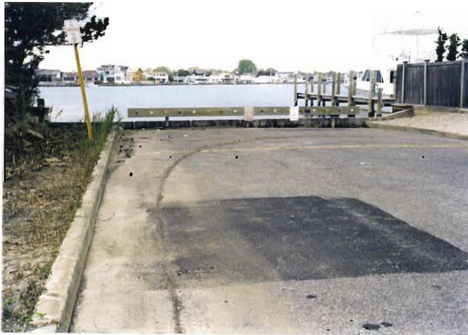
Photo 30: At Johnson Street facing west to Barnegat Bay.
