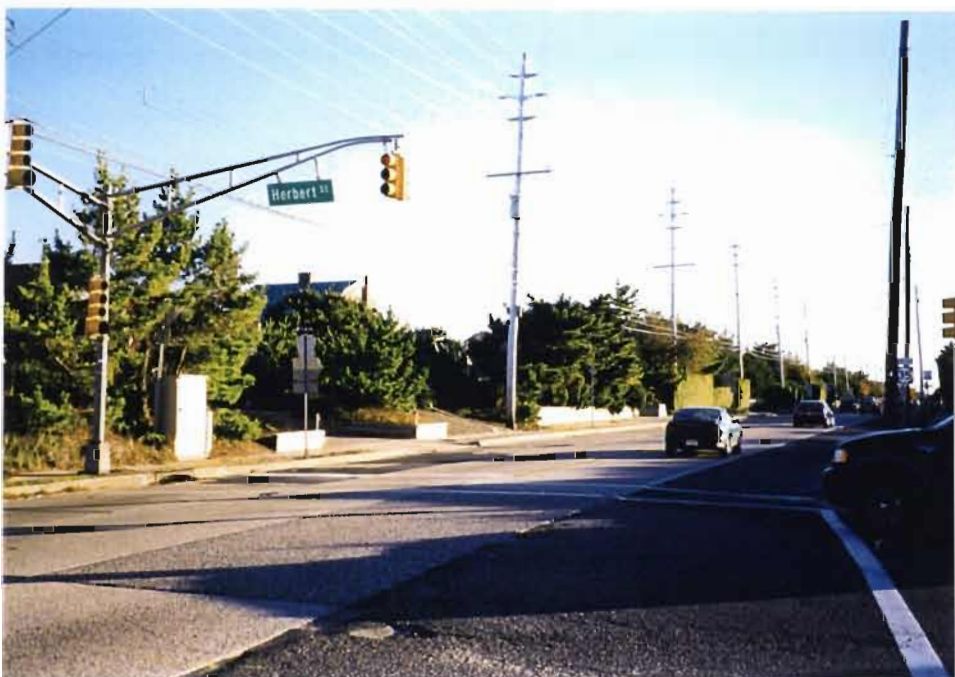
Photo 10: NJ Route 35 at Herbert Street facing southeast.
