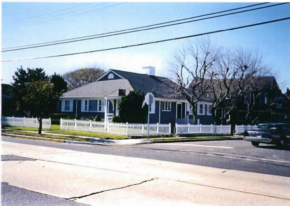
Photo 16: NJ Route 35 at intersection of Harris Street facing west in Bay Head Borough. This photo shows the roadway condition as well as another example of a wood picket fence along the corridor. This fencing is not similar in style to the fencing that lined NJ Route 35 historically and is not a recommended option for use along the corridor.
