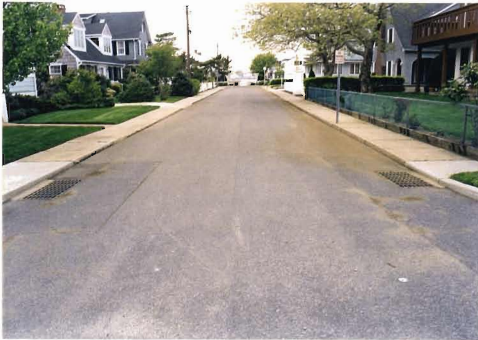
Photo 29: Egbert Street at Clayton Avenue facing west to Barnegat Bay.
