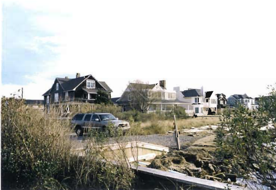
Photo 6: Bay Avenue at Barnegat Bay facing southeast.
