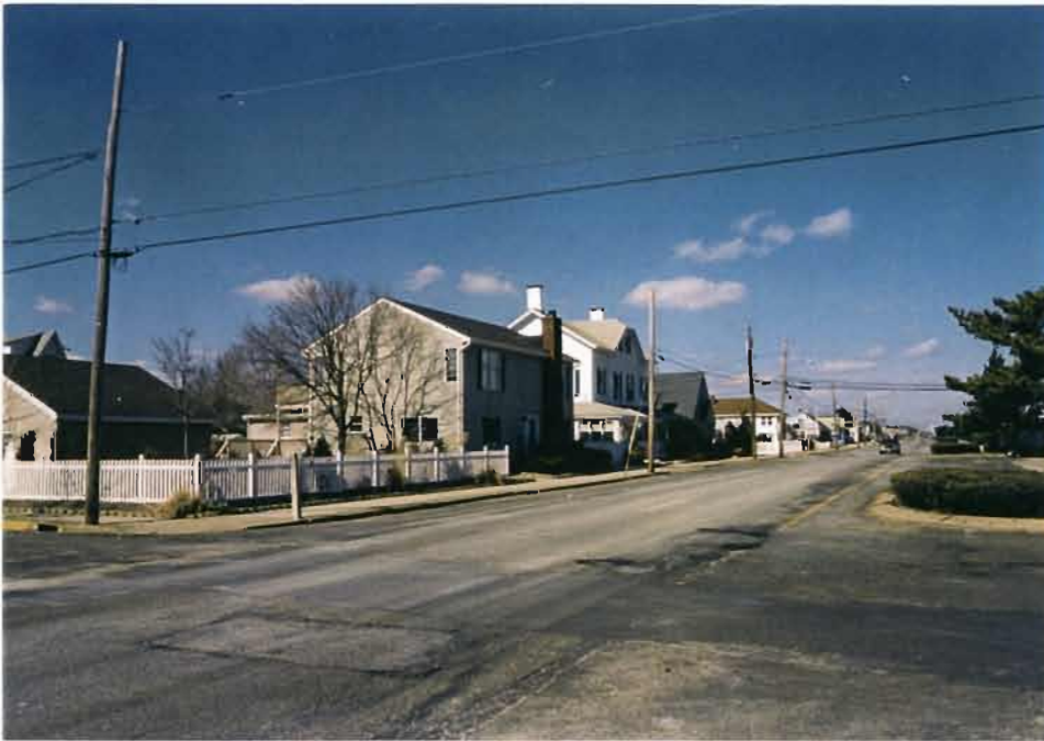
Photo 2: At intersection of NJ Route 35 and North Avenue facing northwest in Seaside Park. This photo shows the conditions of the roadway and features an example of plastic picket fencing. This fencing is not similar in materials or style to the fencing that lined NJ Route 35 historically and is not a recommended option for use along the corridor.
