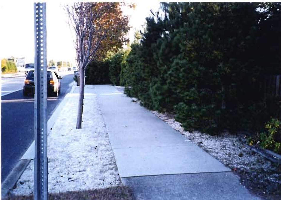
Photo12: NJ Route 35 at Stephens Place facing south.
