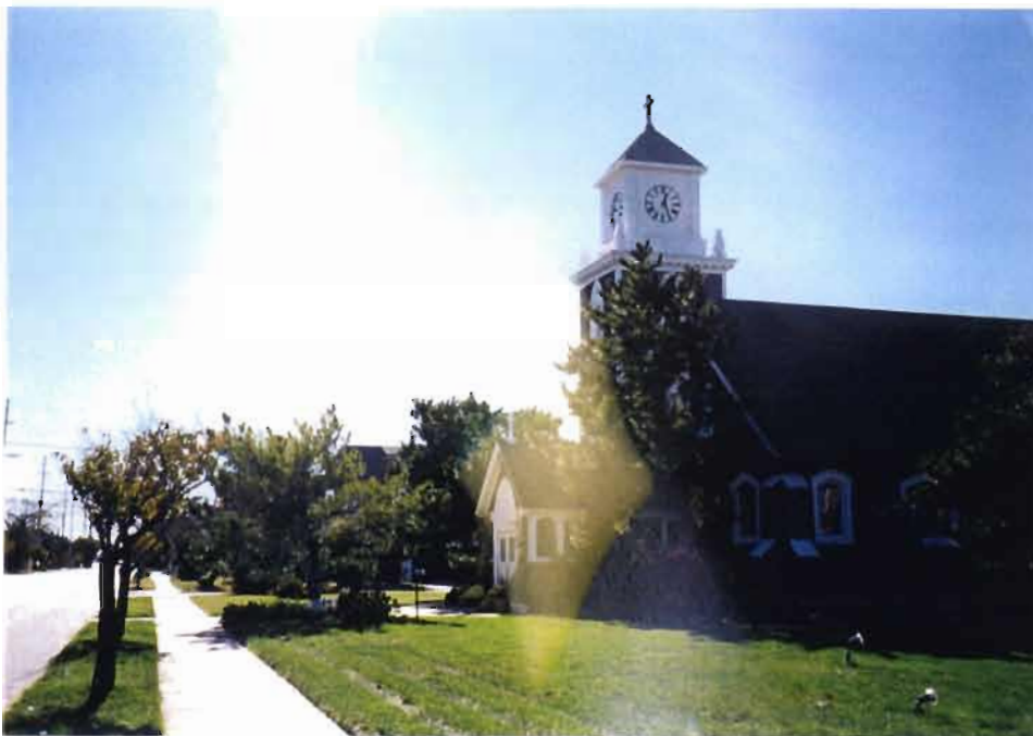
Photo 16: NJ Route 35 at Goetz Street facing south.
